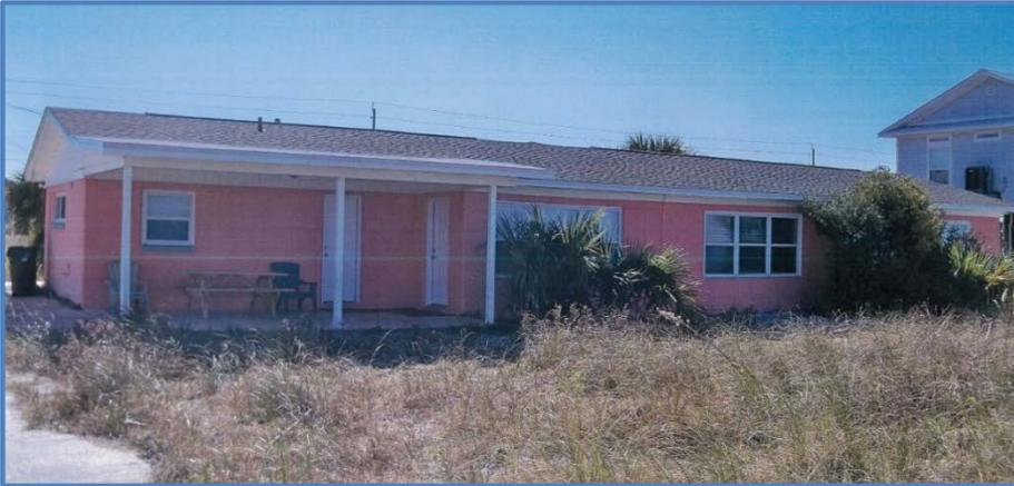
*This is a typical older home on Santa Rosa Island—built on a concrete slab at ground level.*
