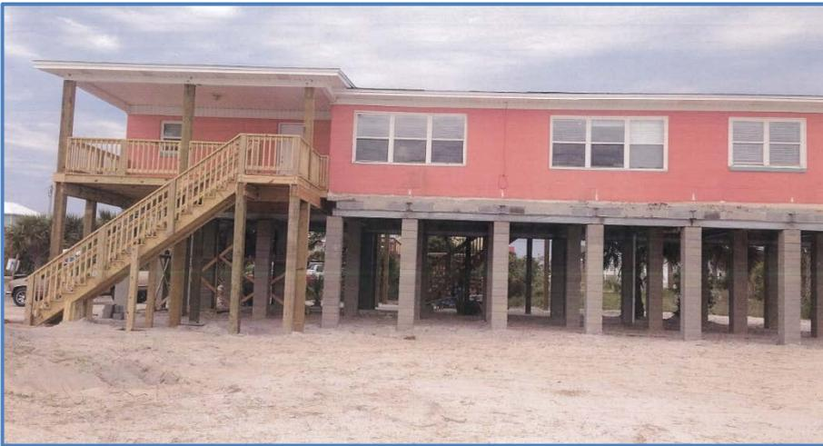
*Below, the same home after being raised above the expected flood level on pilings that allow waves and storm surge to flow beneath the structure.*
