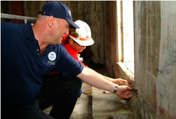
FEMA Mitigation Specialist Marshall Marik inspects for structural damage to the Hilo, Hawaii Fire Station with U.S. Army Corps structural engineer Peter Lam after a recent series of earthquakes. November 13, 2006. FEMA Image.
