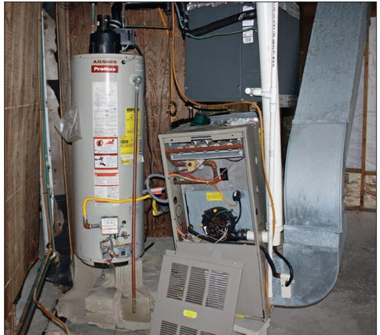
Figure 1: A water heater and furnace system damaged by Hurricane Sandy floodwaters (Beach Haven, NJ)
