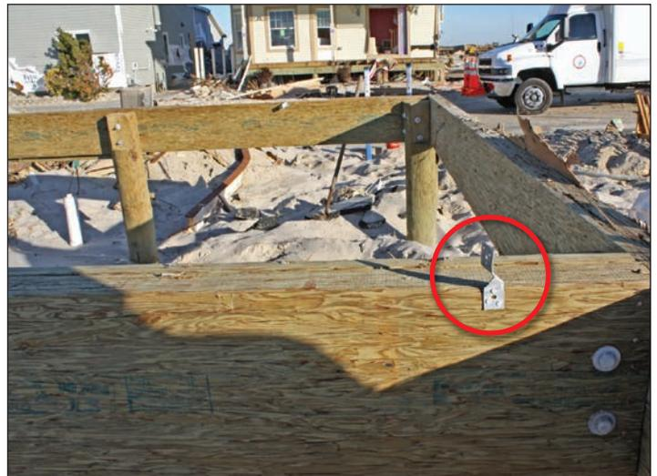
**Figure 1: Building with insufficient connectors (red circle) washed off its pile foundation when elevated floor-to-pile connectors failed. Stronger connectors were used on the house in the background (Ortley Beach, NJ).**
