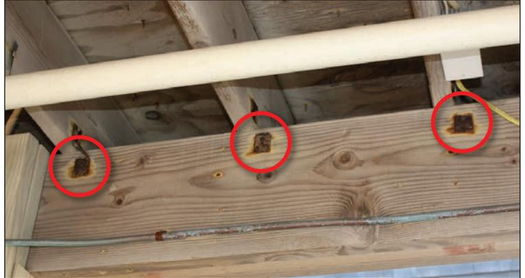
**Figure 5. Corroded connectors (red circles) and lack of blocking mean there is no longer a continuous load path providing uplift and shear transfer to foundation piles (Fire Island, NY)**
