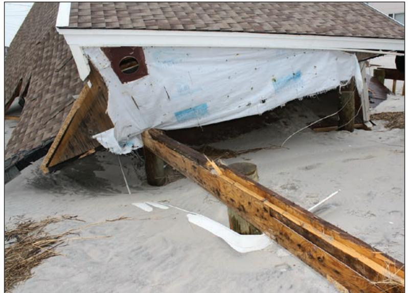
**Figure 3: Building with connectors nailed along the grain in the upper edge of the wood beam resulted in the beam splitting (Beach Haven, NJ)**
