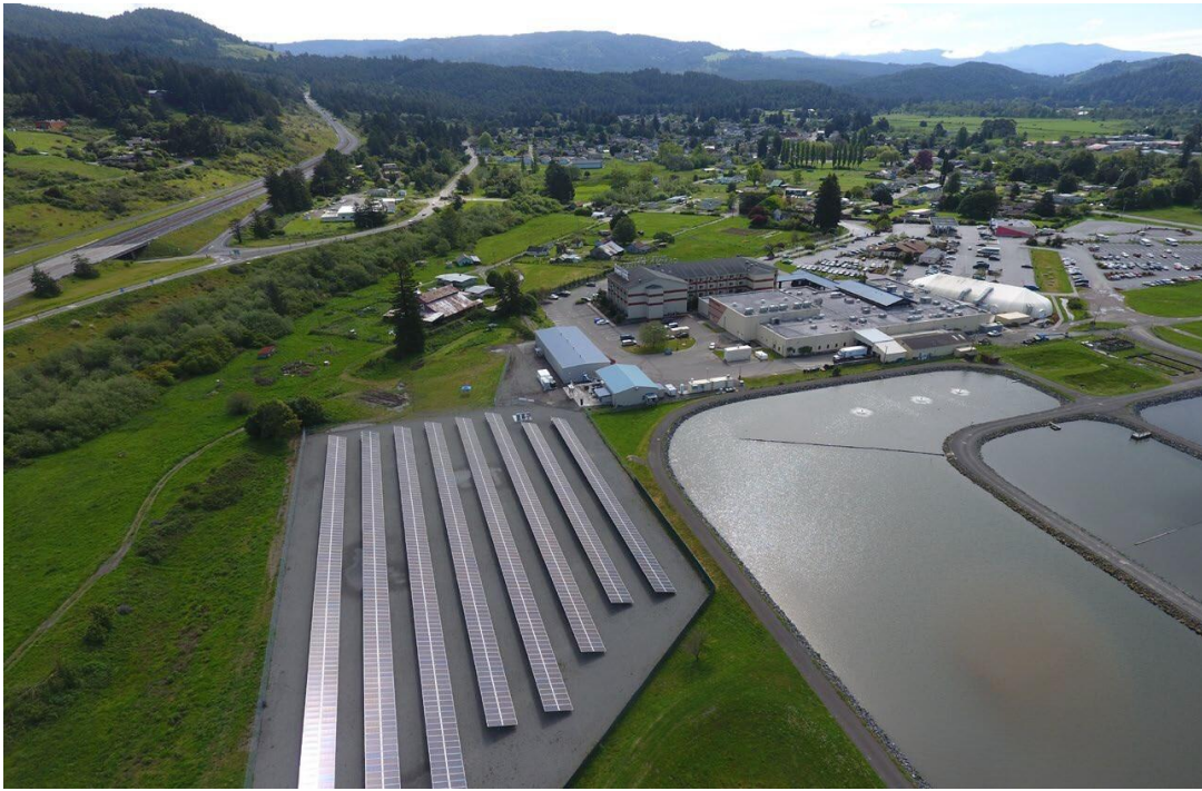
Blue Lake Rancheria Tribe Microgrid Project in Humboldt Bay, CA
