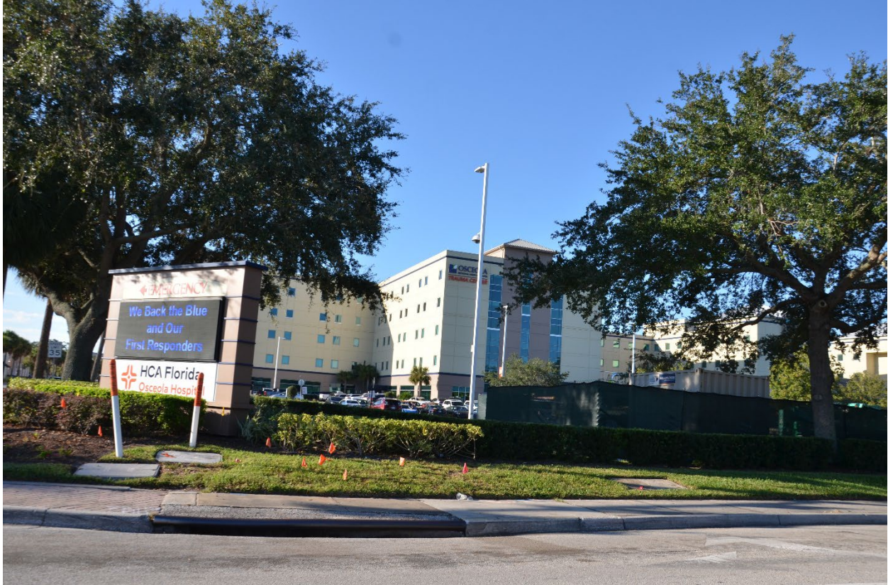
Figure 5-15: Access roads at Osceola Regional Medical Center Trauma Center that flooded, isolating the hospital for 2 hours (Osceola County, Zone AE)
