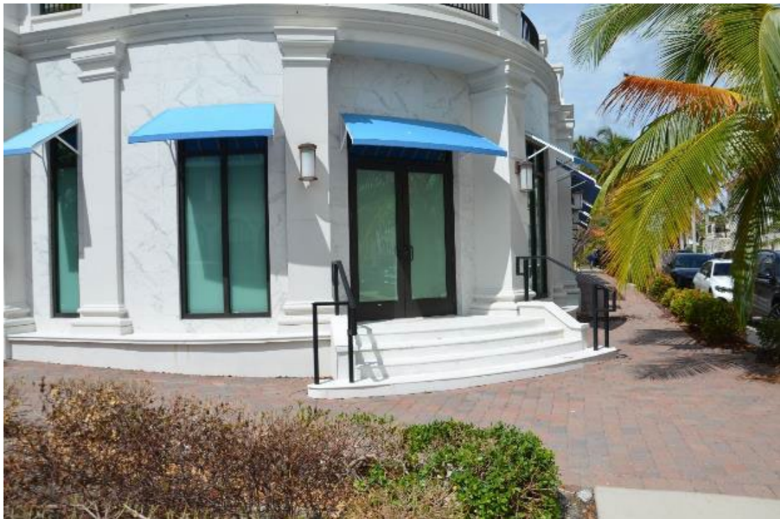
Figure 3-66: Building elevated on fill and foundation walls in downtown Naples (Collier County, Zone AE)
