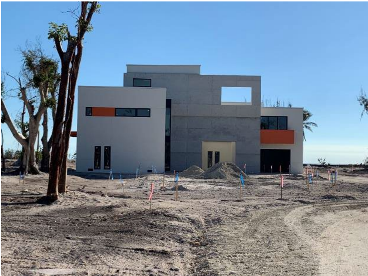
Figure 3-10: Large CMU structure on Sanibel Island (Lee County, Zone VE, Seaward of CCCL)
