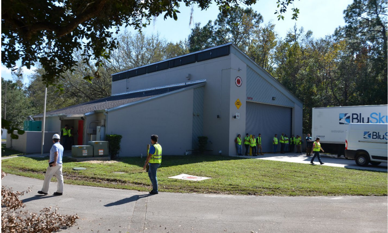
Figure 5-49: Volusia County Fire Station #12 (Volusia County)
