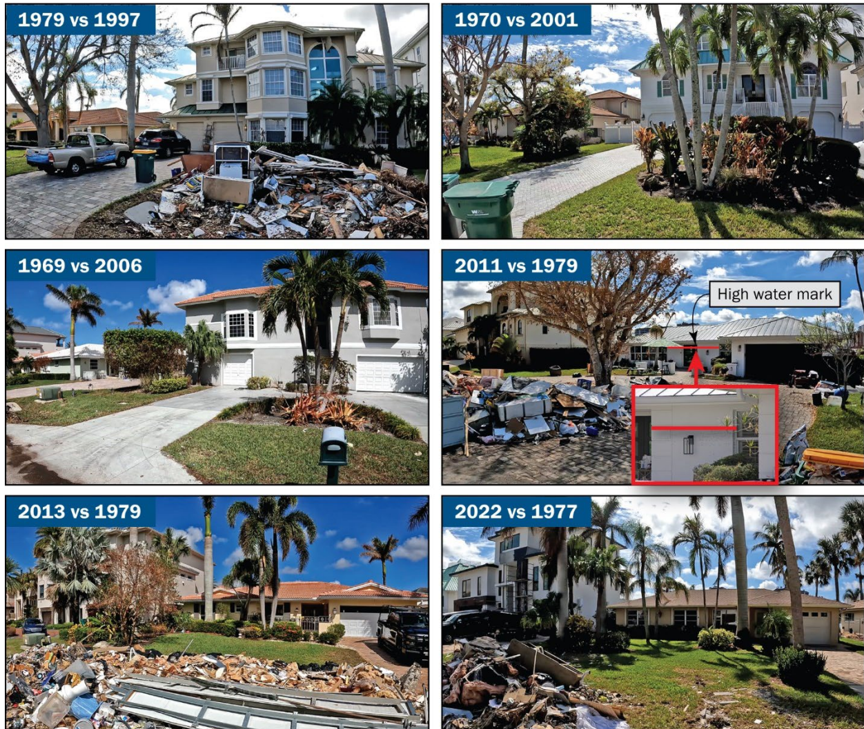
Figure 25: Representative single-family houses in Area of Interest No. 11 from 1969 to 2022
