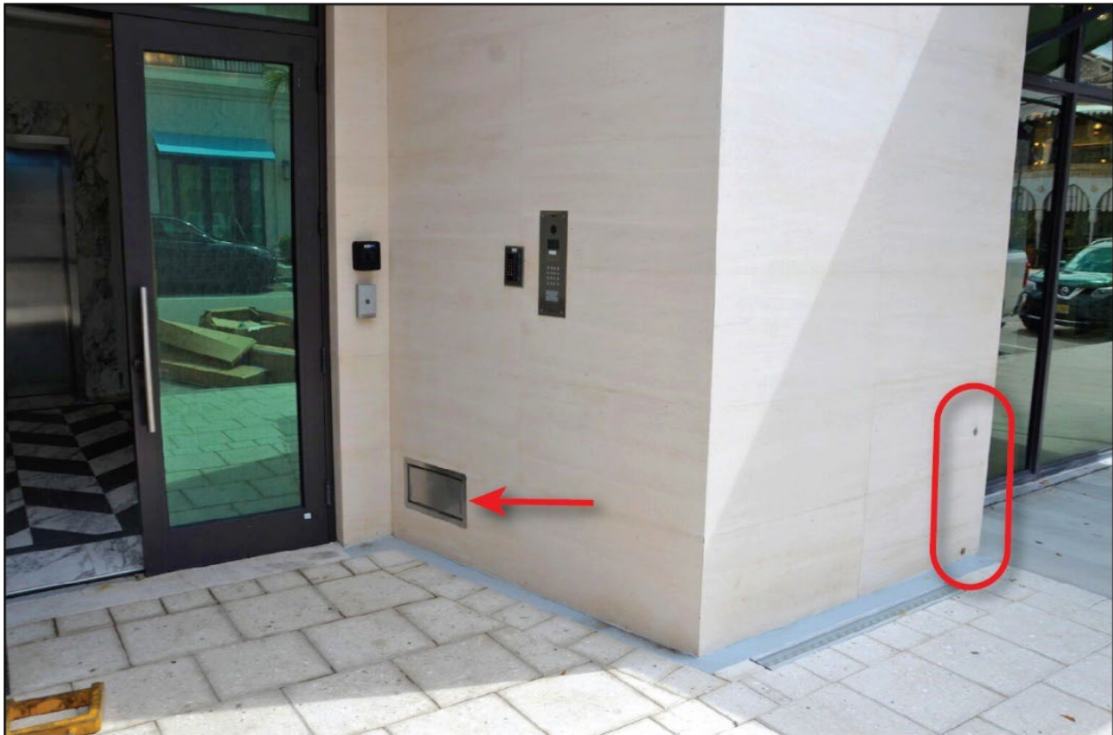
Figure 3-73: Mixed-use building with wet floodproofing measures (arrow) in residential access area and dry floodproofing measures (circle) in retail space/non-residential area (Collier County, Zone AE)
