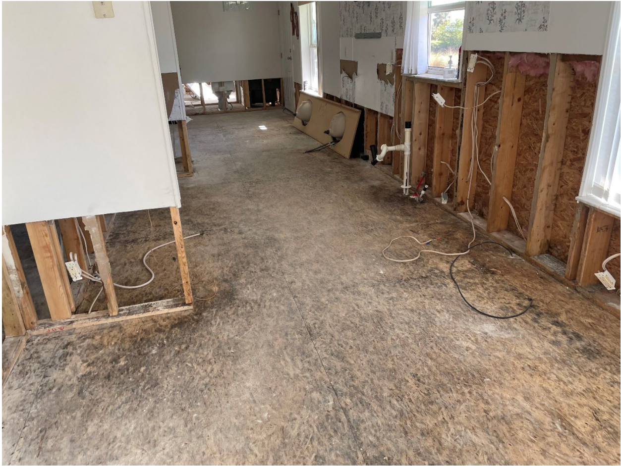
Figure 3-115: Common manufactured home interior finishing damage observed in Old Bridge Village (Lee County, Zone AE)
