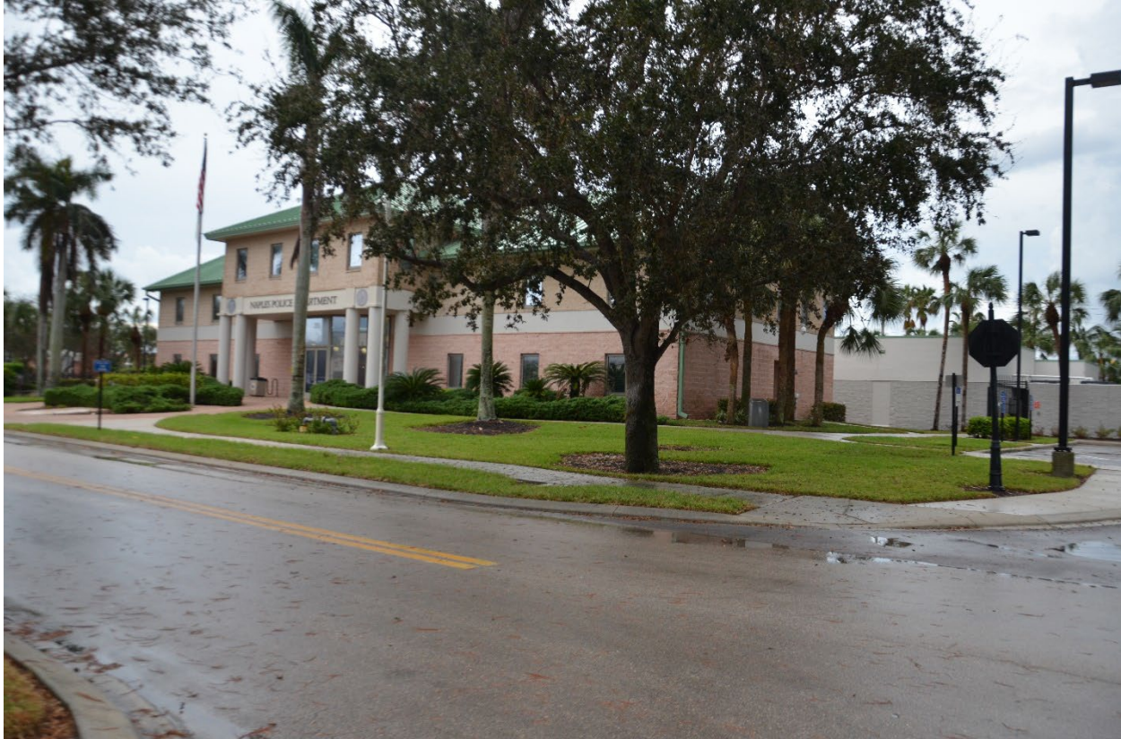
Figure 5-74: Naples Police Department with the 1999 addition in the foreground and the older 1978 structure in the background to the right (Collier County, Zone AE)
