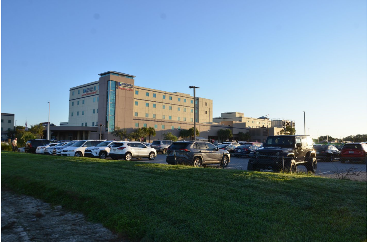
Figure 5-14: Osceola Regional Medical Center Trauma Center parking lots that were flooded (Osceola County, Zone AE)
