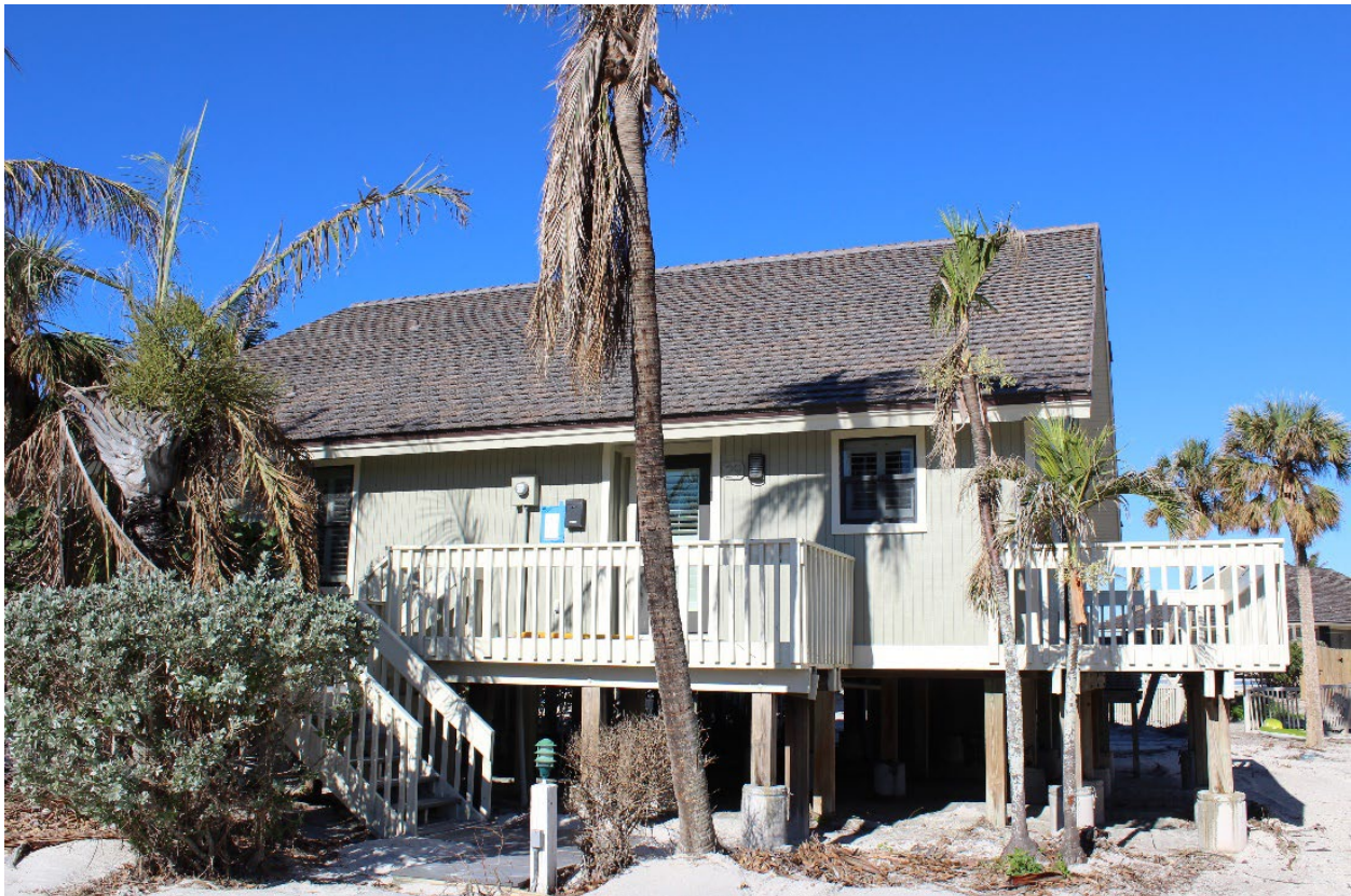
Figure 4-20: A house built in 1974 with a tile replacement in July 2020 with no visible damage (EWS = 123 mph, DWS = 162 mph) (Captiva)
