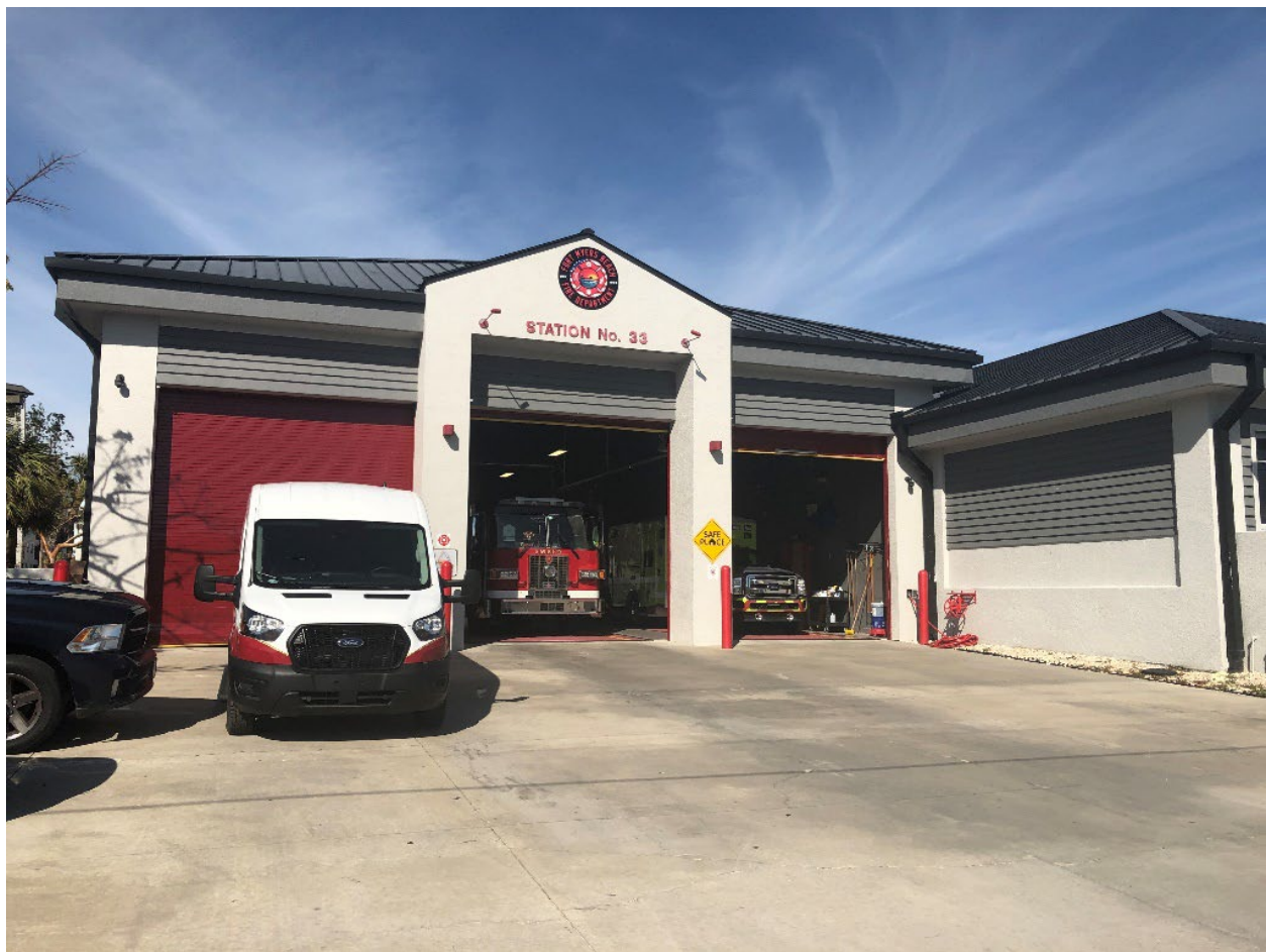
Figure 5-55: Fort Myers Beach Fire Station #33 (Lee County)
