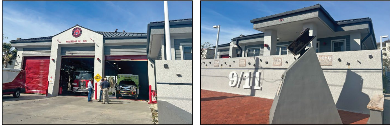
Figure 5-29: Fort Myers Beach Fire Station #33 apparatus bay (left) and commercial and residential area (right) (Lee County, Zone AE)
