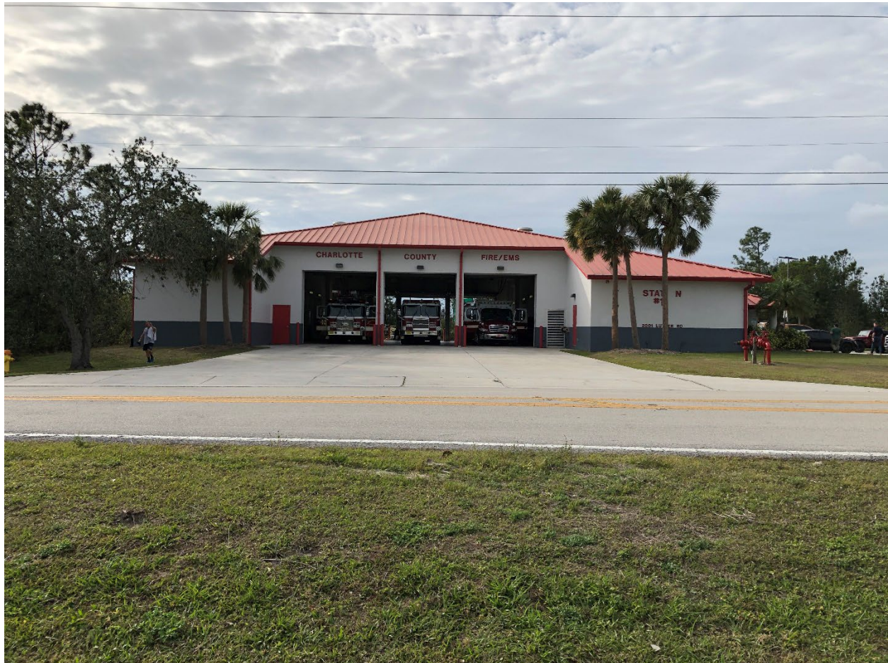
Figure 5-71: Charlotte County Fire Station #12 (Charlotte County)
