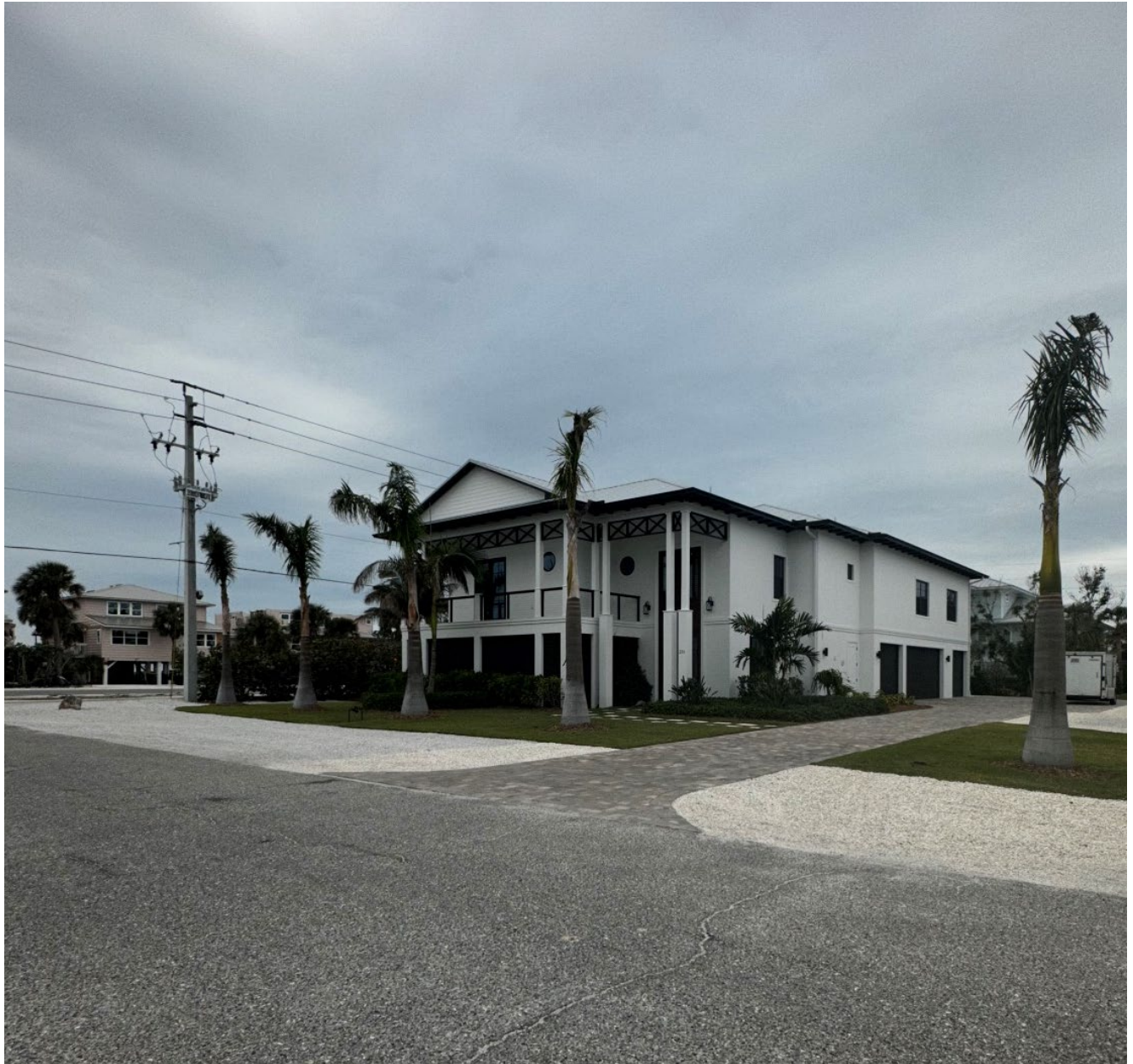
Figure 4-49: A house built in 2022 that had no visible signs of damage (EWS = 130 mph; DWS = 150 mph) (Boca Grande)
