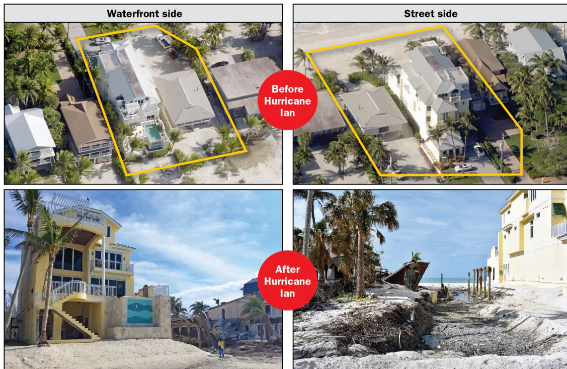
Figure 3-26: Photos before and after Hurricane Ian depicting significant scour on Bonita Beach (Lee County, Zone VE, Seaward of CCCL)
