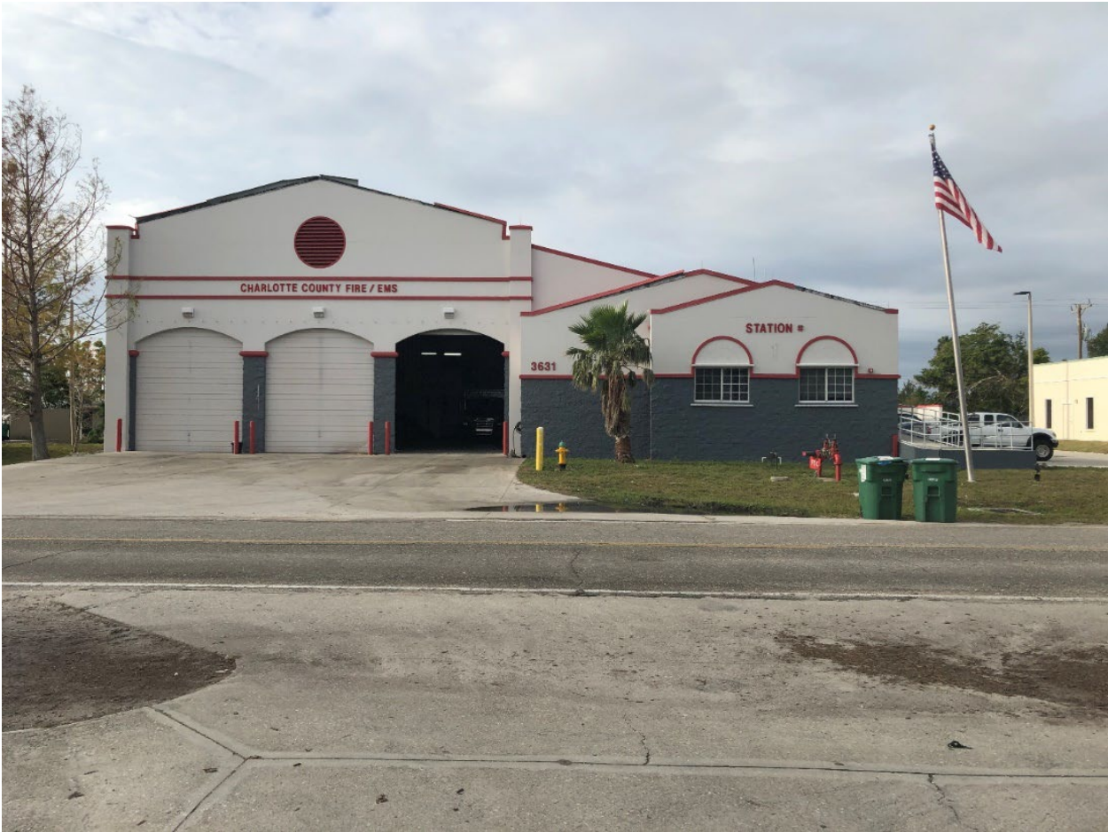
Figure 5-66: Charlotte County Fire Station #1 (Charlotte County)
