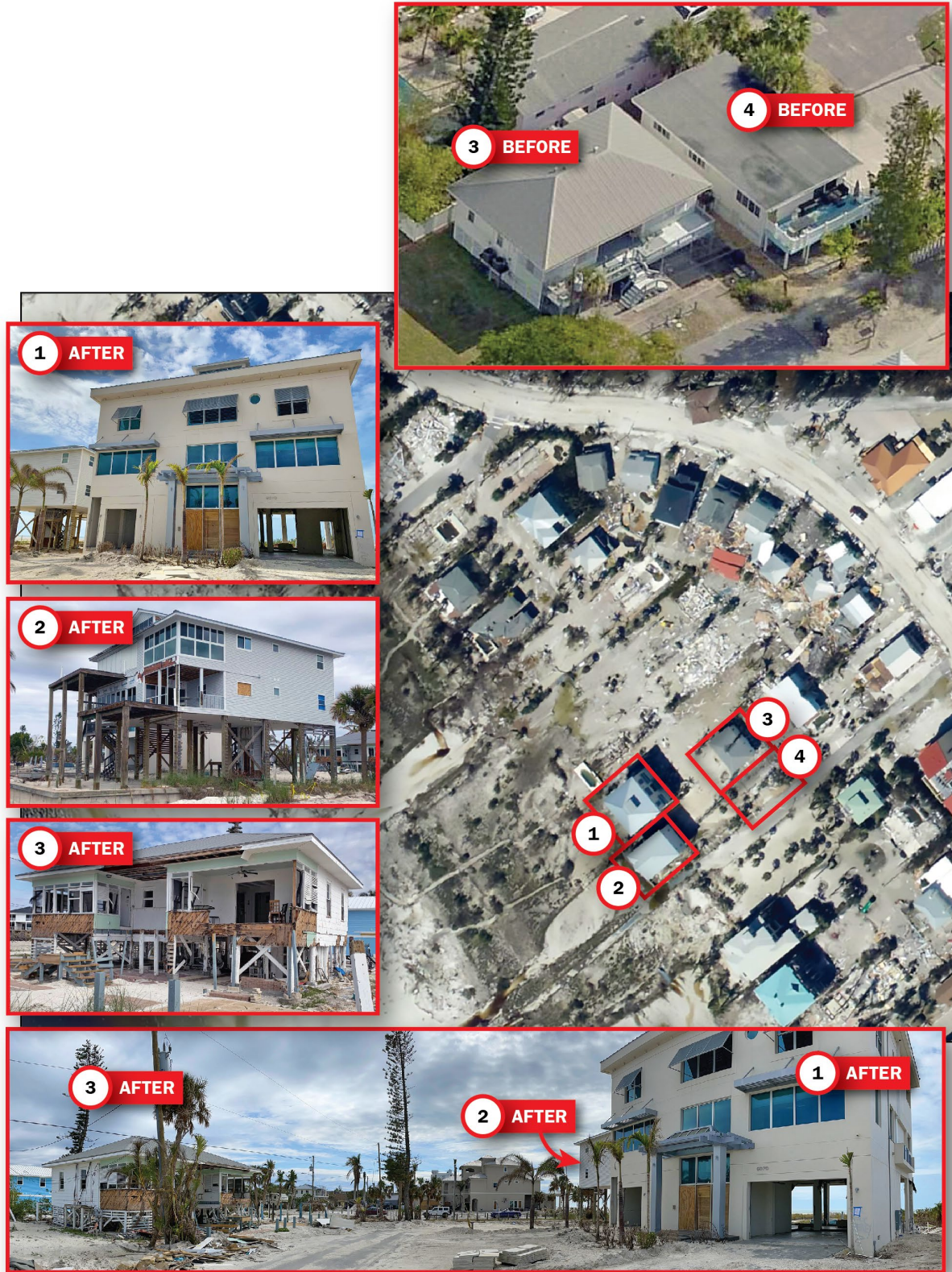
Figure 3-9: New concrete construction on coast (#1) could have provided shelter against waves to older, vulnerable structure (#3) on Fort Myers Beach (Lee County, Zone VE)
