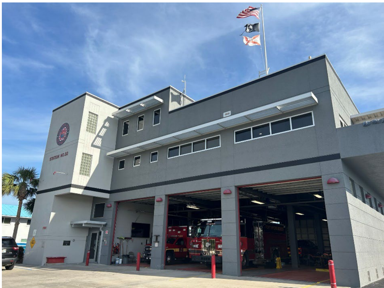
Figure 5-59: Fort Myers Beach Fire Station #32 (Lee County)
