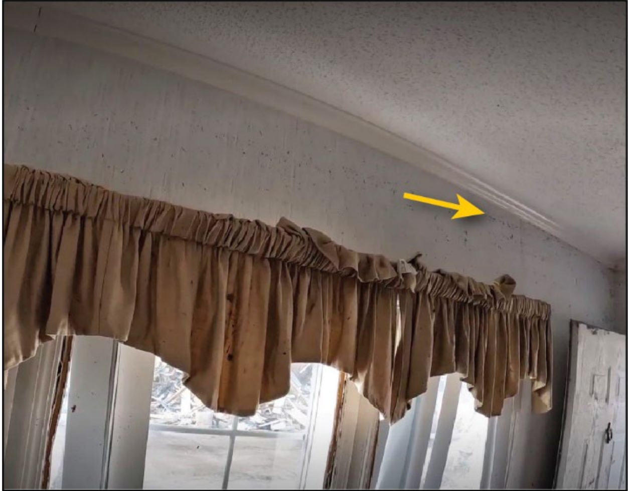
Figure 3-125: HWM near ceiling in Port Carlos Cove manufactured home (Lee County, Zone VE)
