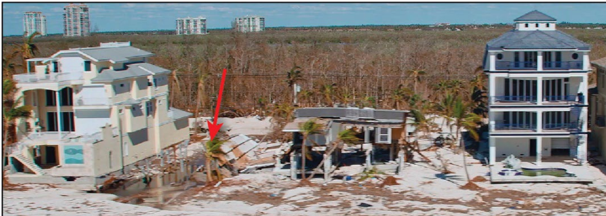
Figure 3-25: Scour beside and under houses in Bonita Beach (Lee County, Zone VE, Seaward of CCCL)
