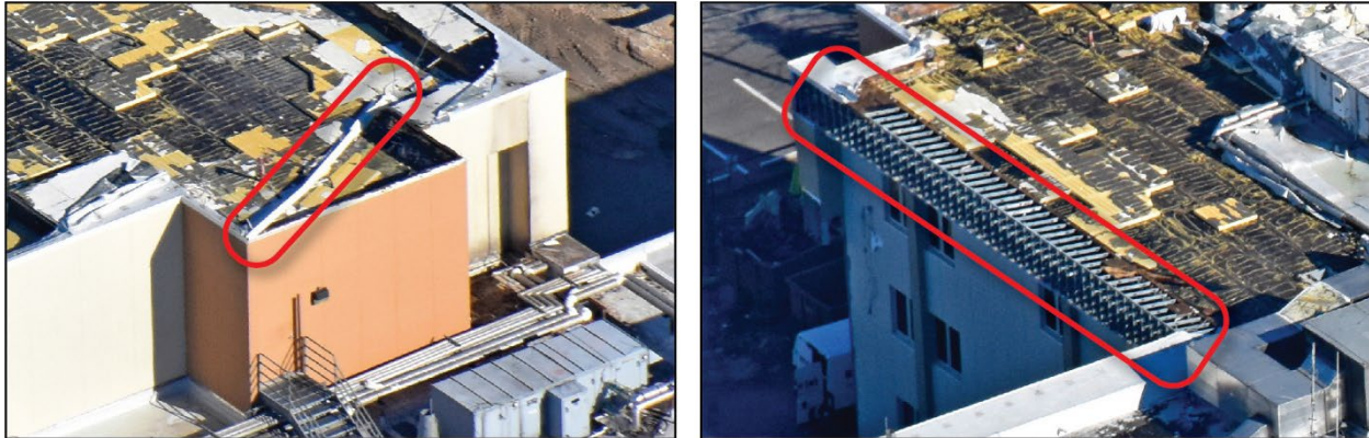
Figure 5-10: Detached nailing strip over a stairwell (left) and damaged mansard envelope system (right) (Southwest Florida)
