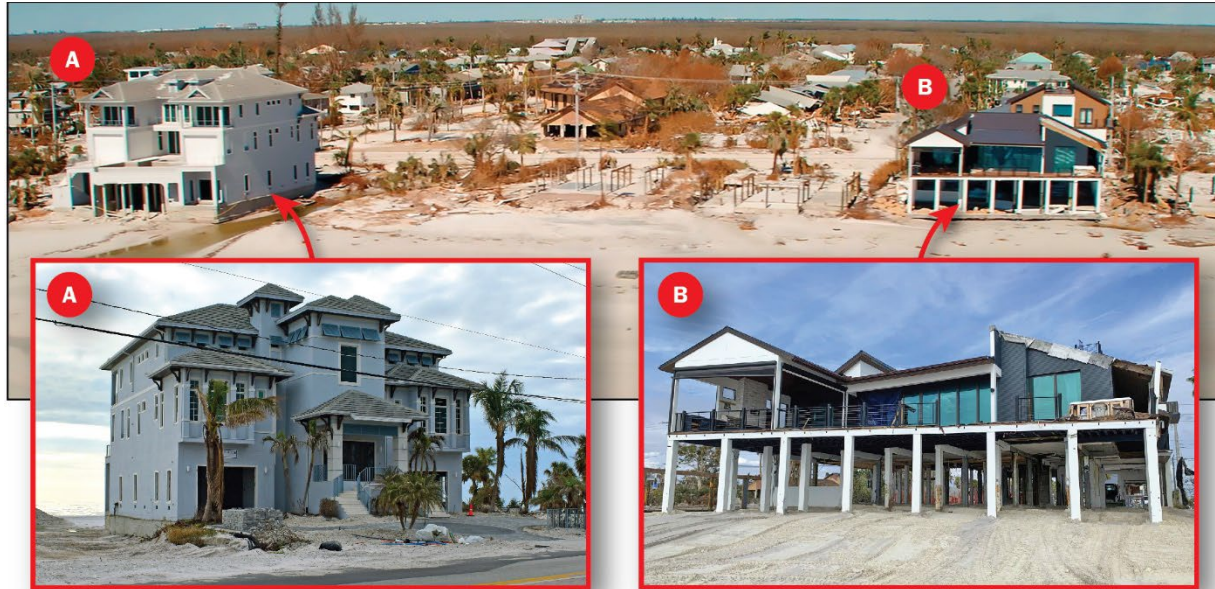
Figure 3-13: Comparison of nearby breakaway walls in Fort Myers Beach (Lee County, Zone VE, Seaward of the CCCL)
