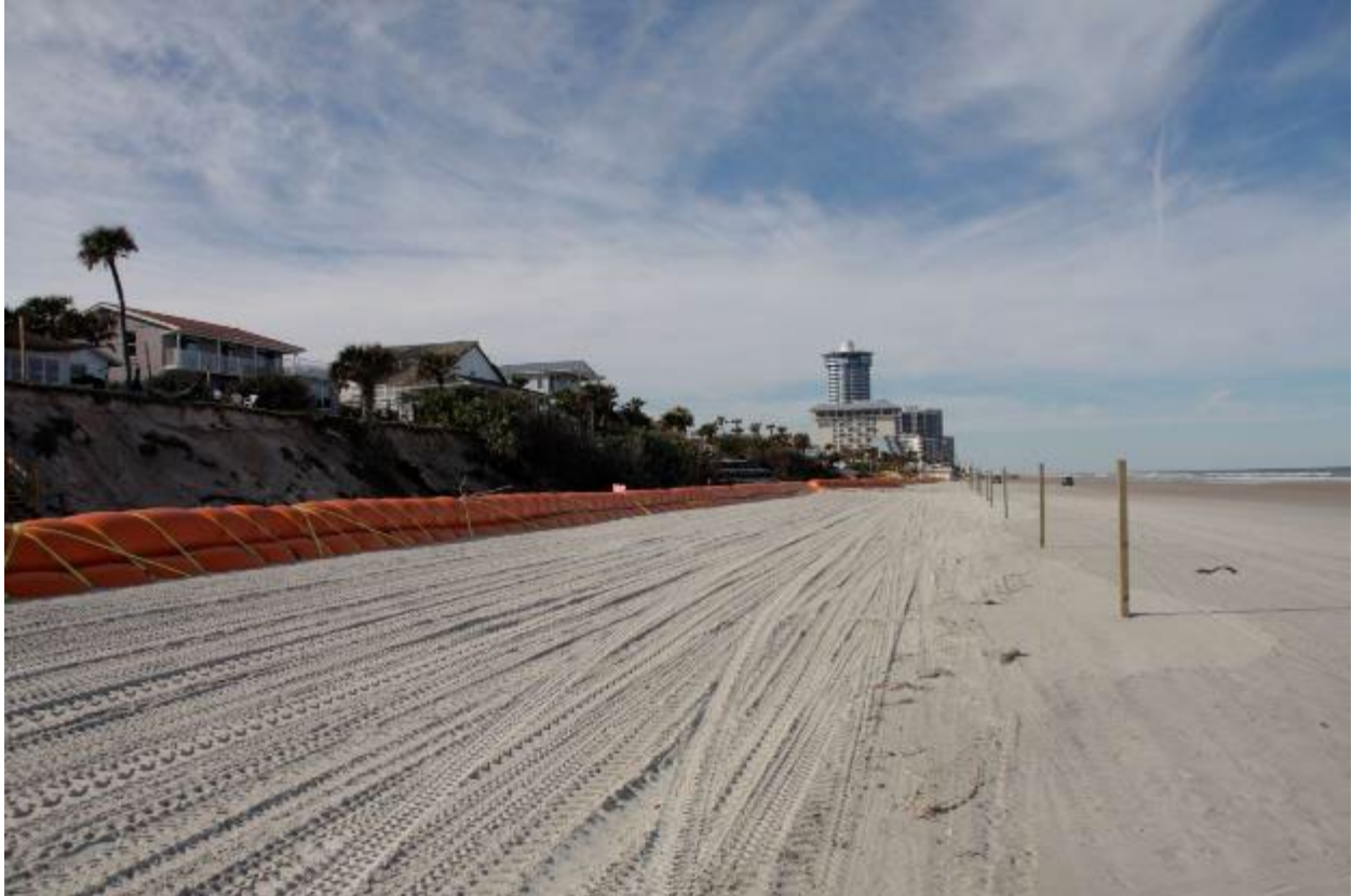
Figure 3-39: Temporary erosion control installed along Daytona Beach Shores to help counteract further coastal erosion in an area where seawalls were destroyed (Volusia County)
