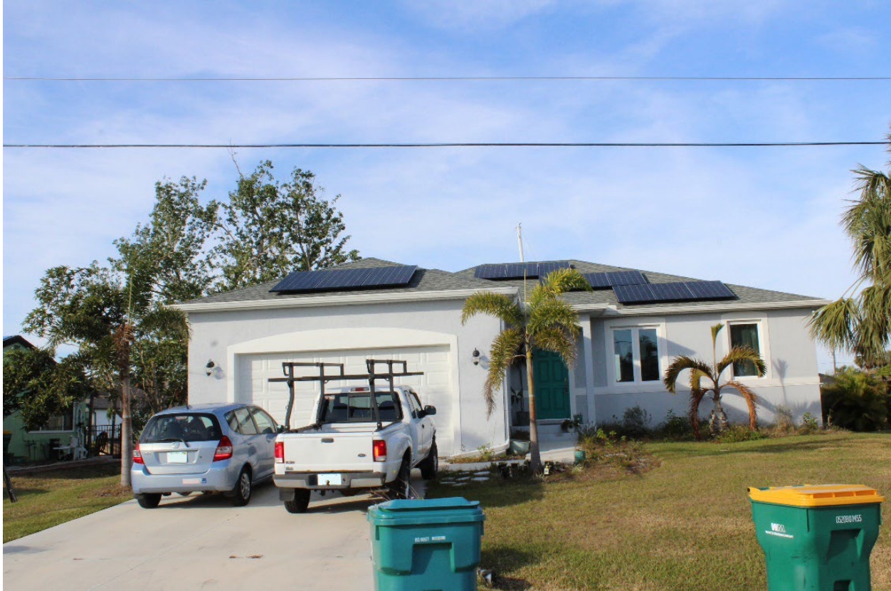
Figure 4-32: A house built post-2020 with asphalt shingle roof and photovoltaic panels; no damage observed (located in the Port Charlotte neighborhood in Figure 4-31) (EWS = 127 mph)
