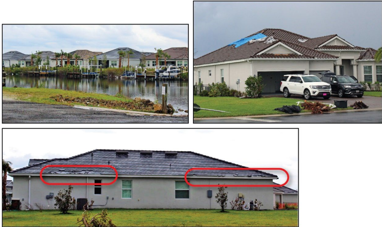
Figure 4-24: Neighborhood built in 2020 and 2021 with tile roof coverings with minor and moderate damage (EWS = 126 mph; DWS = 153 mph) (Port Charlotte)
