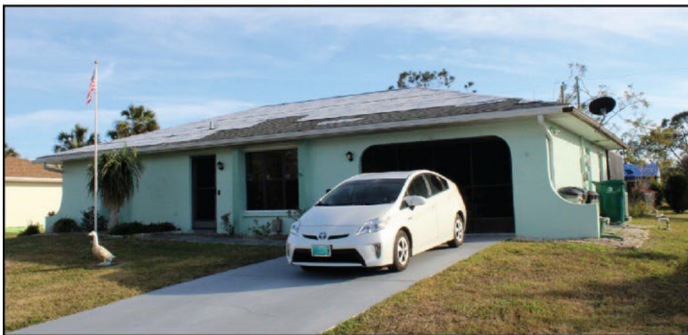
Figure 4-33: Houses with asphalt shingle roofs; top built in 1984 and reroofed in 2022 (no damage observed); middle built in 1984 (damage observed on NOAA imagery); bottom built in 1990 (damage observed on NOAA imagery) (located in the Port Charlotte neighborhood in Figure 4-31) (EWS = 127 mph)
