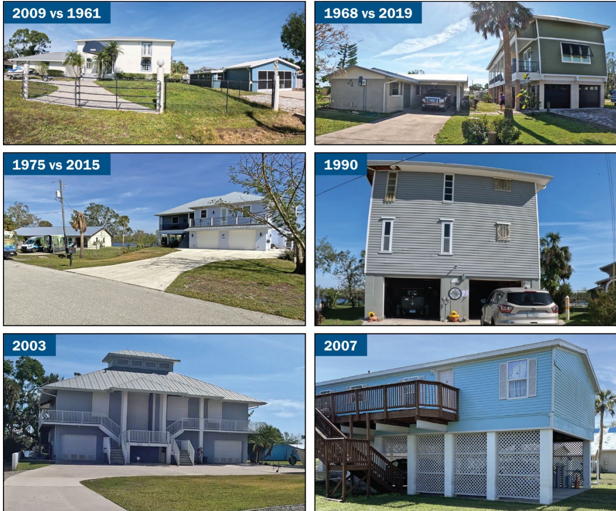
Figure 4: Representative single-family houses in Area of Interest No. 1 from 1961 to 2019
