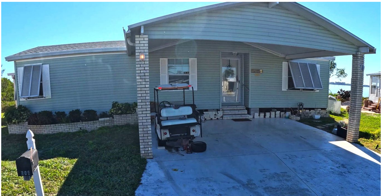
Figure 3-121: Representative manufactured home along Adam Drive that had interior flood damage, elevated approximately 1 foot above ground (Lee County, Zone AE)
