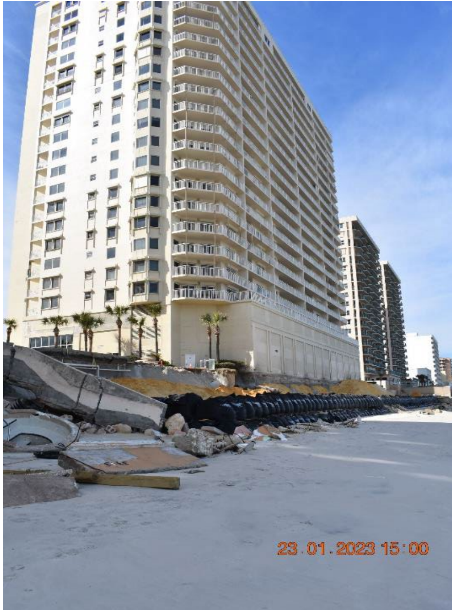
Figure 3-40: Large sediment-filled bags used to counteract further coastal erosion along an area of Daytona Beach Shores where seawalls were destroyed (Volusia County)
