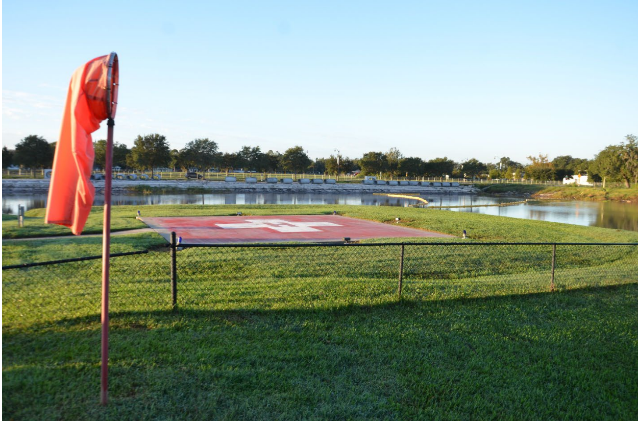
Figure 5-17: Two helipads at Osceola Regional Medical Center Trauma Center that were submerged and inoperable for at least 2 hours during Hurricane Ian (Osceola County, Zone AE)
