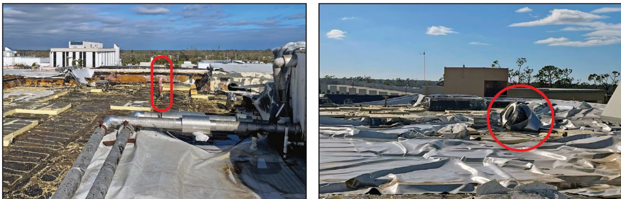
Figure 5-11: Damaged wet fire protection standpipe (left) that resulted in significant water intrusion and damaged exhaust fan and roof cover (right) (Southwest Florida)
