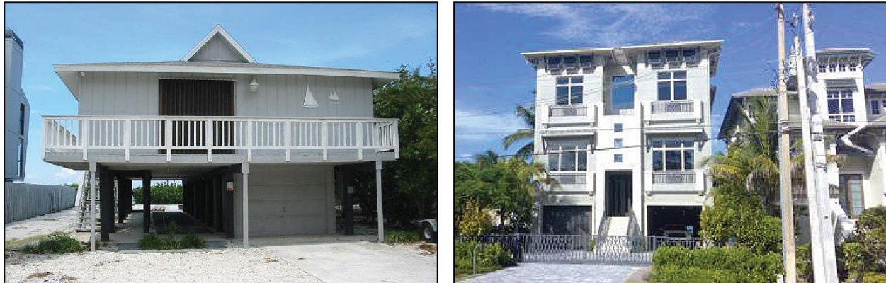
Left image shows typical 1970's construction of a single elevated level on timber piles. The right image shows typical 2010's construction of a multilevel structure using CMU block.
