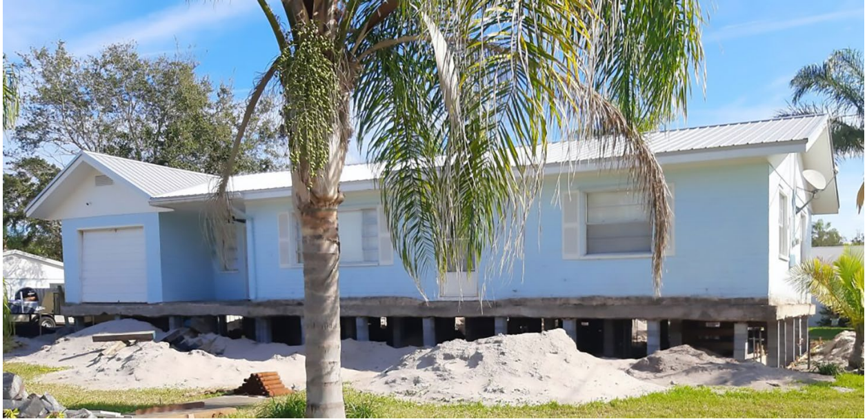
Figure 3-4: House in the process of being elevated (Volusia County, Zone AE)
