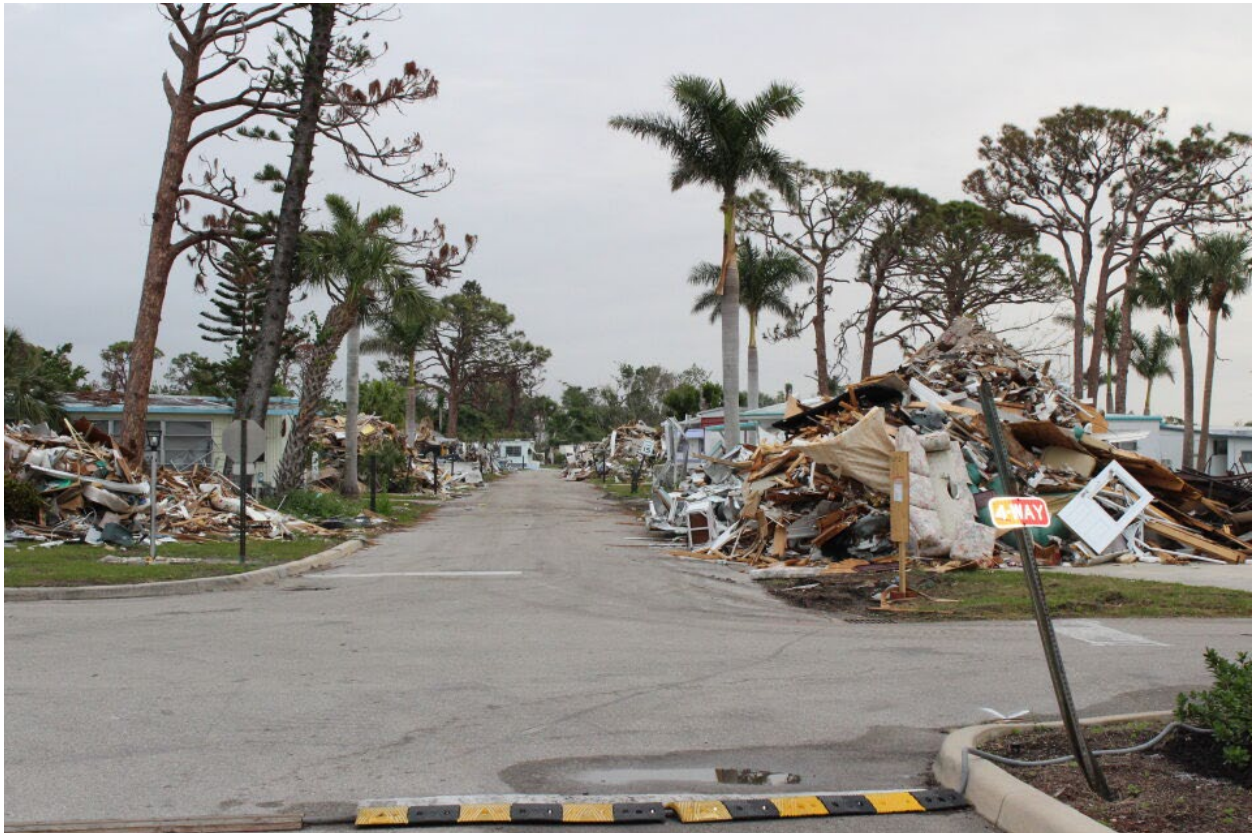
Figure 4-50: Structural damage to pre-HUD manufactured homes (EWS = 129 mph) (Lee County)
