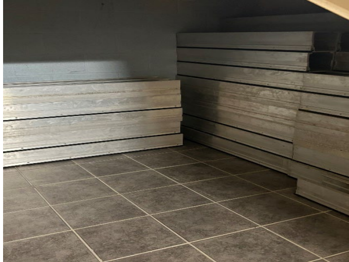
Figure 5-37: Stop logs / flood barriers stored on site when not in use (Lee County, Zone AE)
