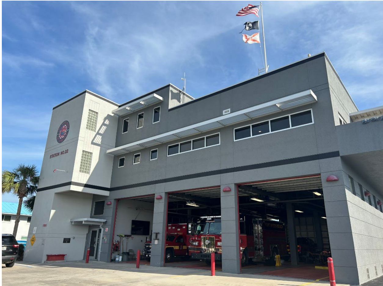
Figure 5-33: Fort Myers Beach Fire Station #32, view looking southeast (Lee County, Zone AE)
