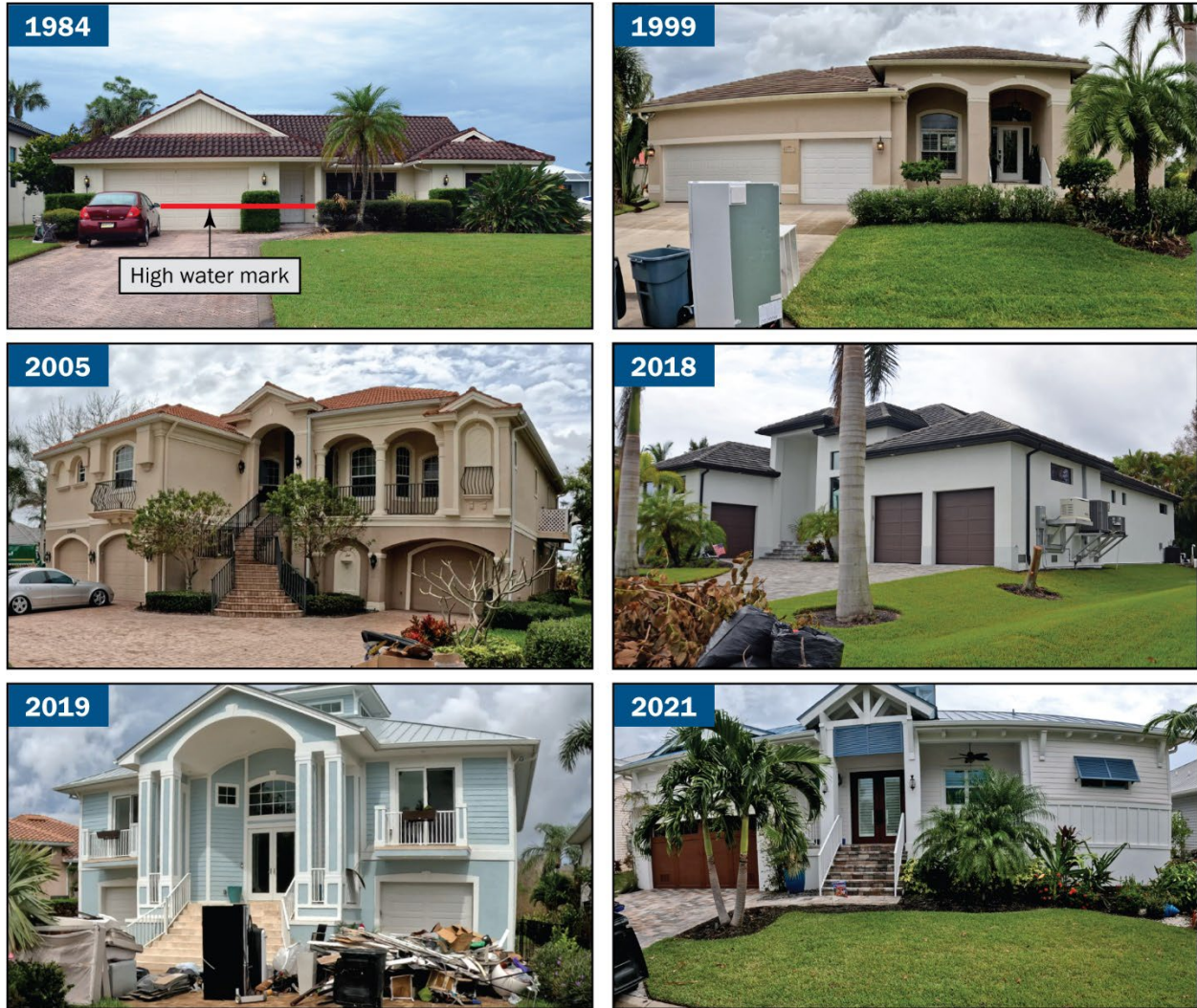
Figure 23: Representative single-family houses in Area of Interest No. 10 from 1984 to 2021
