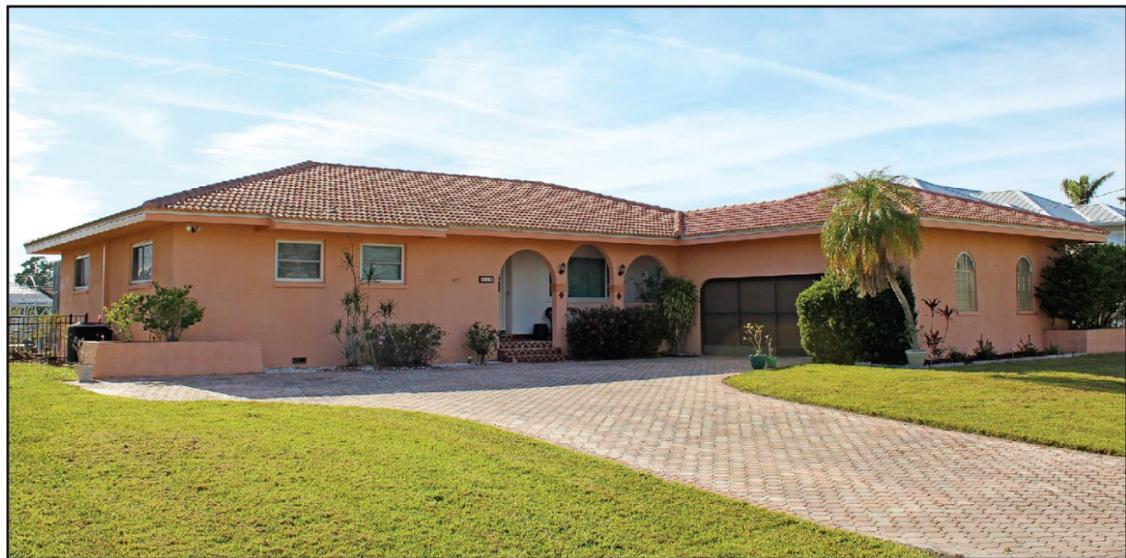
Figure 4-44: A house built in 1975 with no observable roof covering damage, a “storm-related roof replacement” permit was issued post-Hurricane Ian (EWS = 128 mph) (Port Charlotte)
