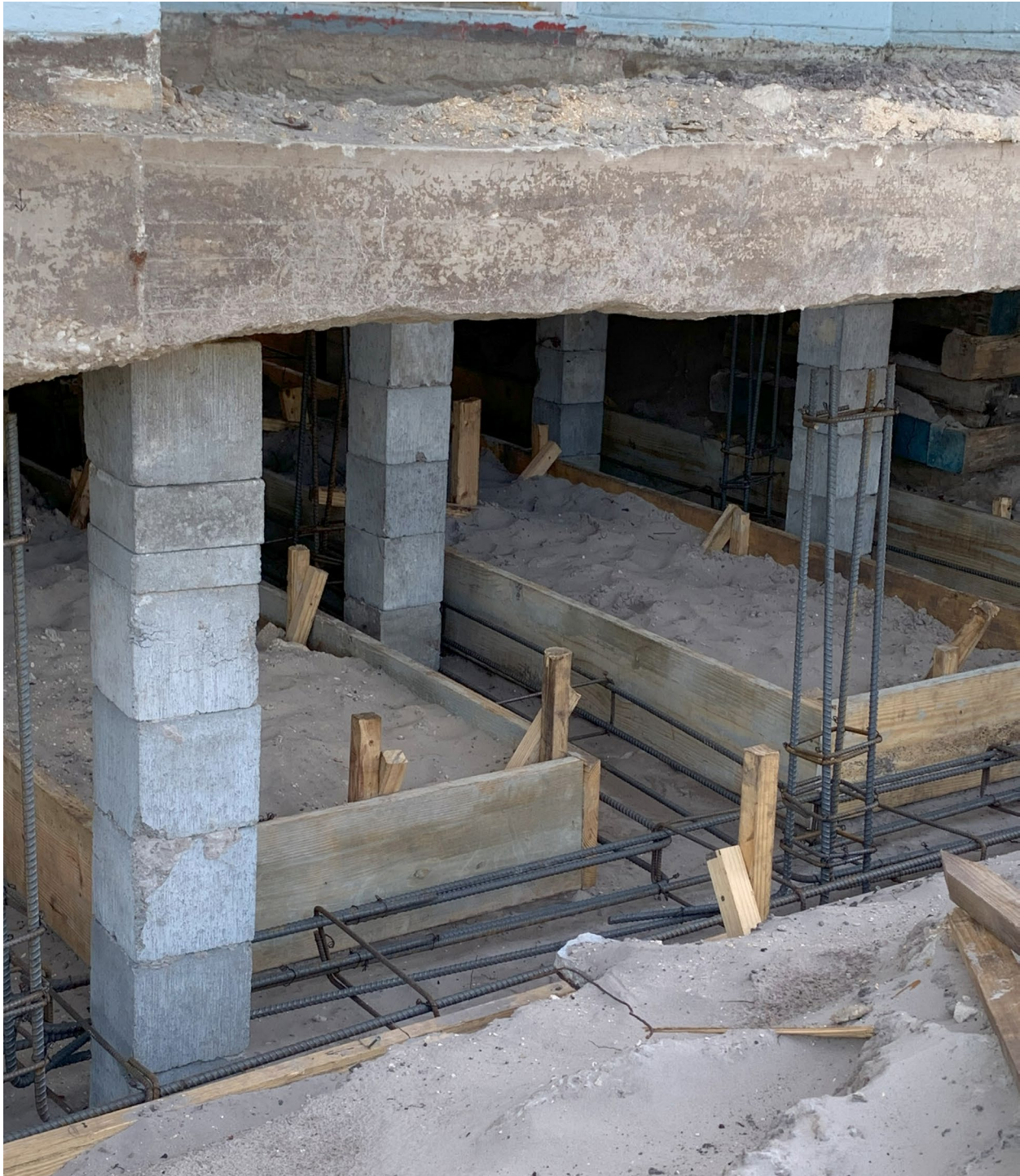
Figure 3-5: View of house elevation foundation preparation and support cribbing
