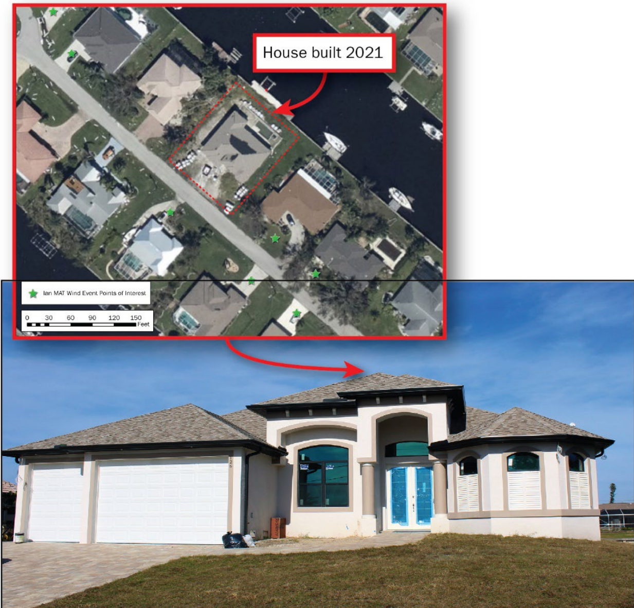
Figure 4-14: A house built in 2021 with significant asphalt shingle damage on the northeast roof slope (EWS = 127 mph; DWS = 150 mph). The inset above shows an aerial image of the house post-Hurricane Ian. (Port Charlotte)
