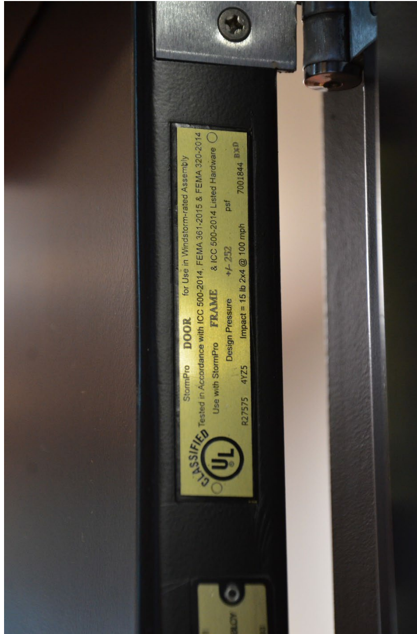
Figure 5-47: Doors to City of Naples ICC 500 EOC (Collier County, Zone AE)
