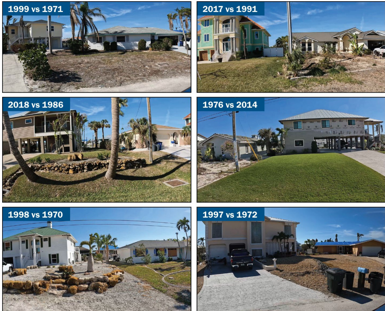
Figure 8: Representative single-family houses in Area of Interest No. 3 from 1971 to 2018
