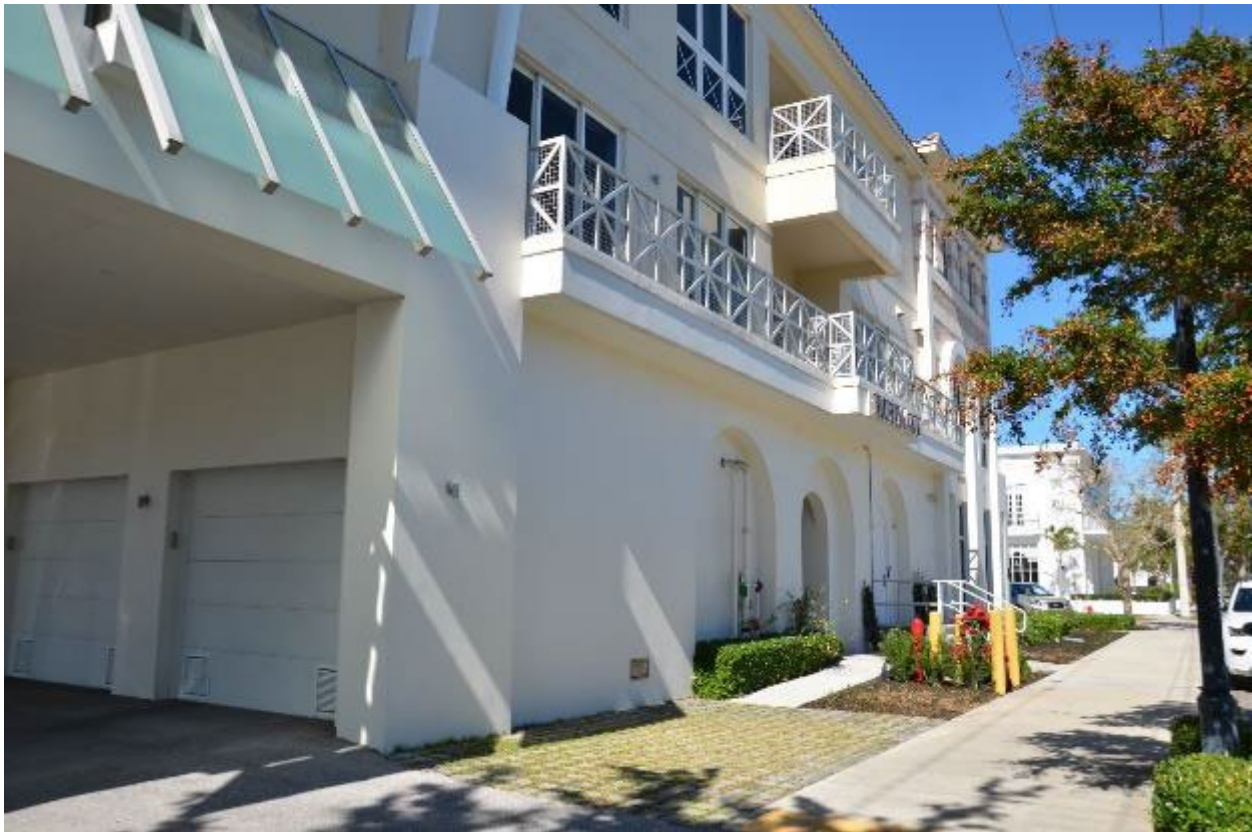
Figure 3-81: Mixed-use building with retail space and parking at grade, with residential apartments above (Collier County, Zone AE)
