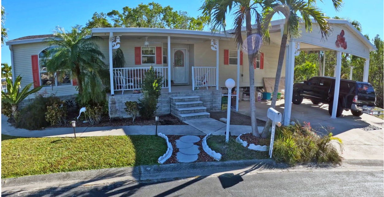
Figure 3-120: Representative manufactured home along Adam Drive that performed well, elevated approximately 3 feet above ground (Lee County, Zone AE)
