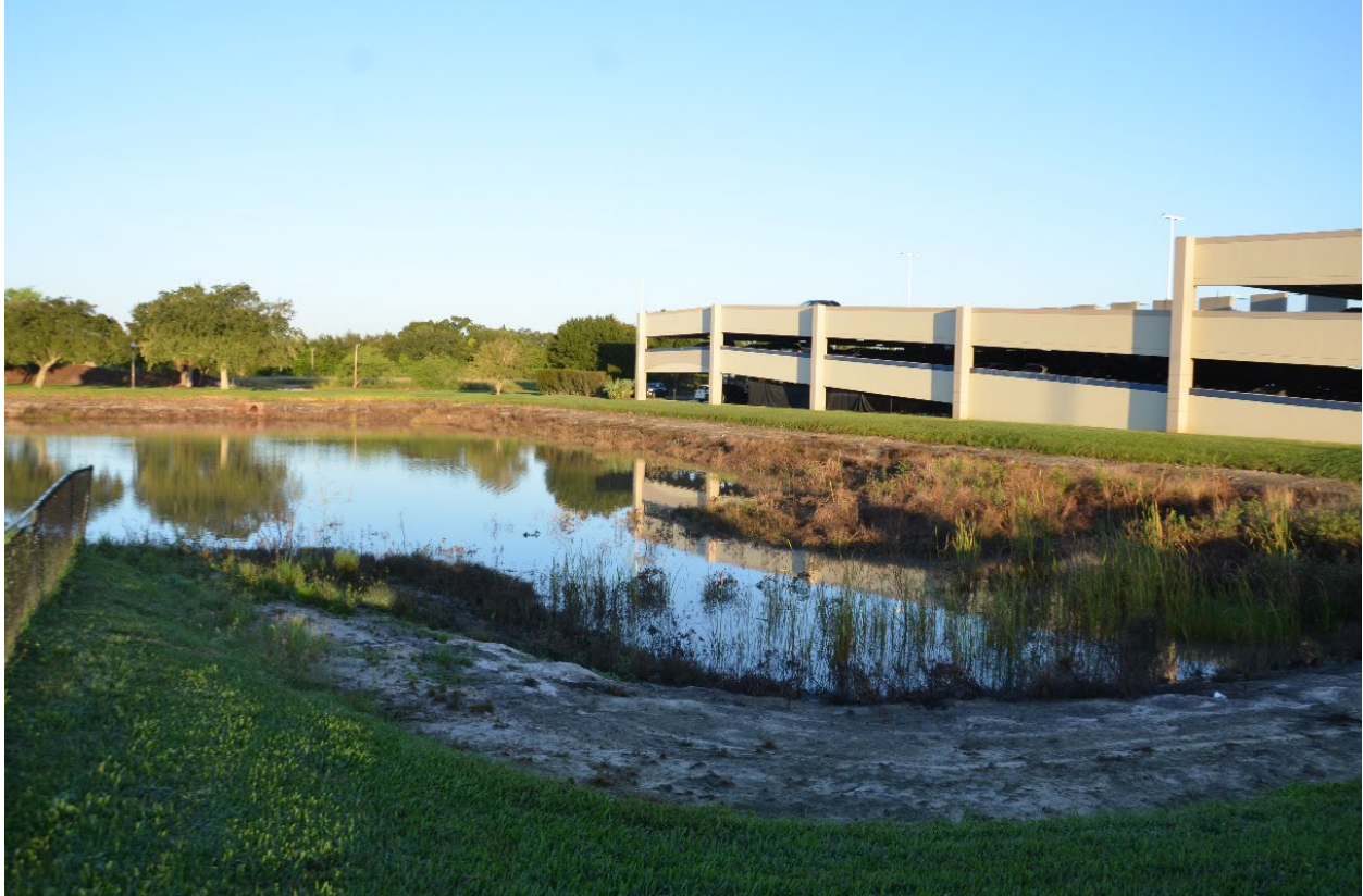
Figure 5-16: Osceola Regional Medical Center Trauma Center parking garage that had approximately 21 inches of water at ground level during Hurricane Ian (Osceola County, Zone AE)
