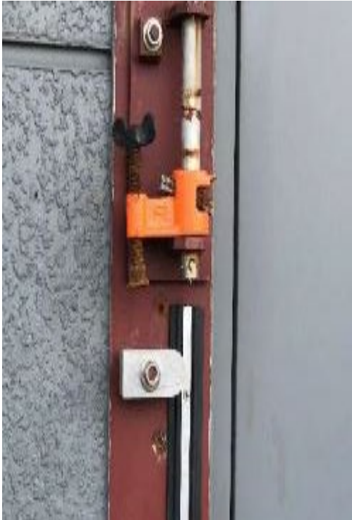
Figure 5-36: Flood barrier fastening device (Lee County, Zone AE)
