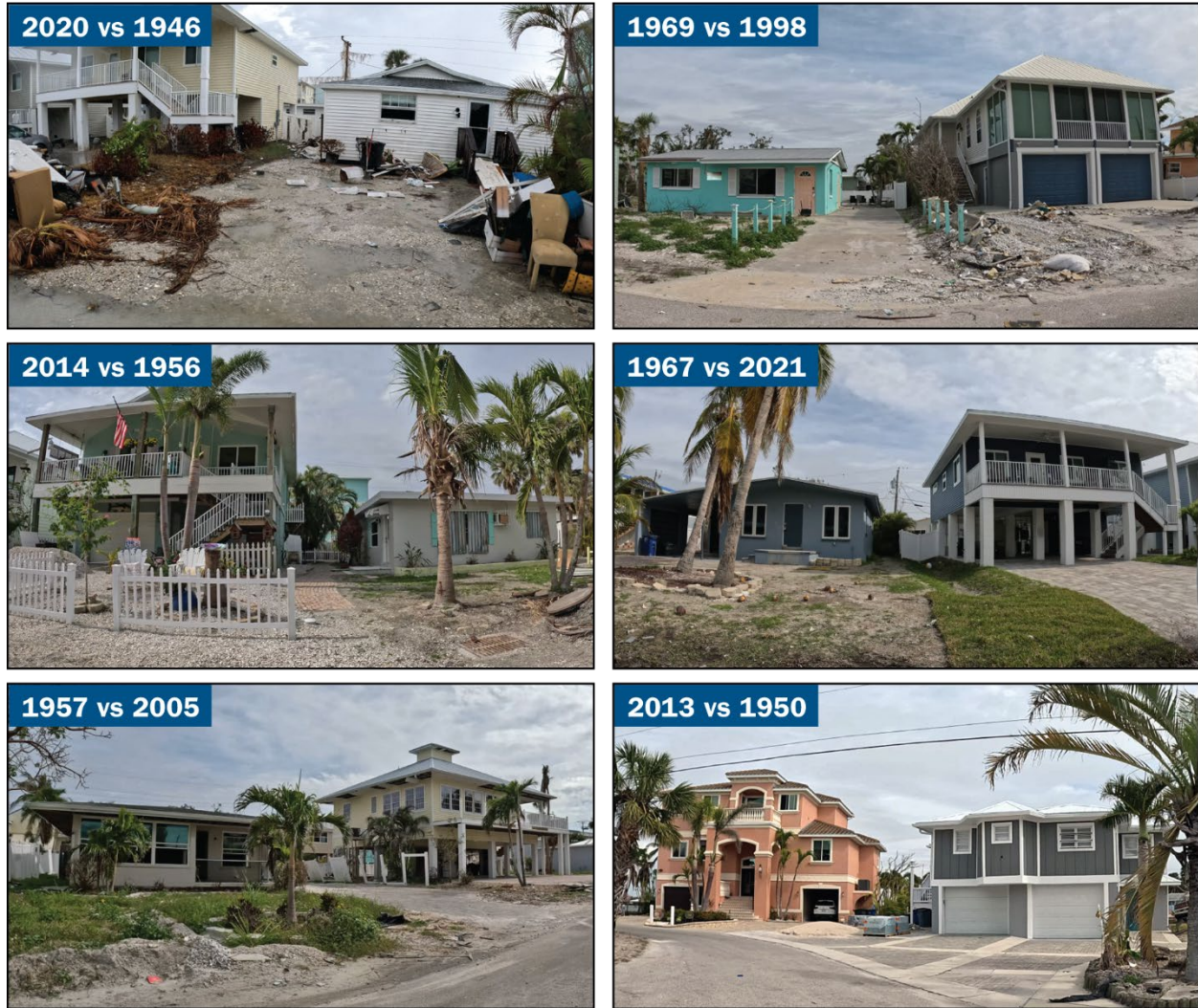
Figure 17: Representative single-family houses in Area of Interest No. 7 from 1946 to 2021
