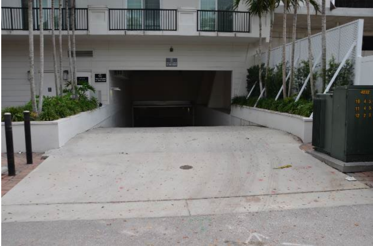
Figure 3-67: Below-grade parking with elevated ramp access in the building elevated on fill and foundation walls (Collier County, Zone AE)
