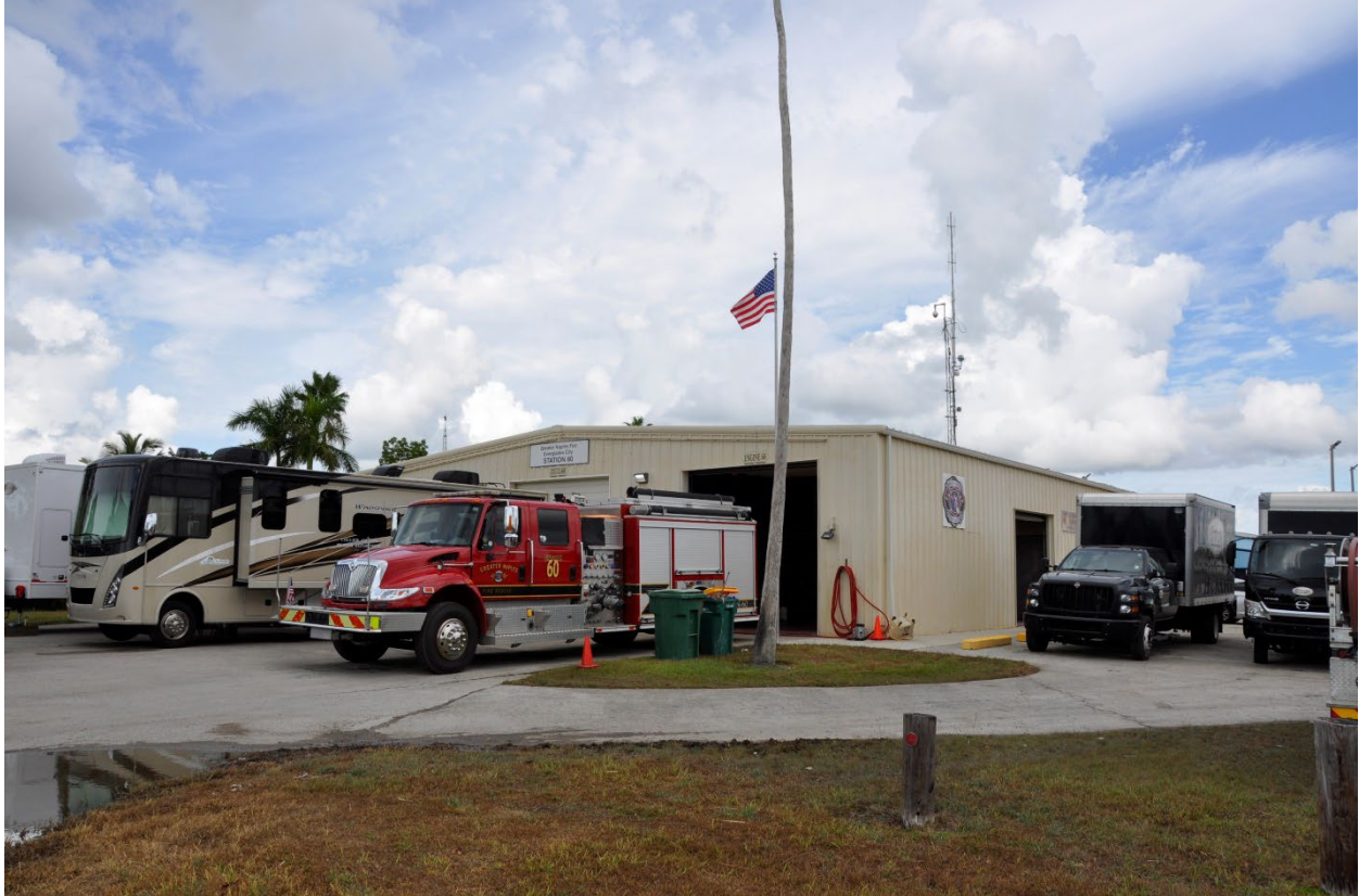
Figure 5-52: Everglades City Fire Station #60 (Collier County, Zone AE)
