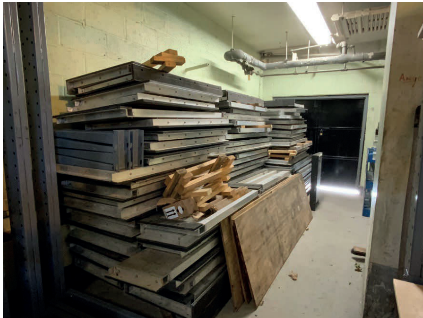
Figure 6. Dry floodproofing panels stored in basement of dry floodproofed building in NYC
