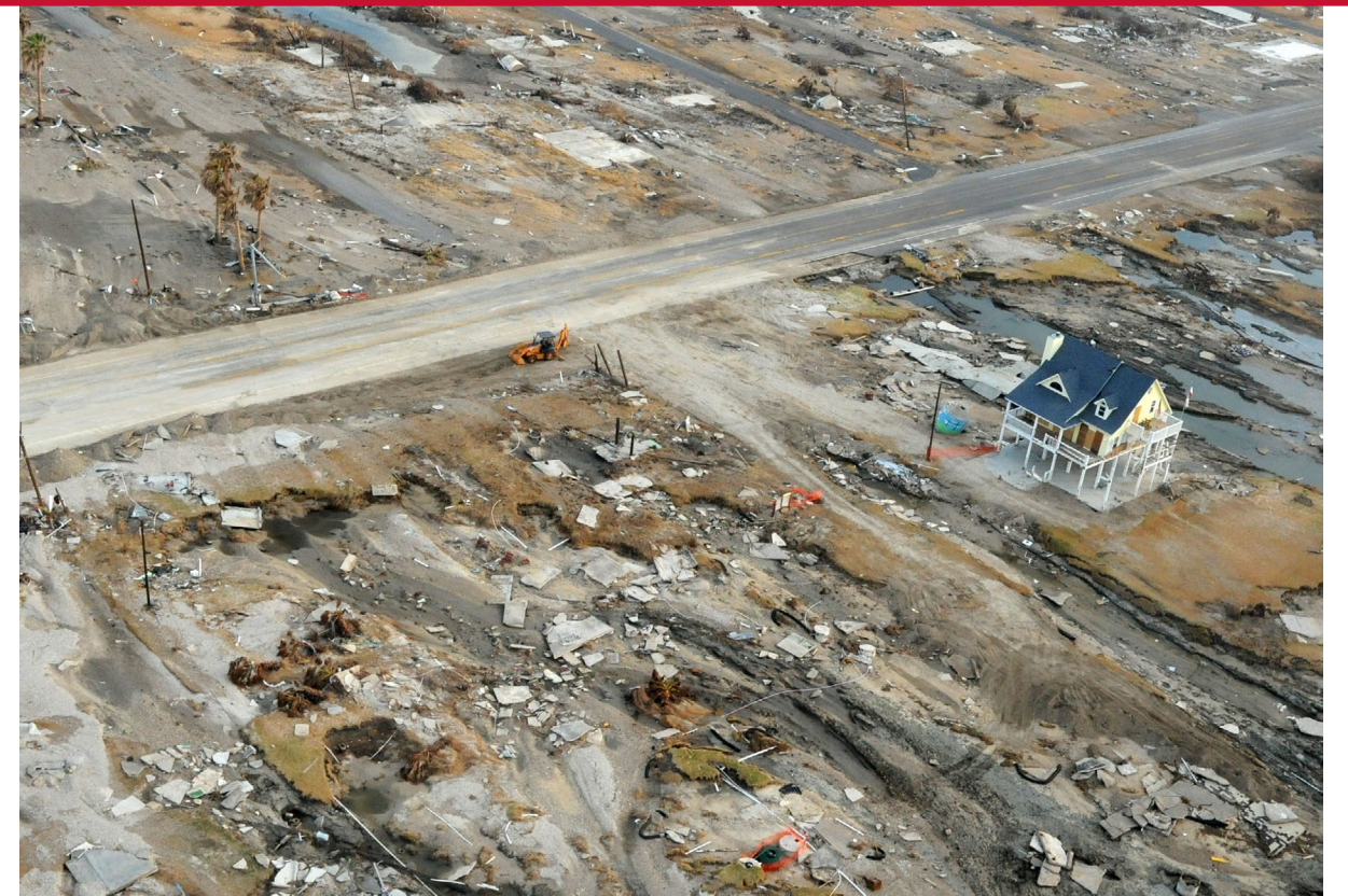
Hurricane destruction surrounding a standing house Source: Jocelyn Augusitno/FEMA / Public domain, https://upload.wikimedia.org/wikipedia/commons/5/55/Hurricane_Ike_Gilchrist_damage_edit.jpg
