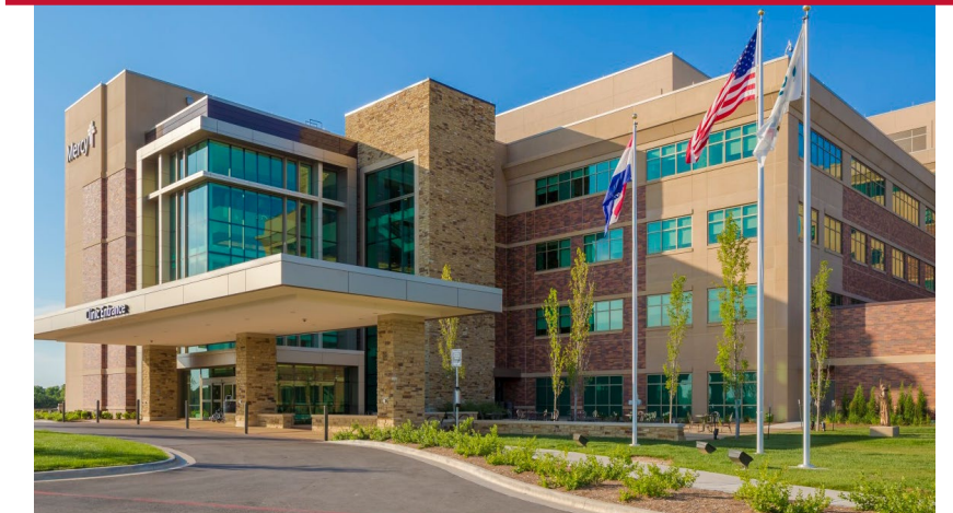
Rebuilt Mercy Hospital as it looks today
