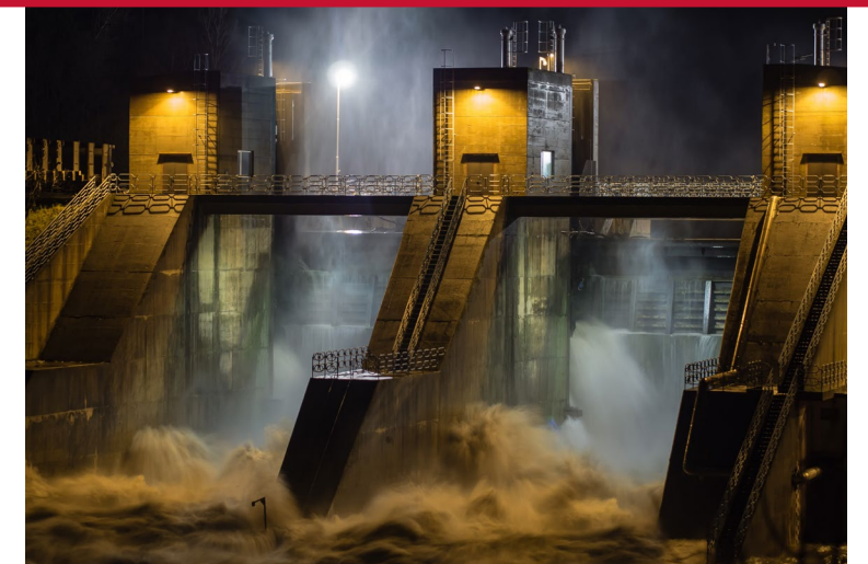
Dam releasing water during a storm
