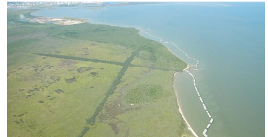
Virginia Point Wetland Restoration Project, aerial view
