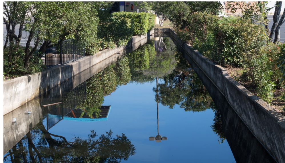
Retention pond used to manage stormwater runoff
