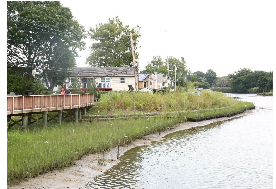
Natural coastal buffer designed to reduce erosion and sedimentation and improve wildlife habitat
