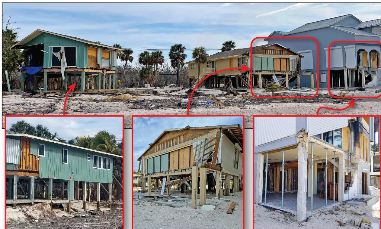
Figure 2: Image (top) shows waterfront houses damaged by coastal flood effects such as waves and velocity in Bonita Springs, Florida. Image (bottom left) shows siding damage above the lowest floor and significant scour, image (bottom center) shows complete loss of a deck as well as damage to glass doors, image (bottom right) shows structural damage to a concrete column and complete loss of a porch.
