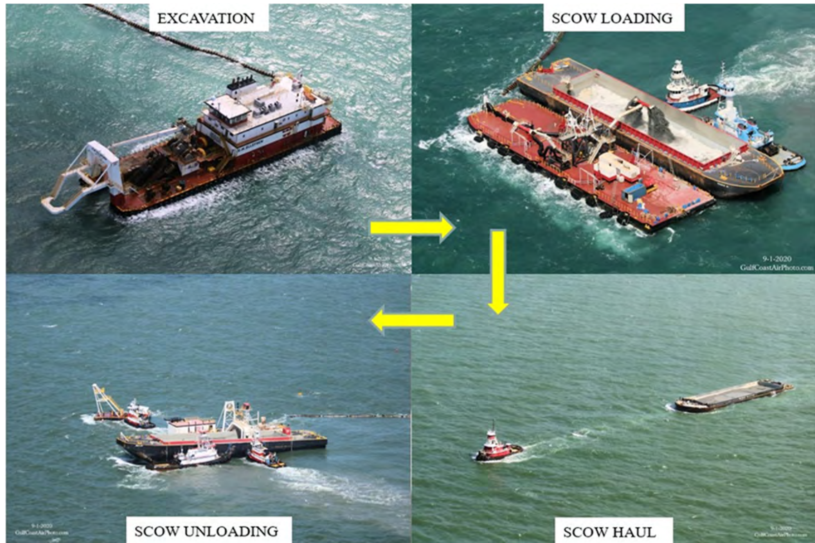
Figure 3. Typical Cutterhead Dredging, Scow Barge Transport, and Hydraulic Unloading
