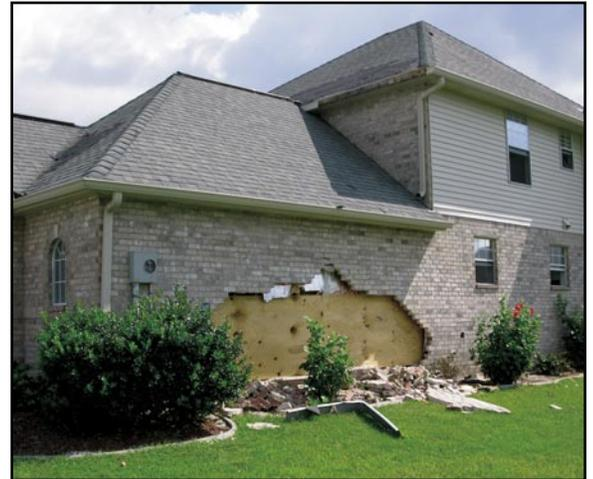
**Figure 1. Failed brick veneer. Plastic foam wall sheathing was installed over the wood studs (plywood was temporarily installed after the brick failure).**
