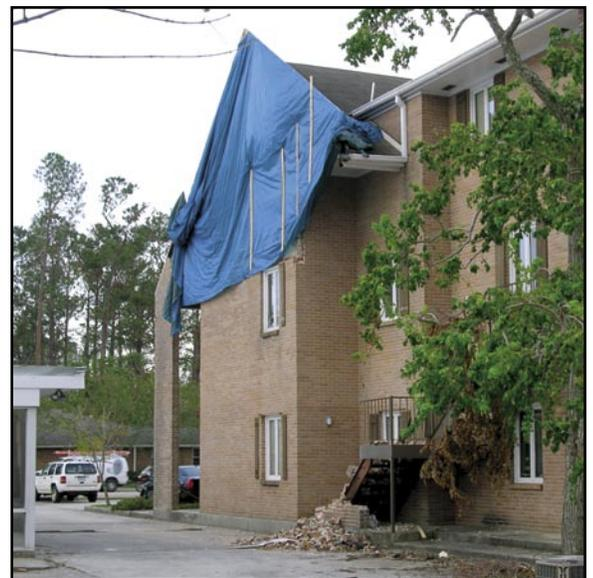
**Figure 2. The upper portion of the brick veneer at this apartment building collapsed. Pedestrian and vehicular traffic in the vicinity of the damaged wall were vulnerable to injury and damage if remaining portions of the wall were to collapse during subsequent storms.**
