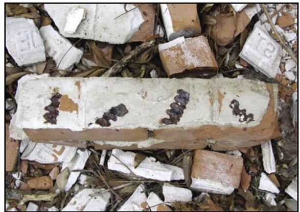
**Figure 6. There were several ties in this portion of the wall, but they failed due to severe corrosion.**
