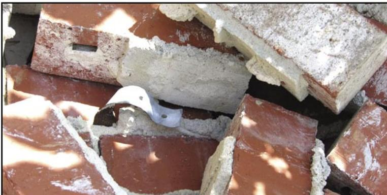
**Figure 3. This tie remained embedded in the mortar joint while the smooth-shank nail pulled from the stud.**
