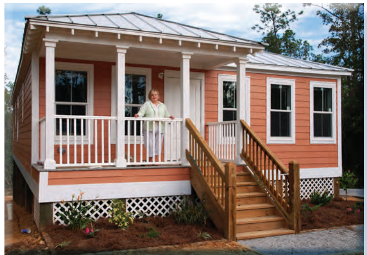
Diamondhead, MS, October 22, 2008 -- Carol O'Brien stands on the porch of a Mississippi Cottage, newly made permanent, that she will move into once she has met her sweat equity hours requirement for Habitat for Humanity. FEMA's Long Term Community Recovery Staff in Mississippi teamed up with Bay-Waveland Area Habitat for Humanity to create a "Coastal Cottage," adapted from an Alternative Housing Pilot Program Cottage. The modifications increase the square footage of the modular unit, meet local zoning requirements and place the cottage on a permanent foundation. Jennifer Smits/FEMA.
