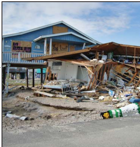
Houses on the beachfront row became battering rams during Hurricane Ike, wrecking neighboring homes.
