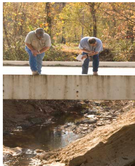
Michael Englehart, FEMA project specialist, looks at the damage done to a bridge in St. Francis County, Ark., with James Bradford, the county's director of road maintenance.
