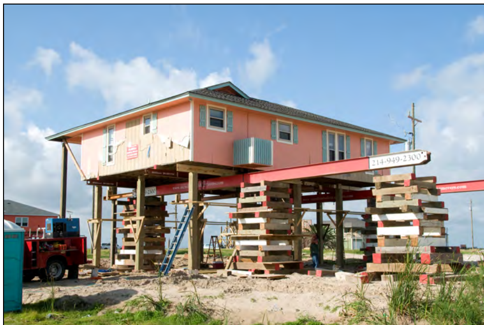
A home being elevated to comply with new requirements for homes being built or repaired in the area devastated during Hurricane Ike. Source: FEMA Photo Library
