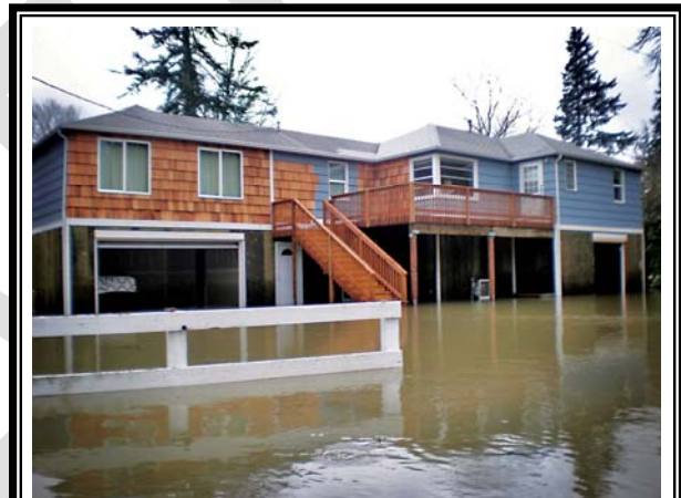
This Snoqualmie home was elevated according to the NFIP criteria and did fine during the 2006 flood.
