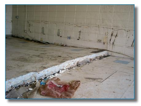
Figure 4-23: Cracked concrete floor slab at Charles B. Murphy Elementary School
