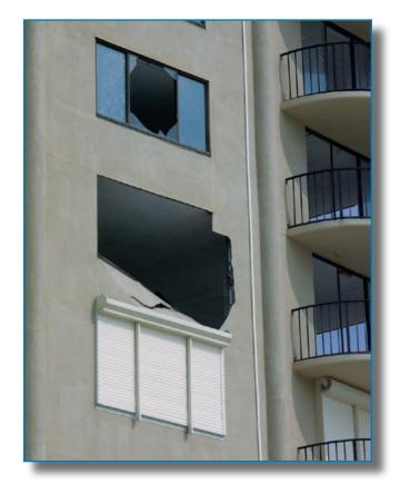
Deploying accordion or panel shutters a few stories above grade is expensive. Although motorized shutters have greater initial cost, their operational cost should be lower. Other options for providing missile protection on upper levels include replacing the existing as-
