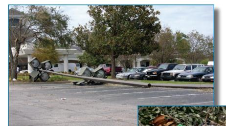
Figure 3-78: Collapsed hospital light fixtures caused by severe corrosion (see inset). Hurricane Ivan (Florida, 2004)
