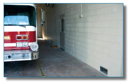
Figure 2-35: The enclosed entry and storage area to the right of the fire truck bays were retrofitted with flood openings.
