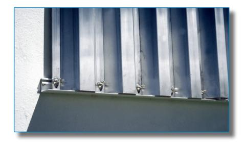
Figure 3-113: The lower window assembly was protected with a motorized shutter. Hurricane Ivan (Florida, 2004)
