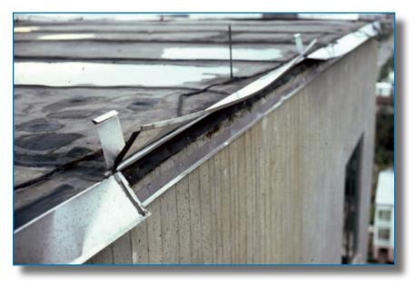
Figure 3-62: The metal edge flashing disengaged from the continuous cleat and the vertical flange lifted. Hurricane Hugo (South Carolina, 1989)
