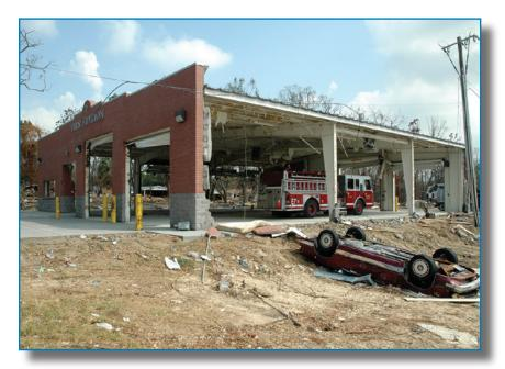
Figure 4-40: Exterior walls on the Gulfport Fire Station #7 washed away by the storm surge
