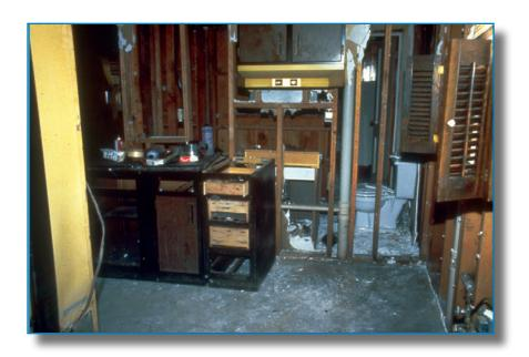
Figure 2-19: Water damage and mold growth extend above the water line
