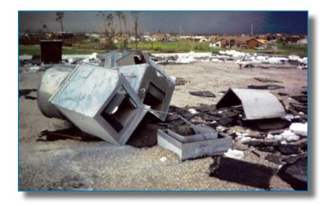
Figure 3-68: This gooseneck was attached with only two small screws. A substantial amount of water was able to enter the building during Hurricane Francis. (Florida, 2004)
