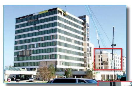
Figure 3-56: EIFS debris blown off the hospital building in the background (red square) broke numerous windows in the MOB in the foreground. Hurricane Ivan (Florida, 2004)
