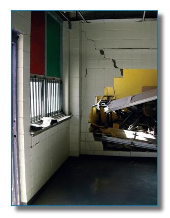
**Buoyancy and uplift:** If below-grade areas are essentially watertight, buoyancy or uplift forces can float a building out of the ground or rupture concrete floors (see Figure 2-15). Buildings that are not adequately anchored can be floated or pushed off foundations. Although rare for large and heavy critical facility buildings, this is a concern for outbuildings and portable (temporary) units.
