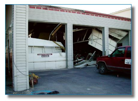
Figure 4-45: Damaged apparatus bay doors at Port Sulphur Volunteer Fire Department.
