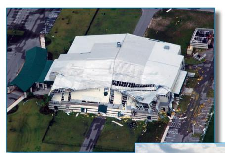
Figure 3-22: Collapse of a large portion of a new pre-engineered metal building used as a shelter for approximately 1,400 people. Hurricane Charley (Florida, 2004)
