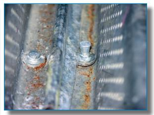
Figure 3-24: Looking down at a sidelap of a deck attached with powder-driven pins. The washer at the top pin blew through the deck.
