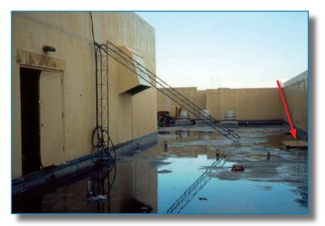
Figure 3-118: The antenna at this hospital collapsed and was whipped back and forth across the roof membrane. Hurricane Andrew (Florida, 1992)
