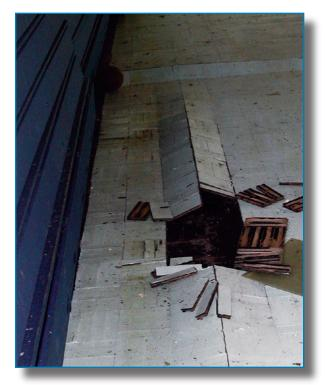
Figure 2-17: This parquet wood gymnasium floor was damaged by dimensional changes due to saturation. Hurricane Katrina (2005)
