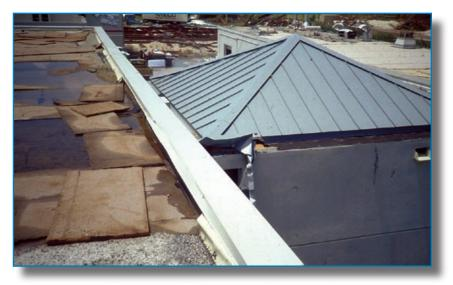
Figure 3-10: The irregularity created by the stair tower (covered with a metal roof) caused turbulence resulting in wind speed-up and roof damage. Hurricane Andrew (Florida, 1992)
