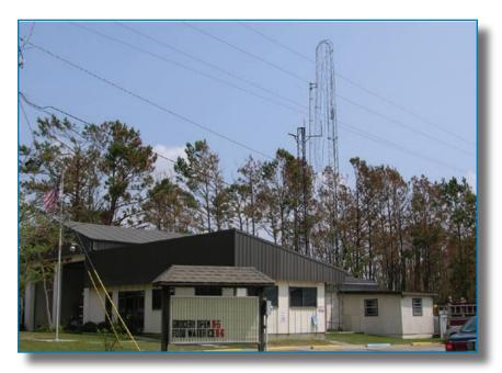
Figure 3-80: The antenna tower at this fire station buckled. Hurricane Katrina (Mississippi, 2005)
