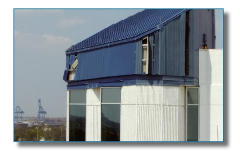
Figure 4-5: Canopy soffit damage at West Jefferson Medical Center
