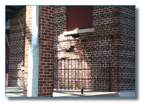
Figure 4-26: Cracked brick veneer at St. Stanislaus High School
