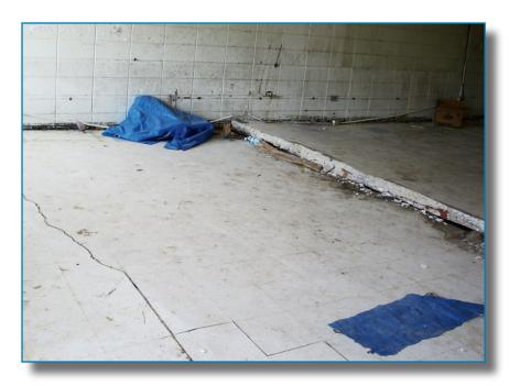
Figure 2-15: Concrete floor ruptured by hydrostatic pressure (buoyancy). Hurricane Katrina (2005)
