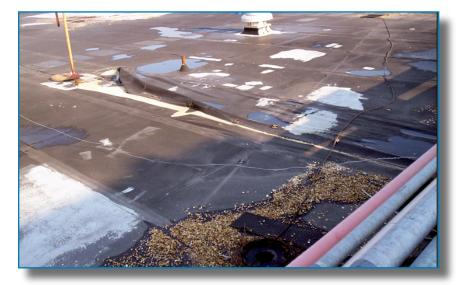
Figure 4-7: Roof membrane starting to peel off at Hancock Medical Center.
