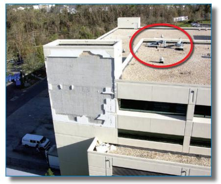
Wind-borne EIFS debris can be devastating to unprotected glazing. At the hospital shown in Figure 3-56, the hospital's original concrete wall panels had been furred with metal hat channels and covered with EIFS. In a large corner area, the EIFS and gypsum board substrate blew off the hat channels and broke a large number of windows in the multi-story connecting walkway
