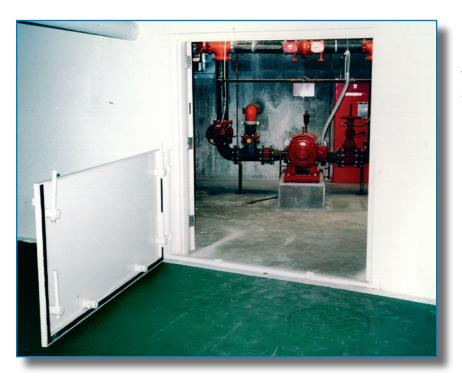
Figure 2-31: Equipment room with watertight door
