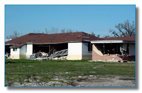
Figure 4-29: Damaged non-loadbearing walls at Charles B. Murphy Elementary School
