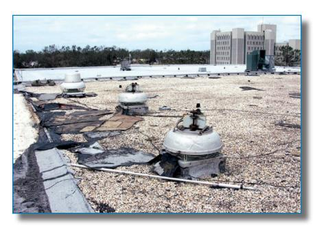
Figure 3-70: Cowlings blew off two of the fans on a police building that housed the county's EOC. Hurricane Ivan (Florida, 2004)
