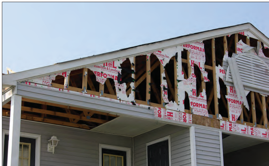
Figure 5-28. Loss of vinyl siding and foam insulation at a gable end wall. Note the missing vinyl soffit (estimated wind speed: 130 mph. Long Beach, Mississippi).
