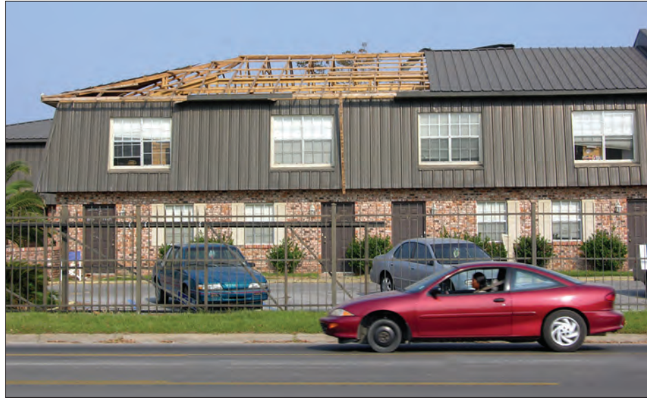
Figure 5-63. Blow-off of nailers caused these panels to progressively fail. The nailers were installed directly over the trusses and, with loss of the panels, rainwater was free to enter the building (estimated wind speed: 105 mph. Pascagoula, Mississippi).
