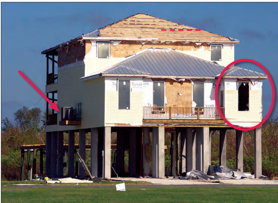
Figure 5-62. Blow-off of one of the nailers (dotted line) caused these panels to progressively fail. Note the cantilevered condenser platform (arrow), a good practice, and the broken window (circle). The house was located in Exposure C (estimated wind speed: 130 mph. St. Bernard Parish, Louisiana).
