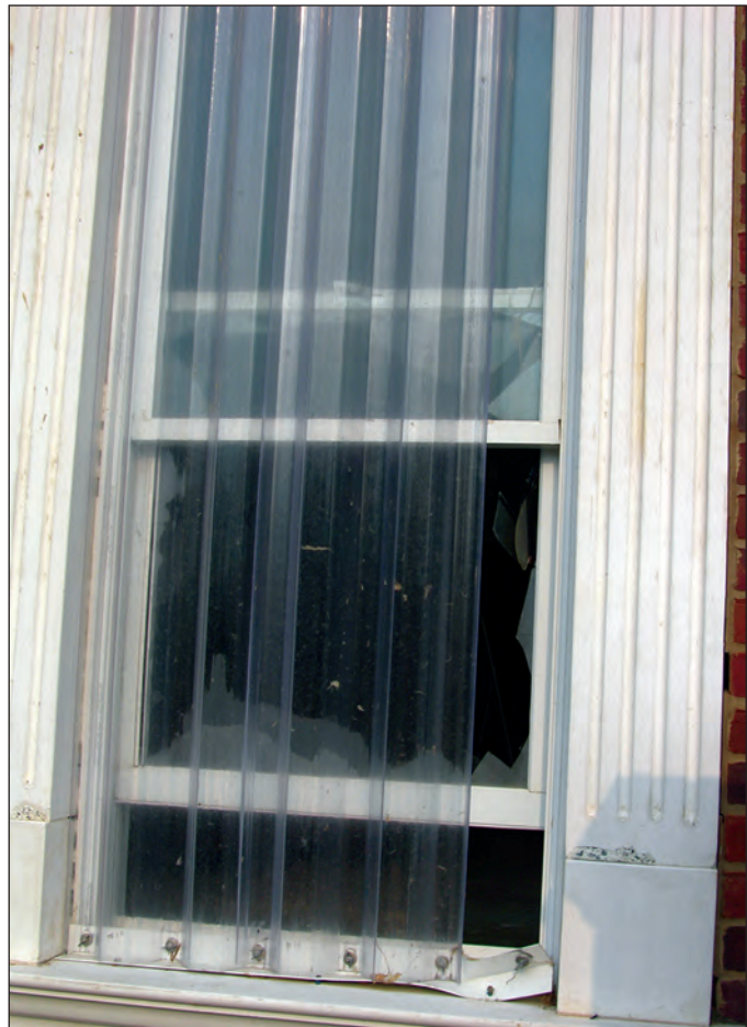
Figure 5-100. This plastic shutter did not completely cover the window. The lower window was broken (estimated wind speed: 105 mph. Pascagoula, Mississippi).
