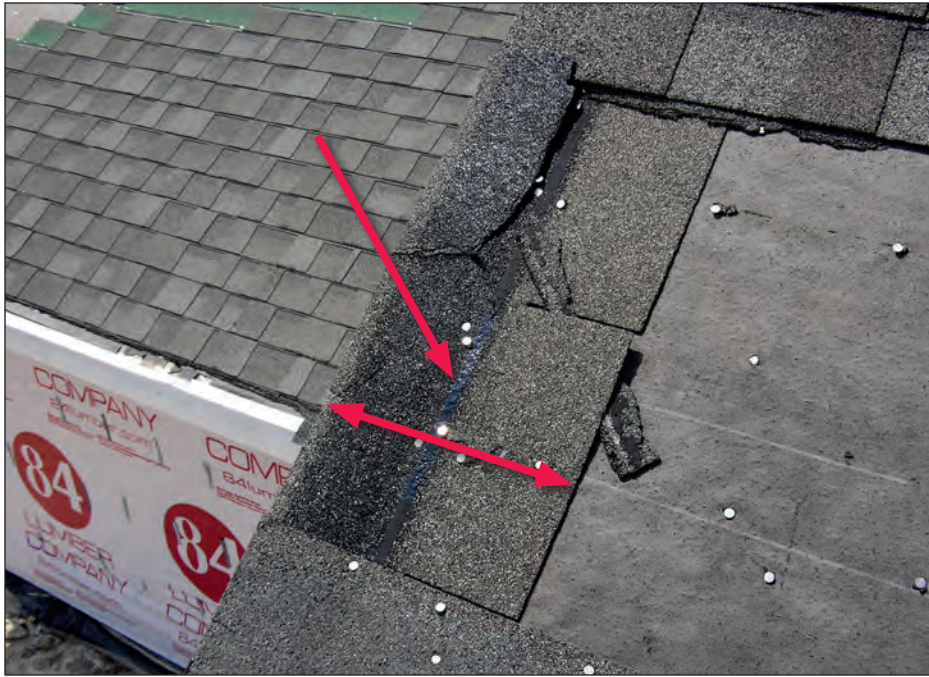
Figure 5-42. Blow-off of shingles at a new house under construction. A bleeder strip (double-arrow) was used along the rake. Note that the tab of the overlying shingle cannot make contact with the bleeder's self-seal adhesive (upper arrow) (estimated wind speed: 125 mph. Waveland, Mississippi).
