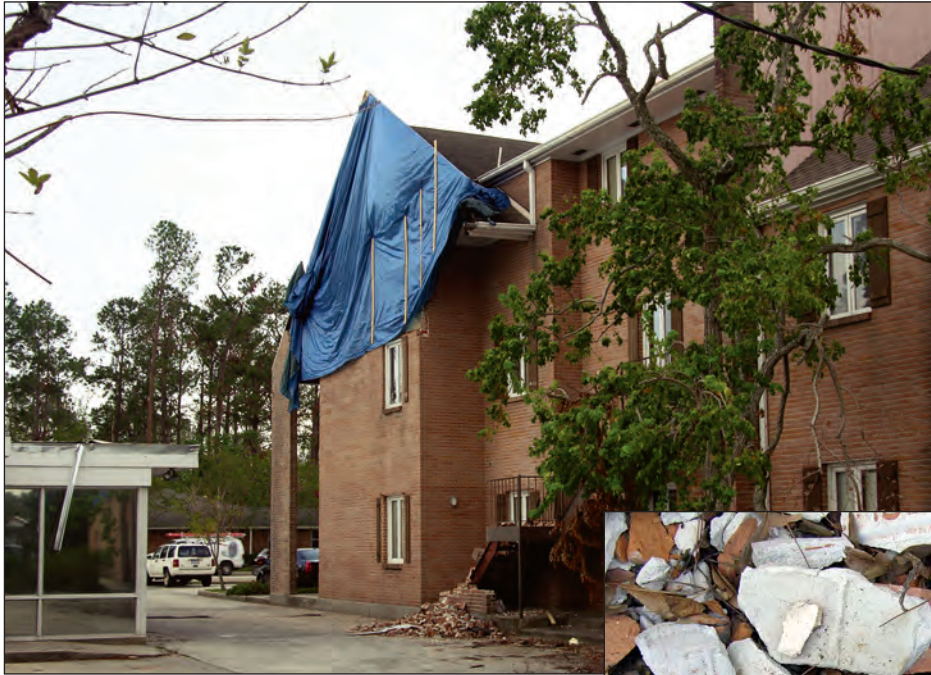
Figure 5-17. Partial collapse of brick veneer at an apartment building; the ties were corroded (inset) (estimated wind speed: 115 mph. Slidell, Louisiana).
