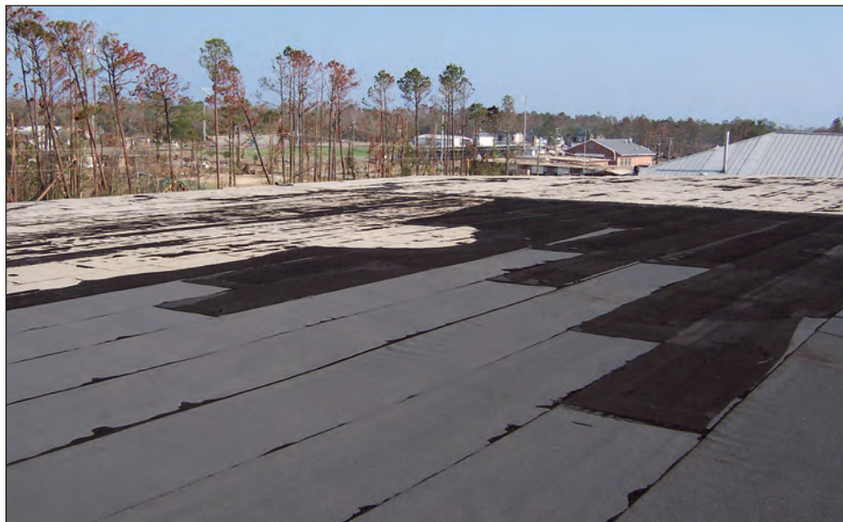
Figure 5-70. The modified bitumen membrane failure at this school was caused by lifting of the edge nailer (estimated wind speed: 130 mph. Pass Christian, Mississippi).
