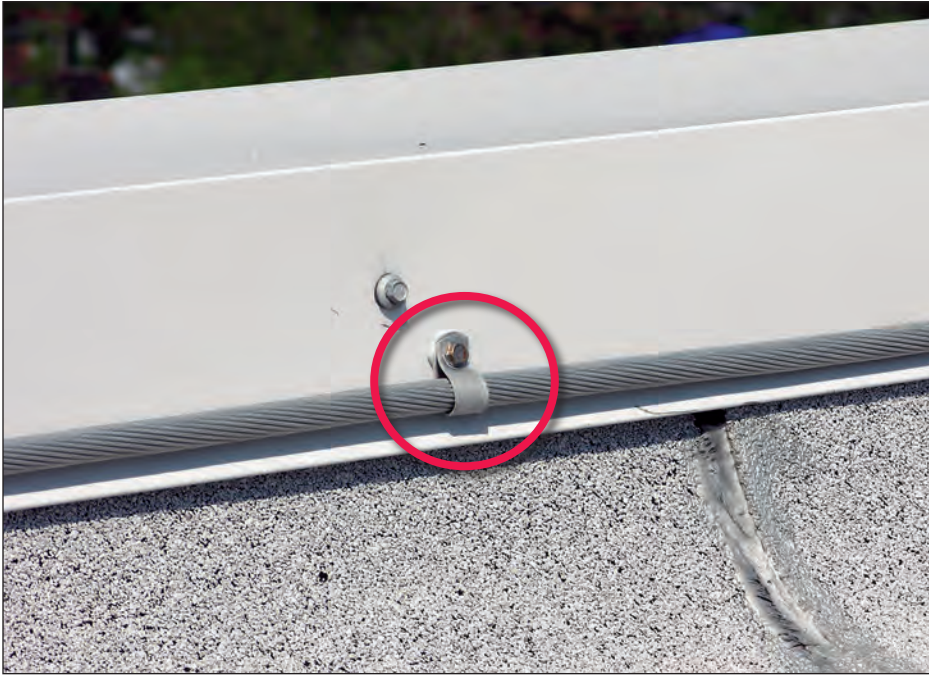
Figure 5-126. Screw-attached looped connectors were used to anchor this conductor (estimated wind speed: 130 mph. Gulfport, Mississippi).
