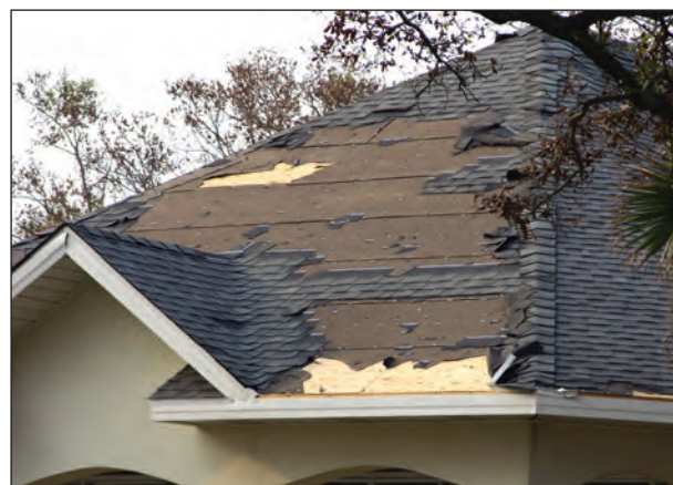
Figure 5-39. These two failures likely initiated at the eave due to an incorrectly installed starter course. Note that, at both roofs, a portion of the underlayment and some of the hip shingles were blown away (estimated wind speed: 115 and 105 mph. Slidell, Louisiana, and Pascagoula, Mississippi, respectively).
