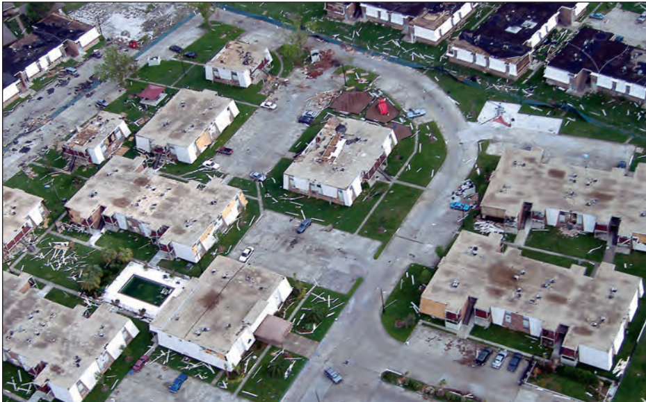
Figure 5-3. A substantial amount of siding (the white lines scattered around the ground) blew off this housing complex (estimated wind speed: 105 mph. Harvey, Louisiana area).
