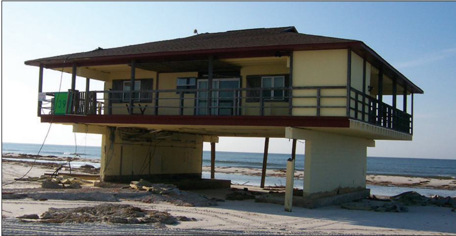
Figure 10-3. Home constructed on solid, shore- perpendicular foundation walls. The walls are supported by reinforced concrete beams placed on driven piles (Dauphin Island, Alabama).
