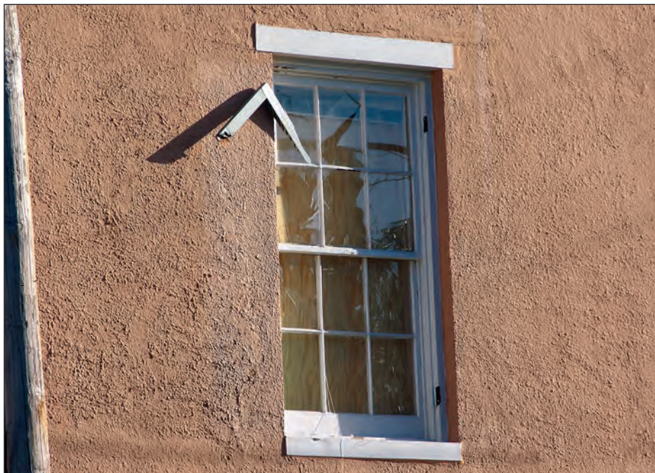
Figure 5-76. This window was broken by a fragment from a shutter (estimated wind speed: 105 mph. New Orleans, Louisiana).
