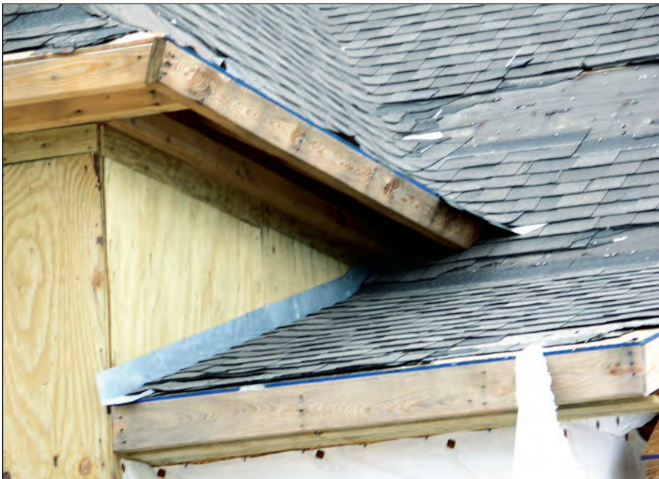
Figure 5-53. Continuous metal flashing at the roof-to-wall intersection of a house under construction. This detail is susceptible to leakage and subsequent dry rot of the deck sheathing (estimated wind speed: 115 mph. Slidell, Louisiana).
