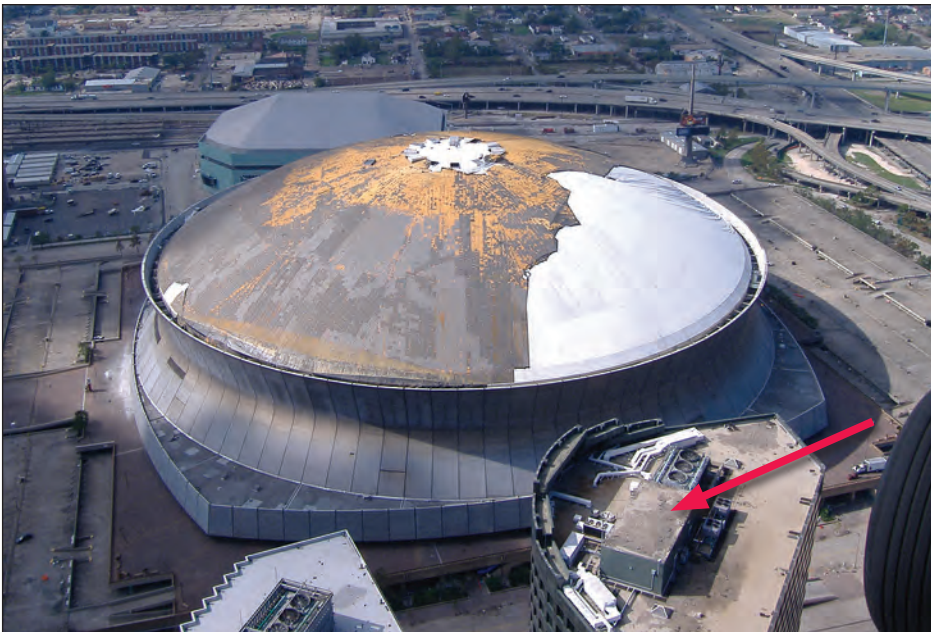
Figure 5-89. Aggregate was scoured on the main roof of Building S5 and blown from the penthouse (red arrow). The building to the left of S5 did not have an aggregate surfaced roof, nor did the lower roofs of the Superdome (estimated wind speed: 105 mph. New Orleans, Louisiana).
