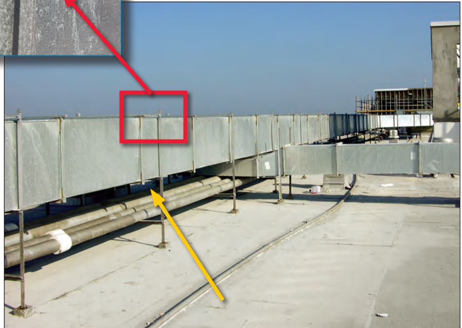
Figure 5-117. Opposite view of Figure 5-116. The ducting on either side of the fan was blown away (red arrows) (estimated wind speed: 120 mph. Biloxi, Mississippi).
