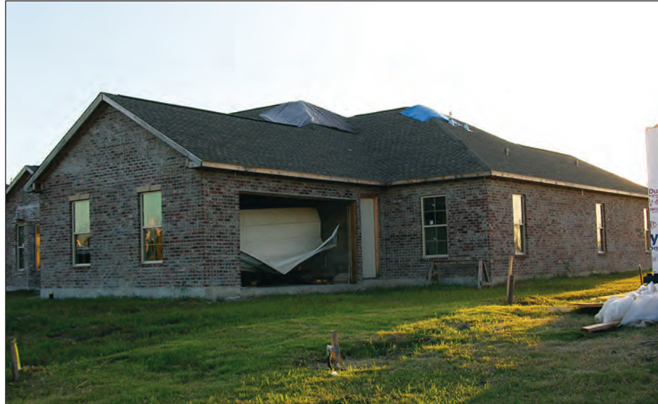
Figure 5-6. Positive pressure blew this garage door from its tracks. At some other residences, negative pressure blew doors outward. Note the damage to the asphalt shingles (estimated wind speed: 110 mph. Belle Chase, Louisiana).
