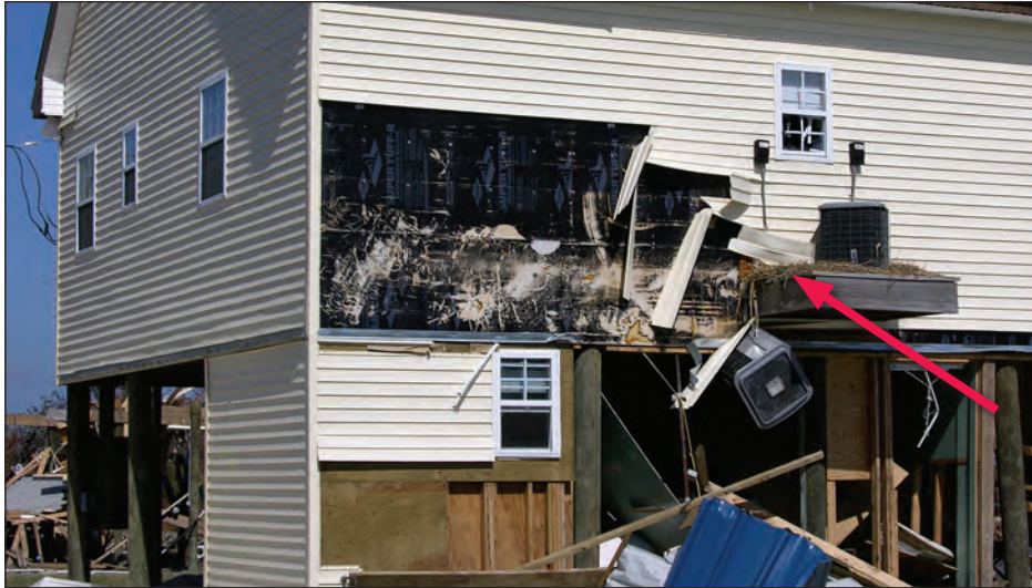
Figure 5-109. One of the condensers was blown off this cantilevered platform (estimated wind speed: 120 mph. Shell Beach, Louisiana).
