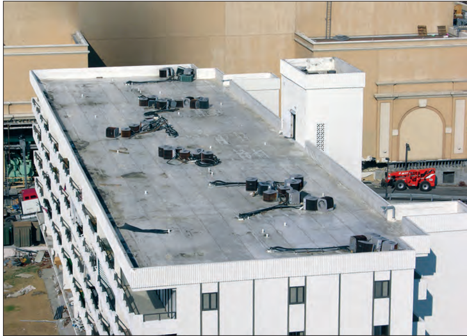
Figure 5-111. These displaced condensers had been placed on wood sleepers that rested on the roof membrane. Sleepers do not provide resistance to uplift or lateral wind loads (estimated wind speed: 120 mph. Biloxi, Mississippi).
