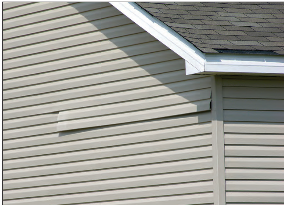
Figure 5-30. When a panel becomes unlatched, it becomes very susceptible to blow-off (estimated wind speed: 120 mph. Ocean Springs, Mississippi).
