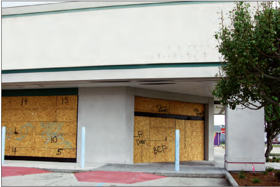
Figure 5-98. Pre-cut OSB shutters (estimated wind speed: 115 mph. Slidell, Louisiana)
