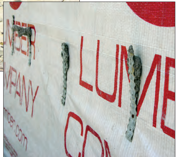
Figure 5-15. Collapsed brick veneer wall that was under construction. Several of the ties had not been embedded into the mortar joints (square/inset) (estimated wind speed: 125 mph. Waveland, Mississippi).
