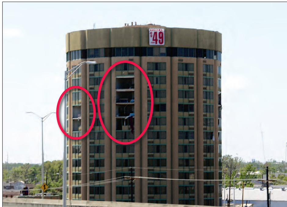
Figure 5-14. Collapse of non-load- bearing walls at a hotel (estimated wind speed: 105 mph. New Orleans, Louisiana)
