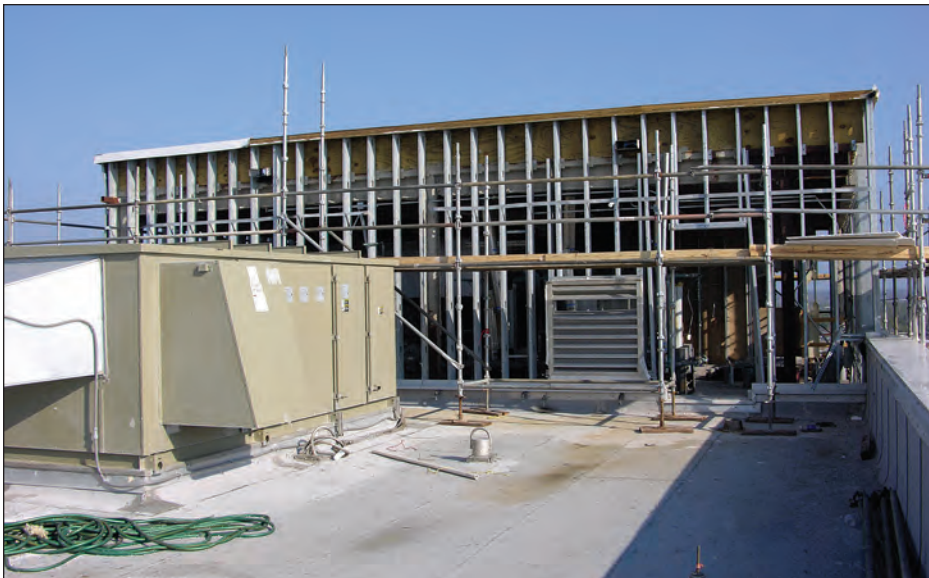
Figure 5-10. Loss of EIFS on penthouse of a new 13-story building in Exposure C. The gypsum board was attached with irregularly spaced screws and detached from the steel studs (estimated wind speed: 120 mph. Biloxi, Mississippi).
