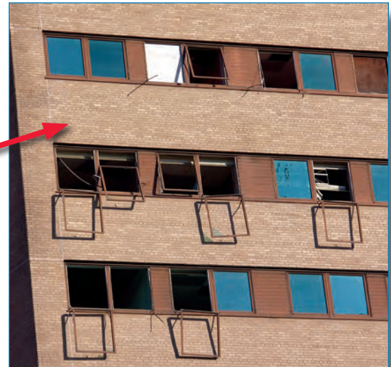
Figure 5-105. Wind pressure caused frame failure at several windows in this building (estimated wind speed: 105 mph. New Orleans, Louisiana).
