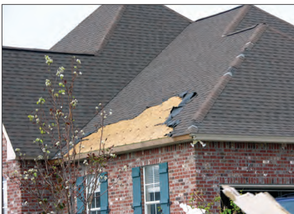
Figure 5-39. These two failures likely initiated at the eave due to an incorrectly installed starter course. Note that, at both roofs, a portion of the underlayment and some of the hip shingles were blown away (estimated wind speed: 115 and 105 mph. Slidell, Louisiana, and Pascagoula, Mississippi, respectively).
