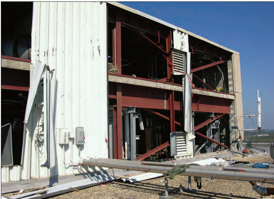
Figure 5-20. The metal wall panels blew off the penthouse on this 15-story building. Rainwater infiltration damaged the elevator controls (estimated wind speed: 130 mph. Gulfport, Mississippi).
