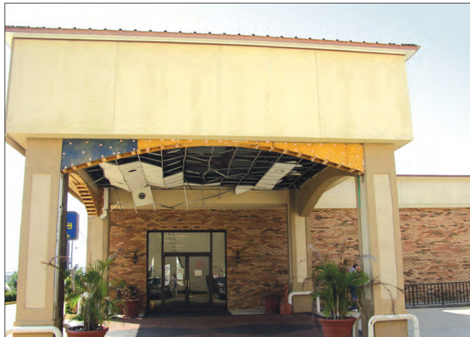
Figure 5-33. Loss of soffit at canopy. The grid support did not have compression struts (estimated wind speed: 130 mph. Gulfport, Mississippi).
