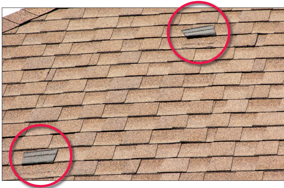
Figure 5-52. Two laminated tabs were lifted (circles) at a house under construction (estimated wind speed: 120 mph. Ocean Springs, Mississippi).
