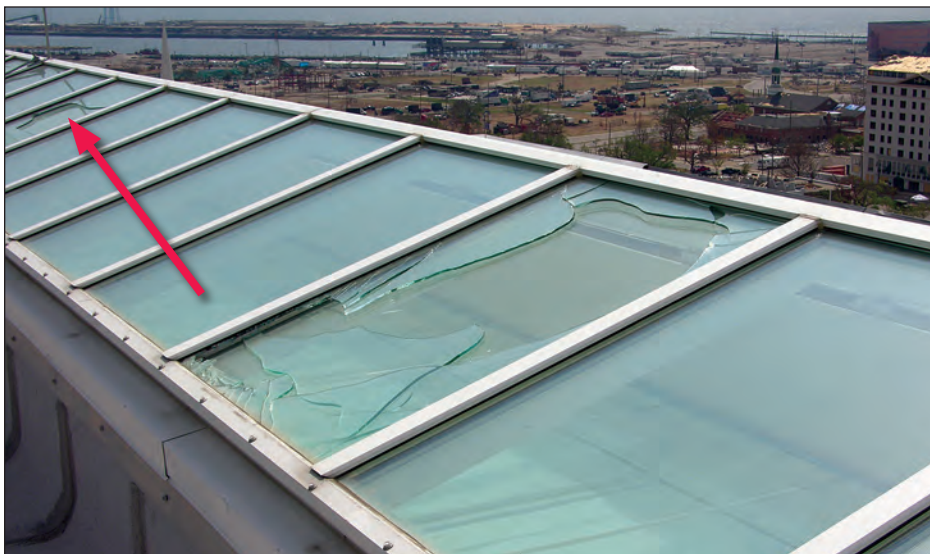
Figure 5-108. Skylight on a new eight-story Federal courthouse. Two of the outer panes were broken. Windborne shards can cause injury and damage buildings and vehicles (estimated wind speed: 130 mph. Gulfport, Mississippi).
