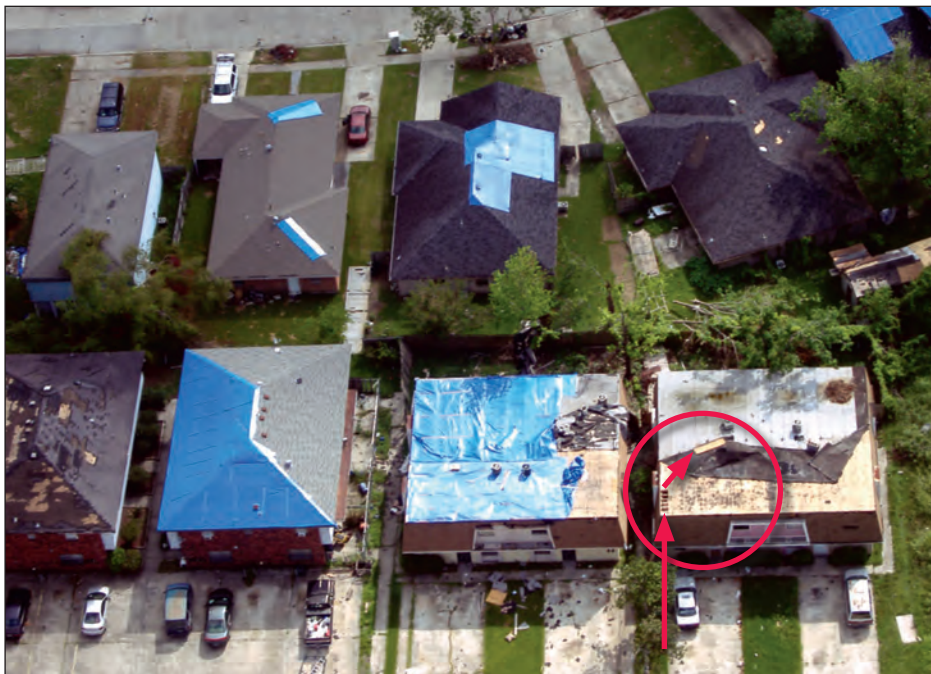
Figure 5-34. Asphalt shingles were damaged on seven of these houses. The two houses on the lower right had built-up or modified bituminous cap sheets. The blow-off at the lower right was likely initiated by blow-off of a deck panel from the corner (estimated wind speed: 105 mph. New Orleans, Louisiana area).
