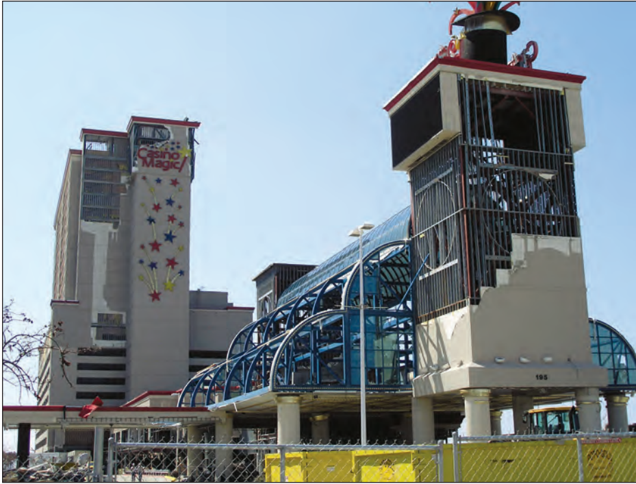
Figure 5-9. Multi-story building in Exposure C, showing severe EIFS damage. The gypsum board typically detached from the studs. In some areas, the gypsum board on the interior side of the studs was also blown away (estimated wind speed: 120 mph. Biloxi, Mississippi).
