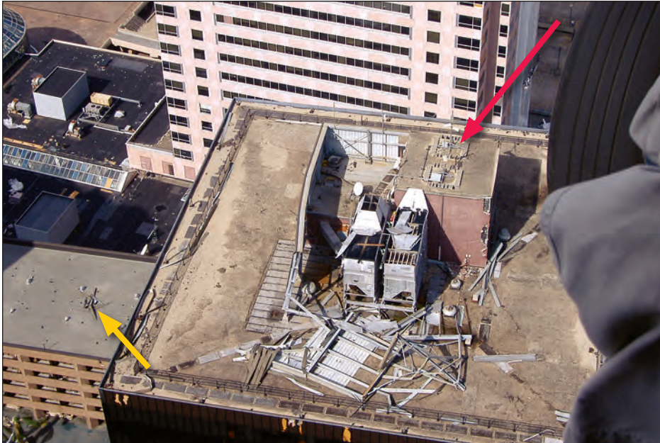
Figure 5-88. View of the roof of S4. Note the glazing damage on the east side of S4 (bottom of figure). Equipment screen wall panels landed on a lower roof (yellow arrow). The penthouse roof (red arrow) did not have a parapet (estimated wind speed: 105 mph. New Orleans, Louisiana).
