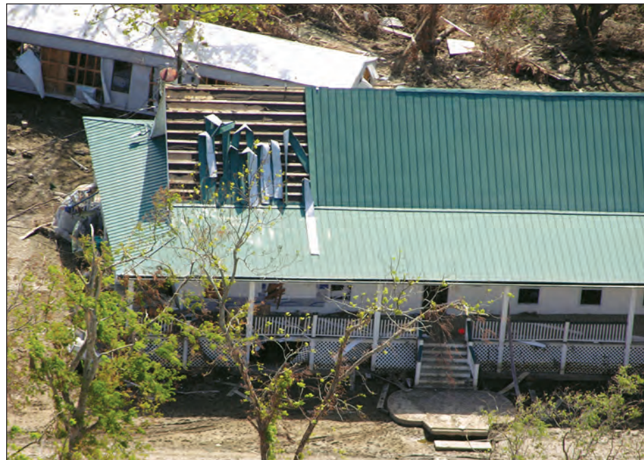
Figure 5-64. Loss of architectural standing seam panels. The panels were installed over 2x4 nailers over underlayment and wood sheathing panels. Much of the exposed underlayment was blown away, thereby allowing rainwater infiltration (estimated wind speed: 130 mph. Buras, Louisiana).
