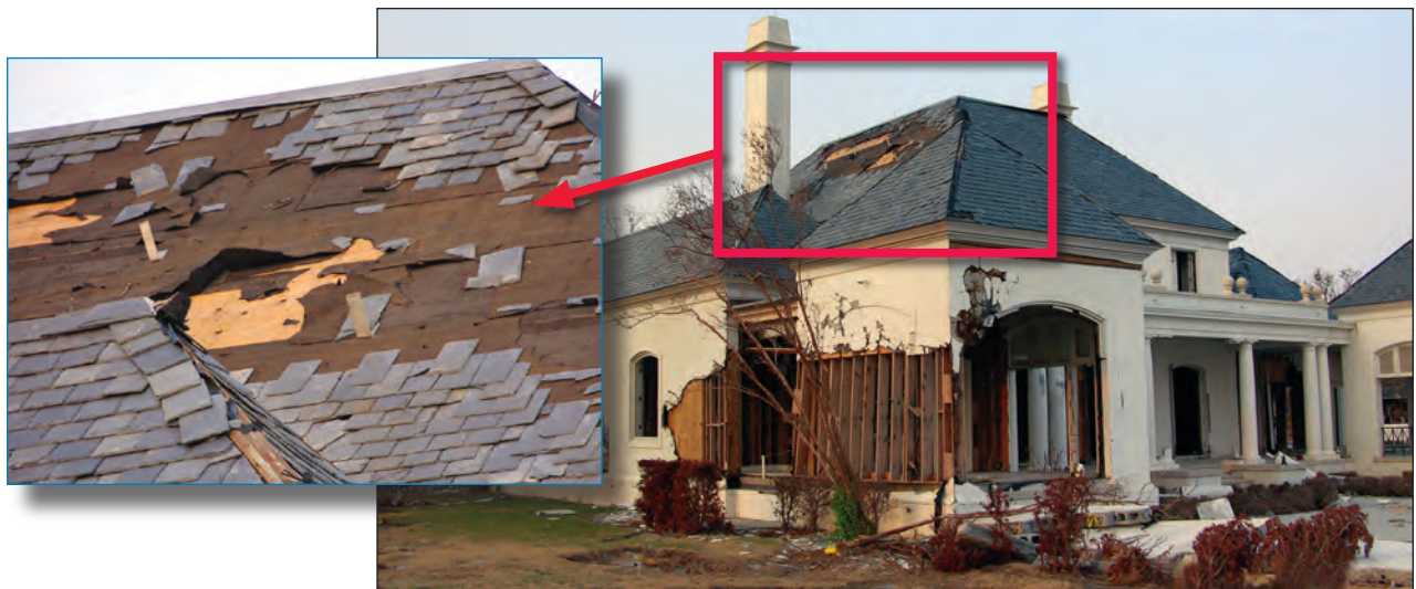
Figure 5-56. Damaged slate roof. The nails typically pulled out of the deck. However, as shown in the square/inset, some of the slates broke and small portions remained nailed to the deck. This house was located in Exposure C (estimated wind speed: 130 mph. Gulfport, Mississippi).
