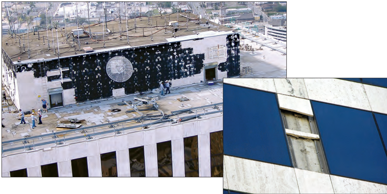
Figure 5-25. Several stone veneer panels blew off the penthouse and caused significant puncturing damage to the modified bitumen membrane roof. A few panels were also blown off the main walls (inset) (estimated wind speed: 105 mph. New Orleans, Louisiana).
