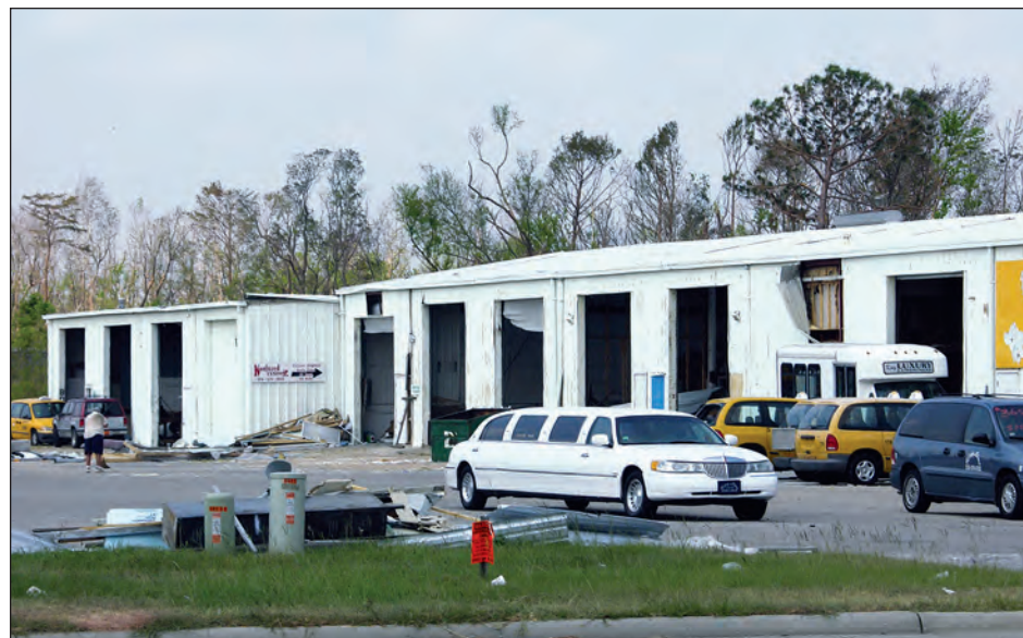
Figure 5-7. Wind-induced damage to several roll-up doors (estimated wind speed: 130 mph. Gulfport, Mississippi)
