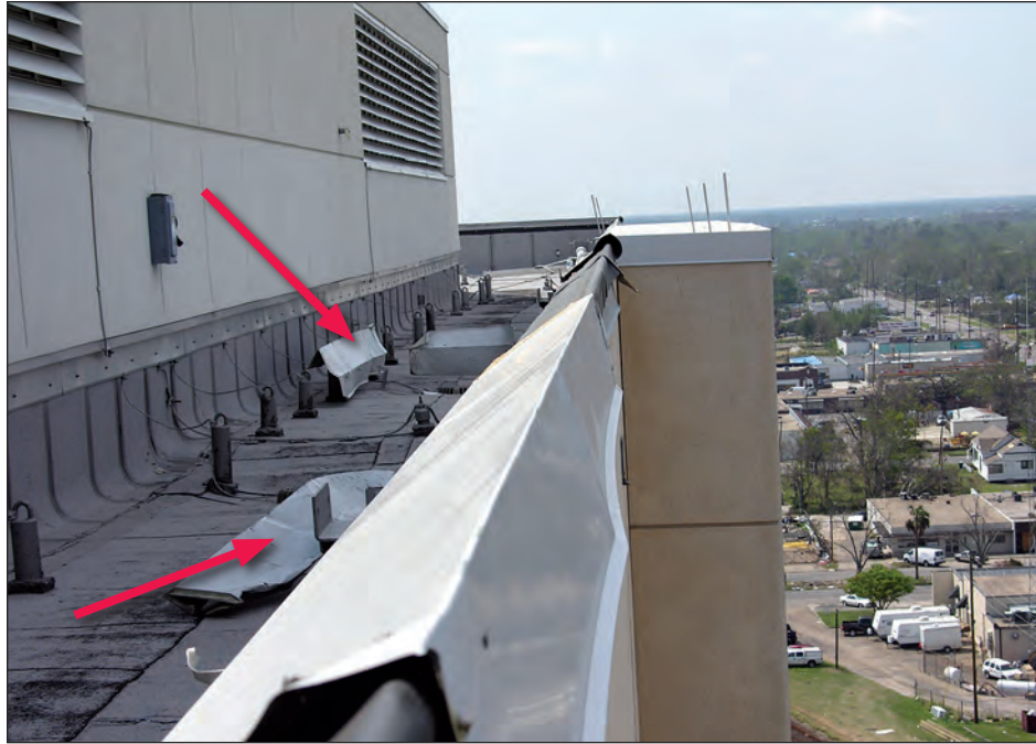
Figure 5-69. This coping unlatched from the cleat because the cleat hem was too short. Two sections of detached coping are resting on the roof (red arrows) (estimated wind speed: 130 mph. Gulfport, Mississippi).
