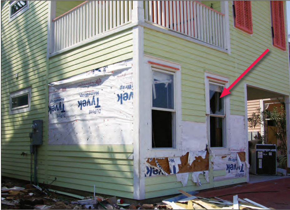
Figure 5-19. Blow-off of fiber-cement siding. Note the broken window at the right (arrow) (estimated wind speed: 125 mph. Bay St. Louis, Mississippi).
