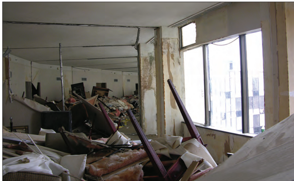
Figure 5-75. Interior view of the hotel shown in Figures 3-47 and 5-82. After the exterior glazing broke, wind knocked down the partitions between the guest rooms and water entered the building (estimated wind speed: 105 mph. New Orleans, Louisiana).
