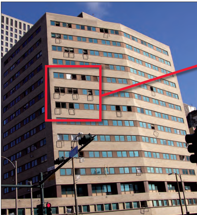
Figure 5-105. Wind pressure caused frame failure at several windows in this building (estimated wind speed: 105 mph. New Orleans, Louisiana).
