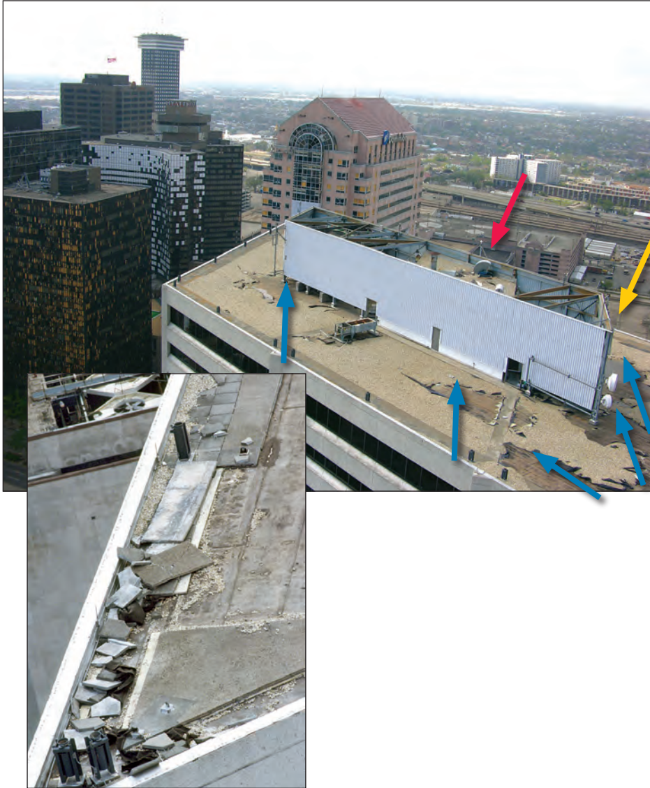
Figure 5-87. Scoured aggregate at Building T1 is shown by the blue arrows. Aggregate was ramped behind the parapet (yellow arrow). A gooseneck lifted from its curb but did not blow away (red arrow). The inset shows displaced pavers and concrete walkway at the windward corner (out of view at the bottom right of the figure) (estimated wind speed: 105 mph. New Orleans, Louisiana).
