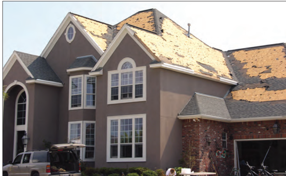
Figure 5-54. Widespread loss of underlayment. With loss of underlayment, water is free to leak into the building and cause extensive interior damage (estimated wind speed: 115 mph. Slidell, Louisiana).
