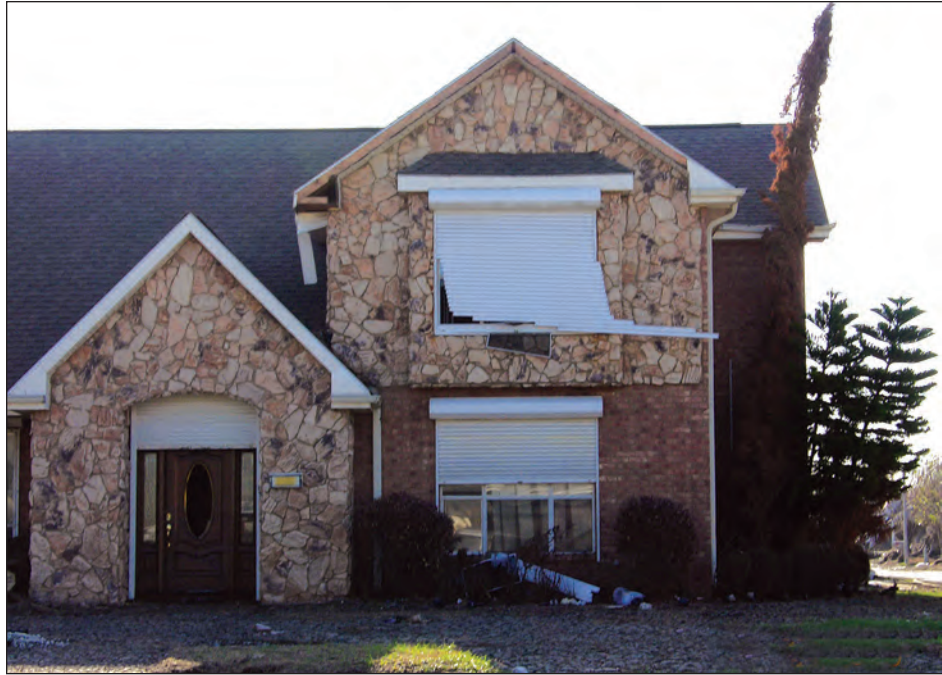
Figure 5-100. This plastic shutter did not completely cover the window. The lower window was broken (estimated wind speed: 105 mph. Pascagoula, Mississippi).
