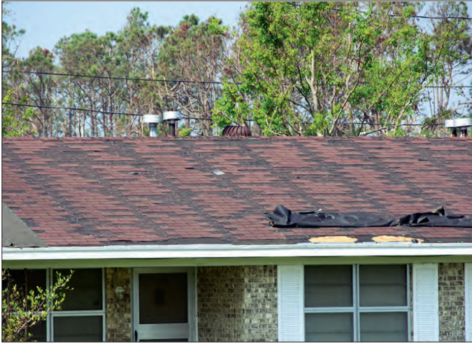
Figure 5-49. The vertical lines of missing tabs are indicative of installation by the raking method. When raked, end nails are frequently not installed. Some shingles and underlayment were also blown from the eave and rake (estimated wind speed: 125 mph. Waveland, Mississippi).
