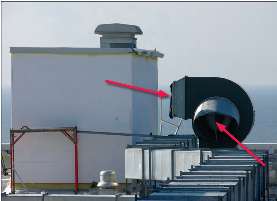
Figure 5-117. Opposite view of Figure 5-116. The ducting on either side of the fan was blown away (red arrows) (estimated wind speed: 120 mph. Biloxi, Mississippi).
