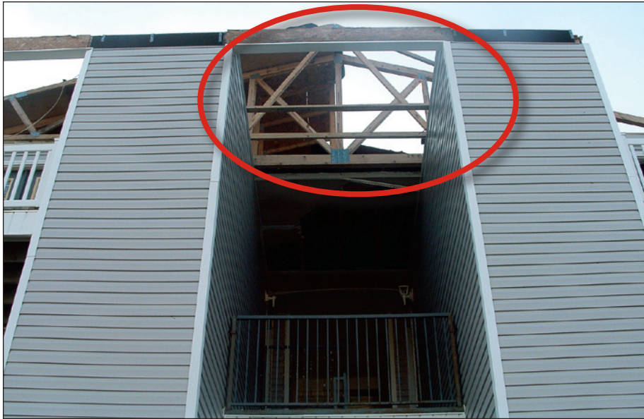
Figure 10-4. Classic soffit failure resulting in attic pressurization and roof decking failure. The stairwell soffit (circled) was blown away during the storm (Long Beach, Mississippi).
