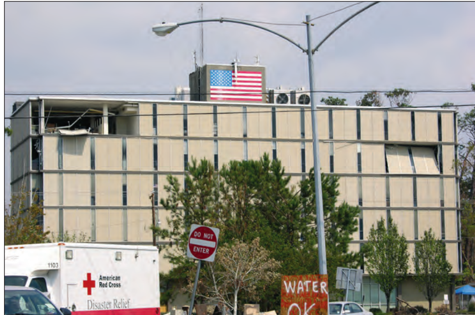
Figure 5-13. Collapse of panelized wall system (estimated wind speed: 115 mph. Slidell, Louisiana)
