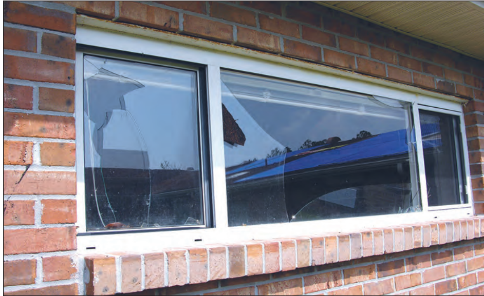
Figure 5-51. Windborne asphalt shingle debris broke several windows in this nursing home. A piece of shingle debris is embedded in the frame (estimated wind speed: 130 mph. Gulfport, Mississippi).
