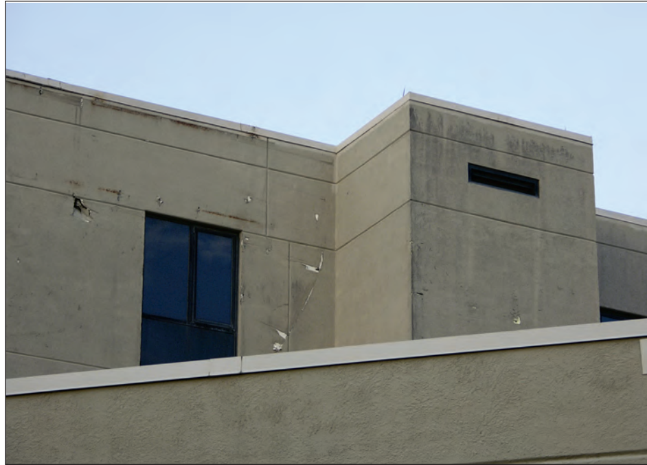
Figure 5-124. A loose LPS conductor whipped the exterior wall and punctured the EIFS in several locations (estimated wind speed: 115 mph. Slidell, Louisiana).
