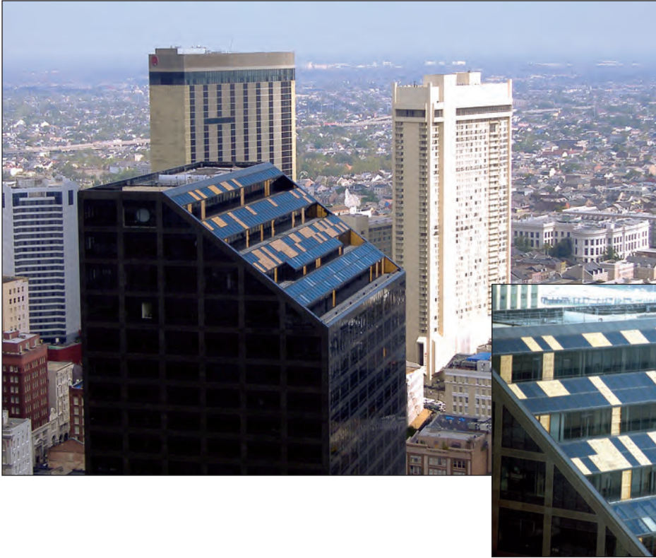
Figure 5-95. Aggregate ballast from the main roof of T7 was the likely source of debris that broke the sloped glazing and nearby windows (estimated wind speed: 105 mph. New Orleans, Louisiana).
