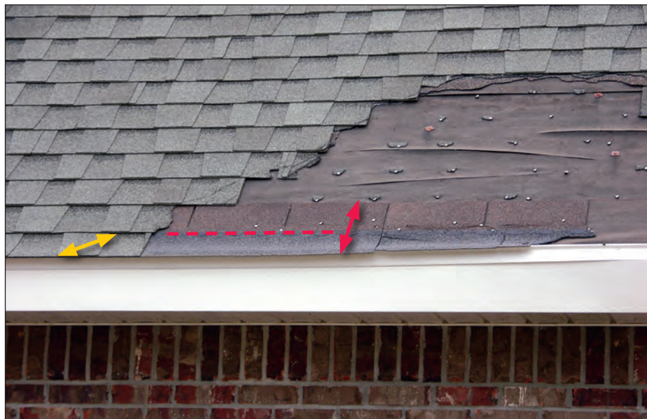
Figure 5-38. Rather than cutting off the tabs of the starter, the starter was rotated 180 degrees (red arrow). The exposed portion of the first course of shingles (yellow arrow) was unbonded because the self-seal adhesive (dashed line) on the starter was not near the eave (estimated wind speed: 130 mph. Long Beach, Mississippi).
