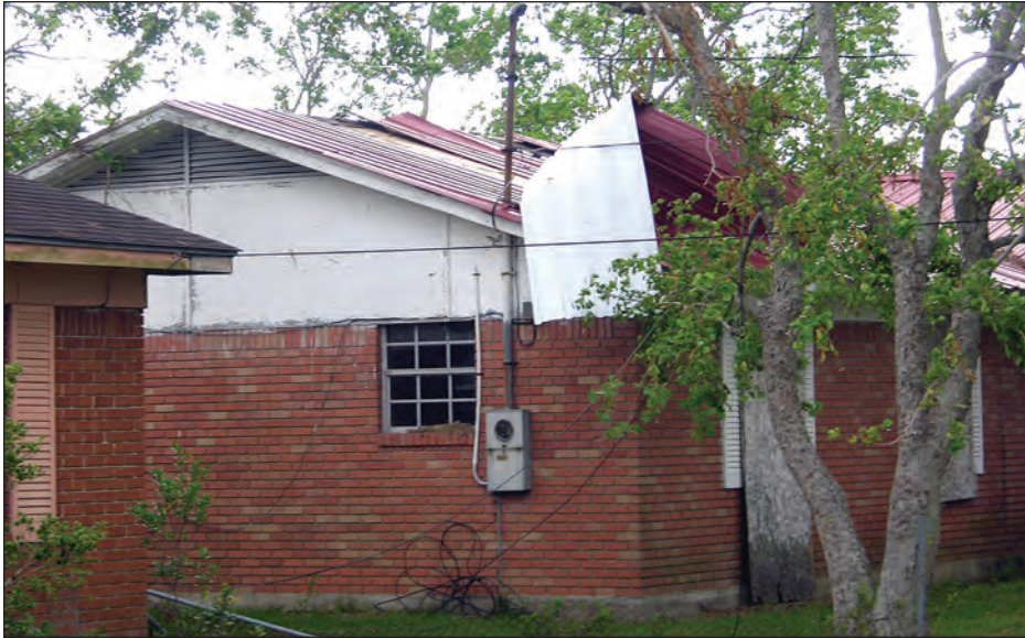
Figure 5-61. Blow-off of decking caused these panels to progressively fail (estimated wind speed: 105 mph. Pascagoula, Mississippi).
