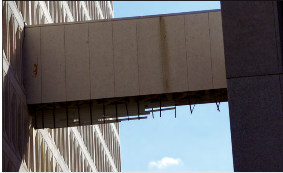
Figure 5-32. Loss of metal soffit from an elevated walkway (estimated wind speed: 105 mph. New Orleans, Louisiana)
