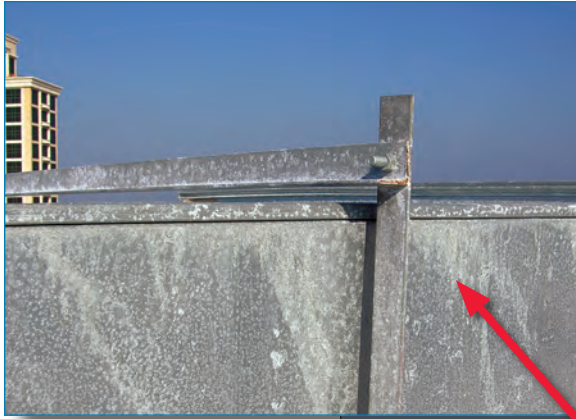
Figure 5-116. These ducts were supported on steel angles (yellow arrow). A steel angle also occurred above the ducts (red rectangle and inset). The building was located in Exposure C (estimated wind speed: 120 mph. Biloxi, Mississippi).
