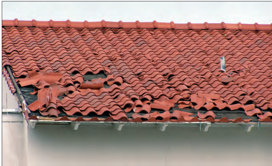
Figure 5-57. Damaged tiles at roof perimeter (estimated wind speed: 120 mph. VA Hospital Chapel, Biloxi, Mississippi)
