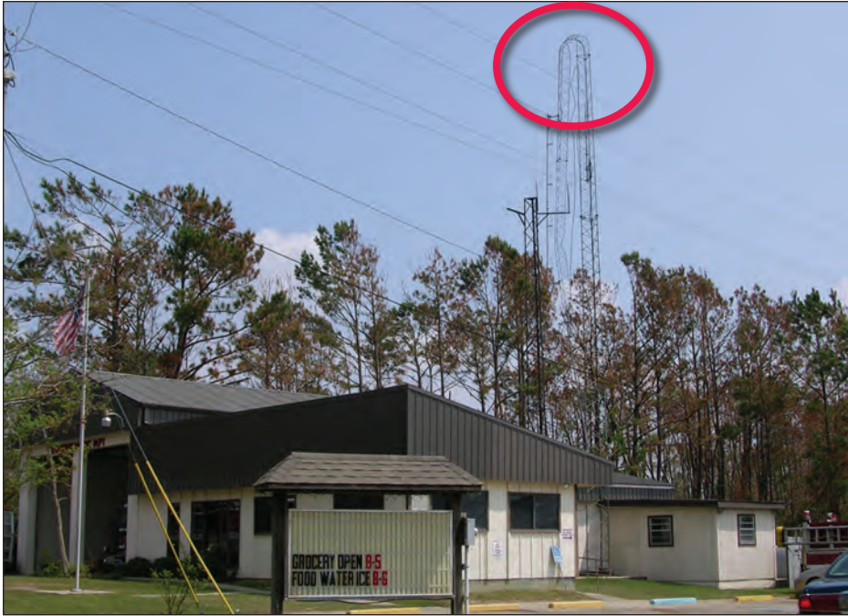
Figure 5-119. The antenna tower at this fire station buckled (estimated wind speed: 120 mph. Diamondhead, Mississippi).
