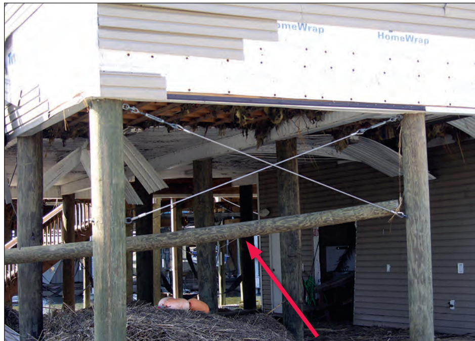
Figure 5-4. Loss of vinyl siding from the underside of an elevated residence in Exposure C. Note the large floodborne pole debris near the steel cable "x" brace (estimated wind speed: 130 mph. St. Bernard Parish, Louisiana).
