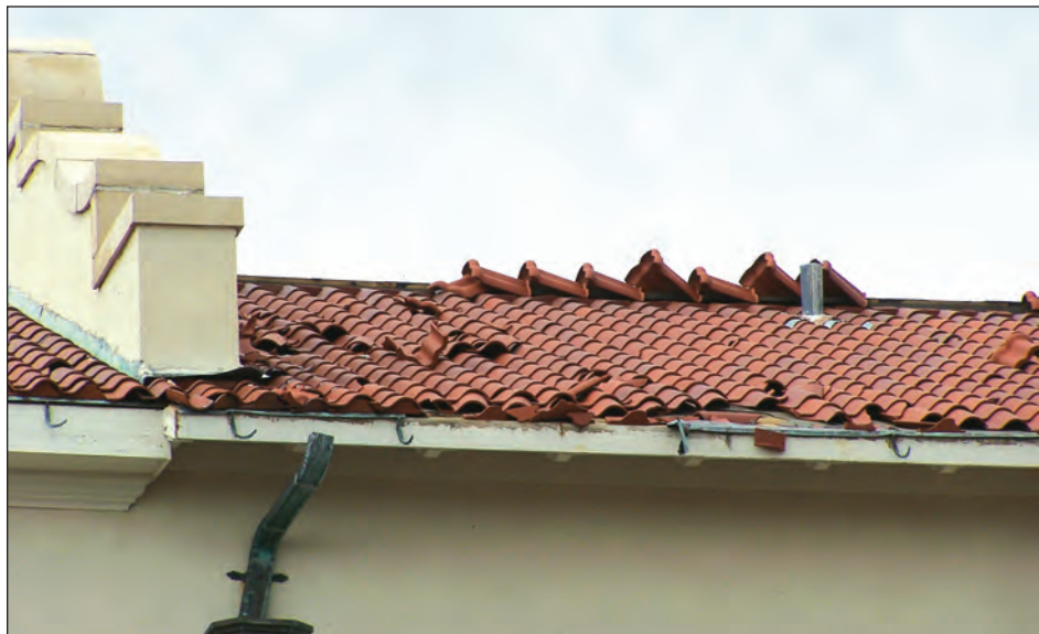
Figure 5-58. Wind turbulence behind parapet resulted in uplift of ridge tiles. Tile was also damaged along the eave (estimated wind speed: 120 mph. VA Hospital Patient Building, Biloxi, Mississippi).
