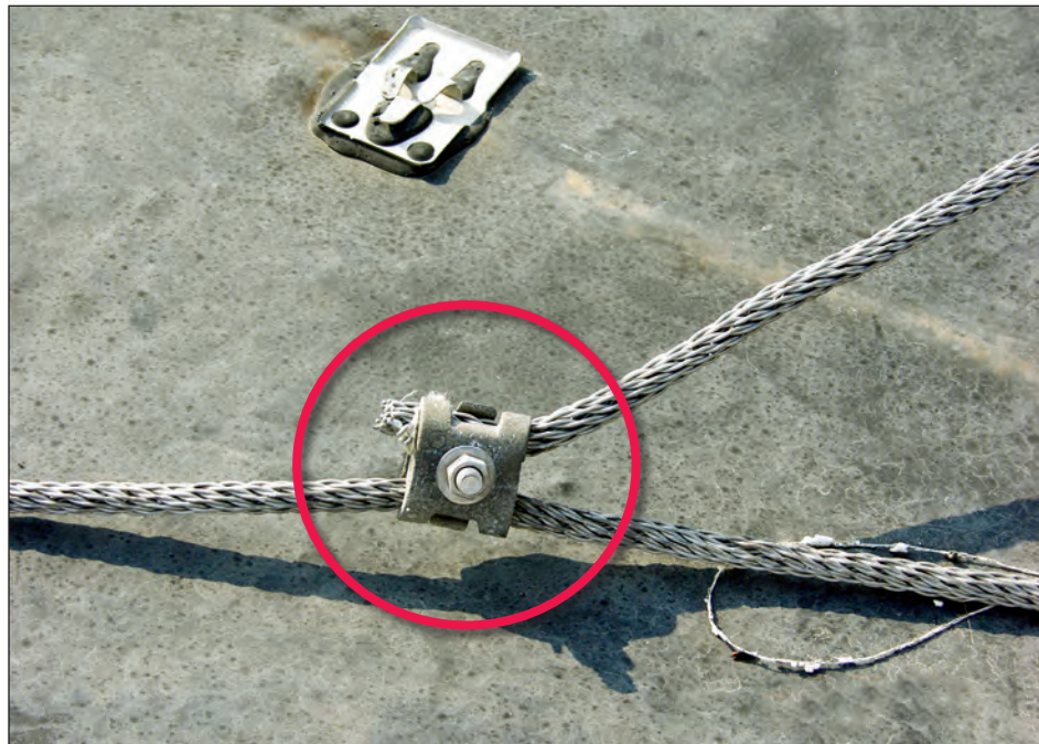
Figure 5-125. A bolted splice connector was used in lieu of a pronged splice connector (estimated wind speed: 130 mph. Gulfport, Mississippi).
