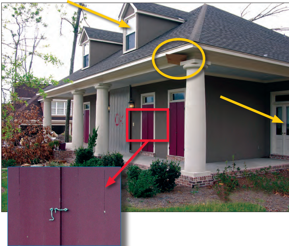
Figure 5-101. Metal shutters were over the main doors, and swinging wood shutters were over the larger first floor windows. However, several windows were unprotected (yellow arrows). The shutter latch (inset) was susceptible to unlatching. Note the wood sheathing debris (yellow circle) (estimated wind speed: 130 mph. Long Beach, Mississippi).
