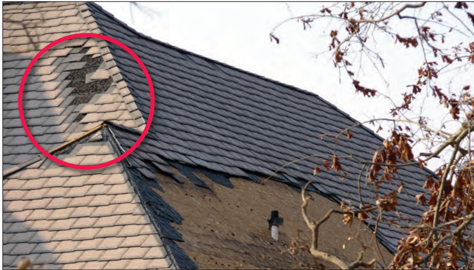
Figure 5-55. Fiber-cement simulating slate. Note the loss of underlayment and the simulated slates broken at the nail line (circle). This house was located in Exposure C (estimated wind speed: 105 mph. Pascagoula, Mississippi).
