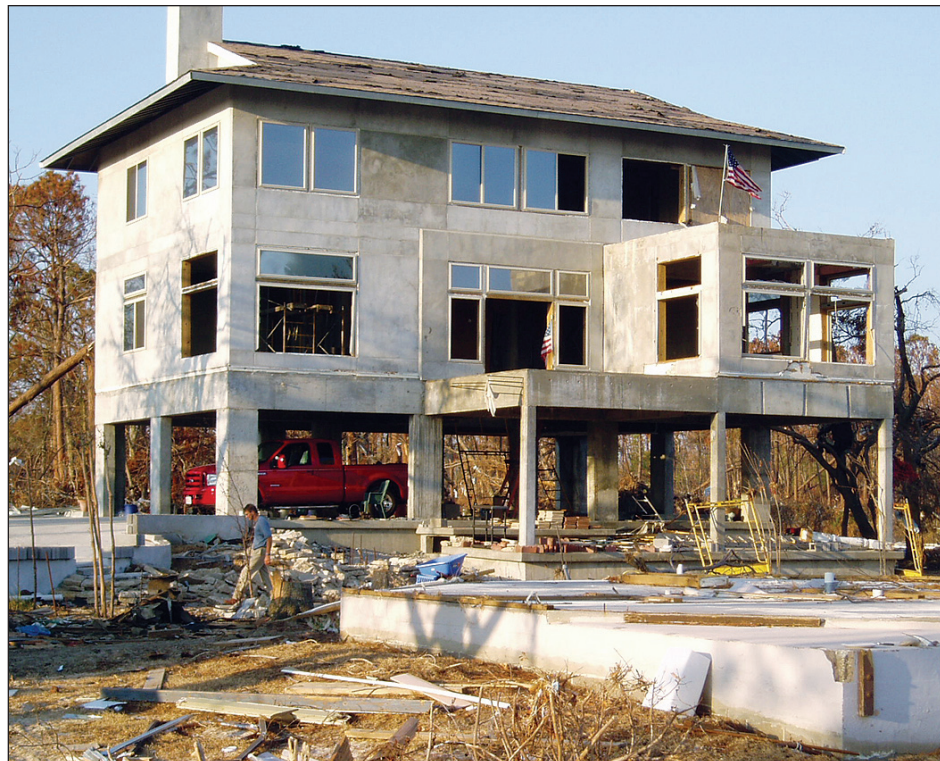
Figure 10-2. Elevation of the lowest floor well above the BFE as indicated by the slab in the foreground (Pass Christian, Mississippi)
