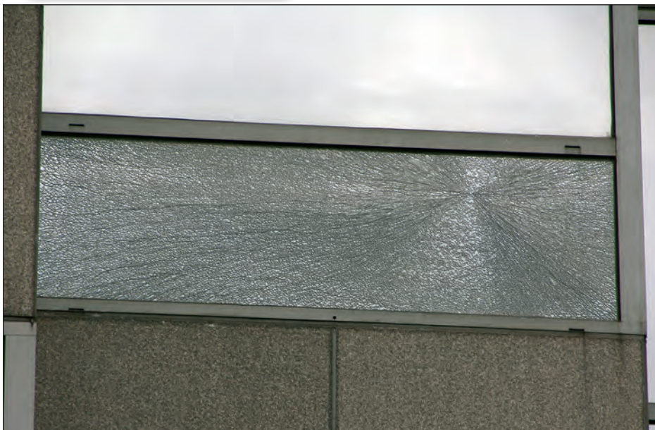
Figure 5-102. The laminated glass broke, but remained in the frame and continued to provide wind and water protection (estimated wind speed: 105 mph. New Orleans, Louisiana).
