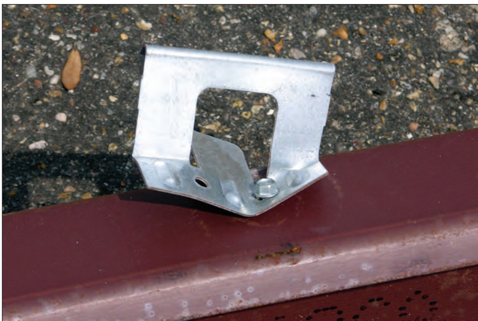
Figure 5-66. The clips for this structural standing seam panel were intended to be attached with two screws. With only one screw, the clips were eccentrically loaded (estimated wind speed: 130 mph. Long Beach, Mississippi).
