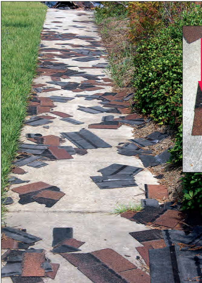
Figure 5-50. Many shingles were blown from a nursing home. Limited checking found three shingles that were missing the right end nail (see inset for one of these). The nails that were installed were placed very high (red arrows); many missed or just nicked the underlying headlap (estimated wind speed: 130 mph. Gulfport, Mississippi).
