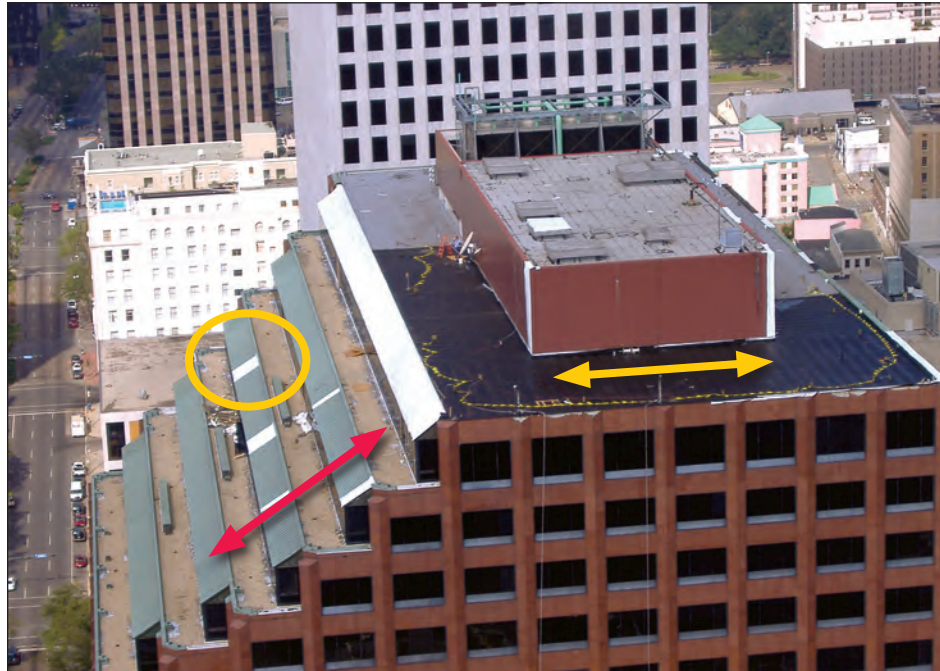
Figure 5-94. The stair-stepped roofs of S6 (red arrow) were aggregate surfaced. Some of the metal roof panels had also blown away (yellow circle). The black area (yellow arrow) is a roof membrane installed after the hurricane (estimated wind speed: 105 mph. New Orleans, Louisiana).
