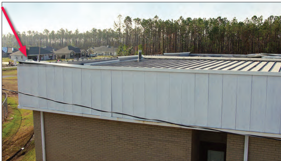
Figure 5-65. The architectural standing seam panels on this school were not continuously seamed. Note the coping damage. This portion of the school was completed in 1988 (estimated wind speed: 125 mph. Waveland, Mississippi).
