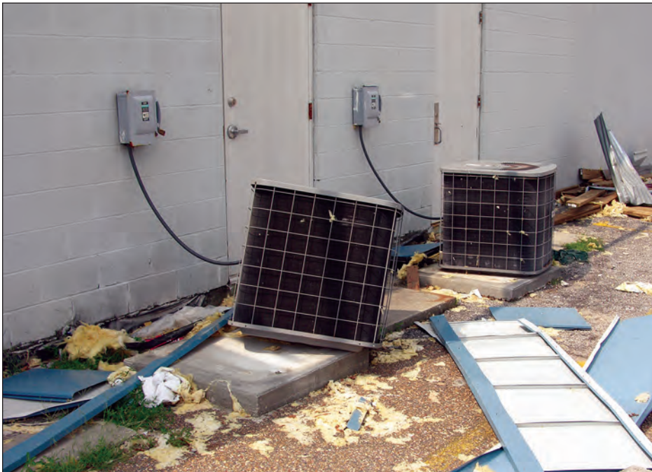
Figure 5-110. Inadequately attached condenser at the police station shown in Figure 3-54 (estimated wind speed: 130 mph. Long Beach, Mississippi).
