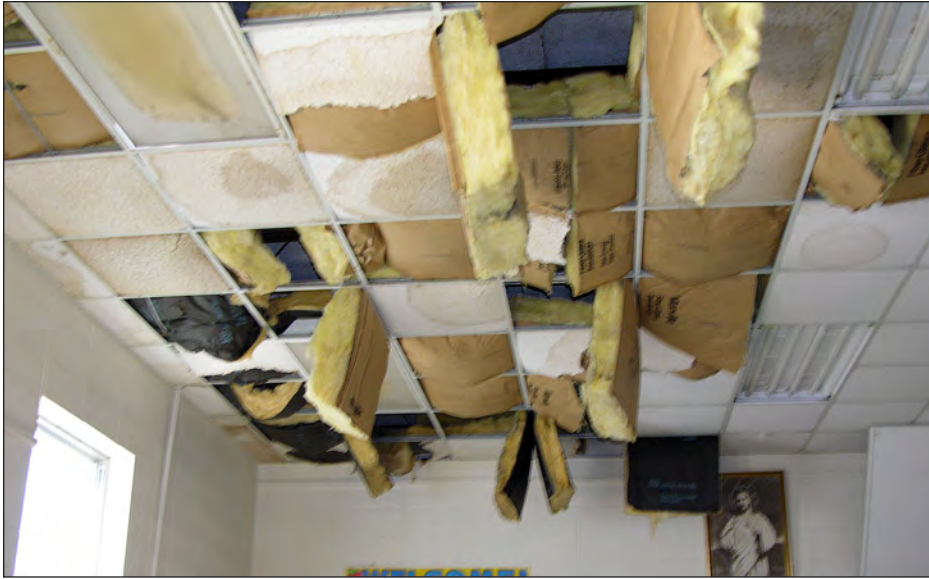
Figure 5-2. After the roof membrane blew off this school, water saturated the fiberglass insulation and ceiling boards, and several of the ceiling boards collapsed (estimated wind speed: 120 mph. Biloxi, Mississippi).
