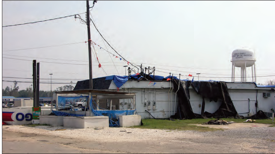
Figure 5-1. Blow-off of a modified bitumen roof membrane at a service station. Note: The cantilevered canopy over the pumps was flipped upside down (estimated wind speed: 85 mph. Mobile, Alabama 1 ).
