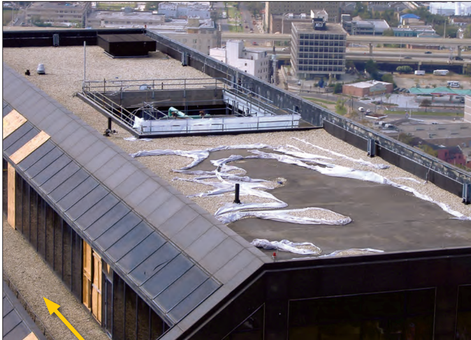
Figure 5-96. Aggregate ballast was scoured and blown from a large portion of the T7 roof. Aggregate also occurred at one, but not all of the stair-stepped roofs (yellow arrow) (estimated wind speed: 105 mph. New Orleans, Louisiana).
