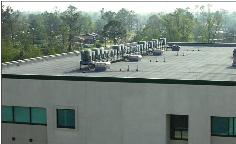
Figure 5-112. The condensers on this new medical office building were anchored to structural steel equipment support stands (estimated wind speed: 130 mph. Gulfport, Mississippi).
