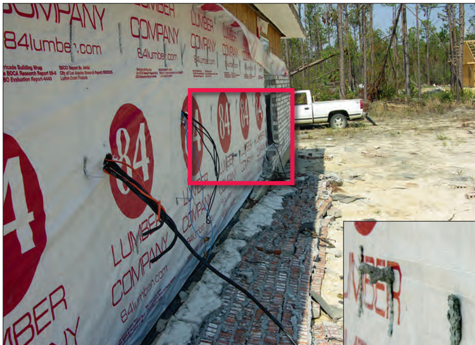
Figure 5-15. Collapsed brick veneer wall that was under construction. Several of the ties had not been embedded into the mortar joints (square/inset) (estimated wind speed: 125 mph. Waveland, Mississippi).
