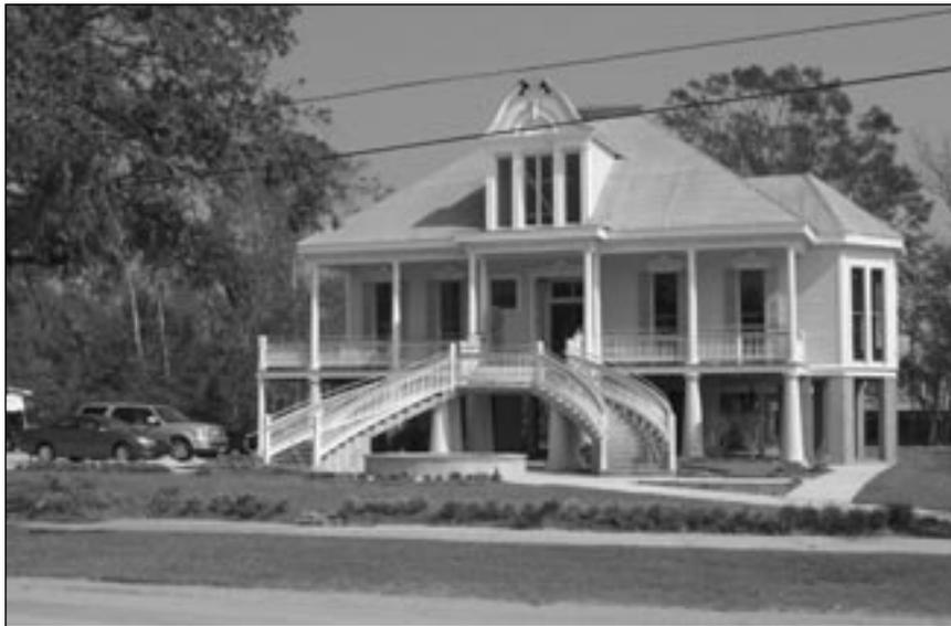
*The Justine Plantation was undamaged by post-Katrina flooding in 2005 because the owners adhered to Mandeville's building codes, requiring that houses sit above the Base Flood Elevation. (Photo by Jeff Markham, FEMA)*
