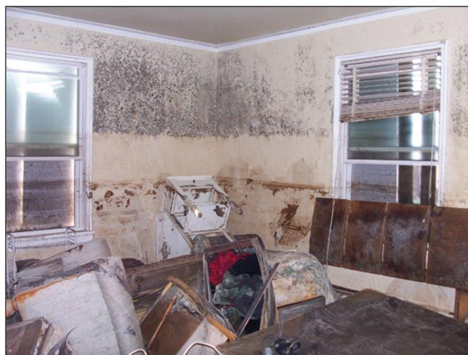
**Figure 1. Typical flood damage to furniture and interior walls (Hurricane Katrina).**
