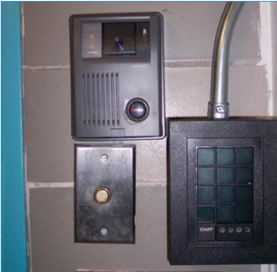
**Figure 5-7:** Electronic entry control device into restricted area.
