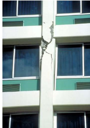
*Damage to older, reinforced concrete building in the 1994 Northridge Earthquake. ©1994 by Peter W. Clark and Regents of the University of California.*
