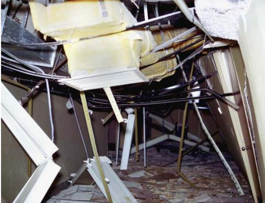
*Non-structural damage to the basement of the Olive View Medical Treatment Building caused by the 1971 San Fernando earthquake. ©1971 by Earthquake Engineering Research Center and Regents of the University of California.*
