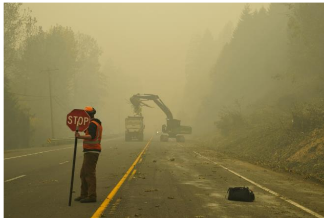
Debris removal during the wildfires. (FEMA, 2020)
