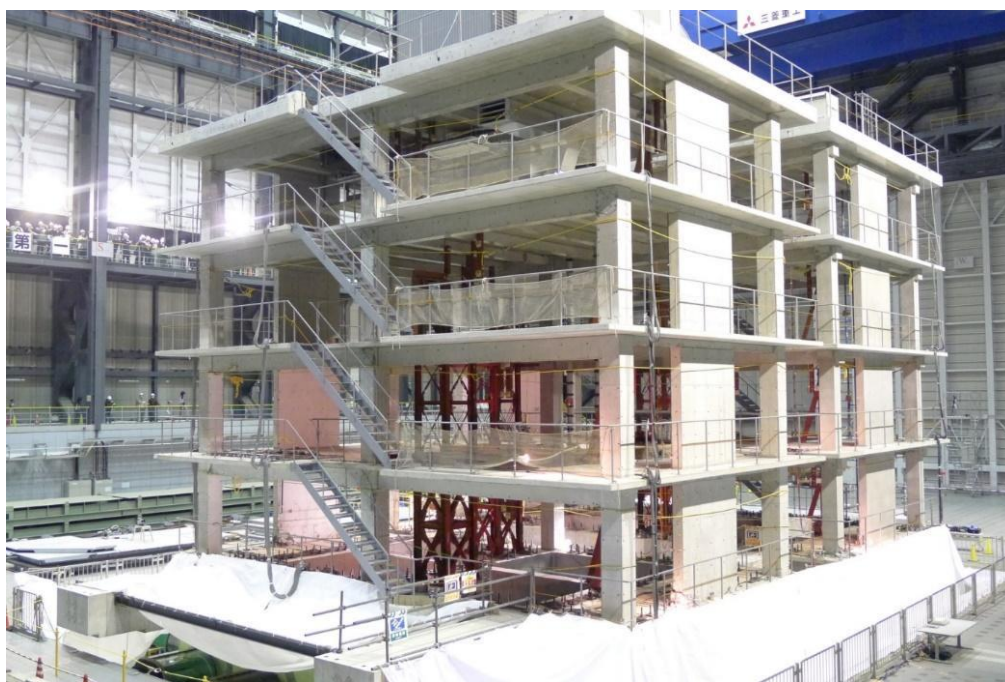
Figure 3-20 RC and PT structures tested at E-Defense shake table (ACI 112-S12).
