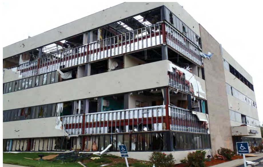
St. John's Regional Medical Center immediately after the 2011 tornado Source: FEMA P-908, Tornado Outbreak of 2011, Materials Assessment Team Report
