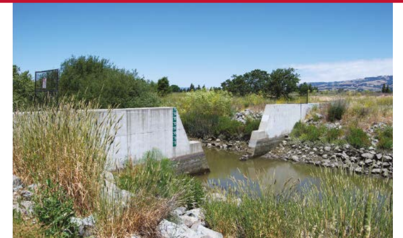
Northern California Flood Control Mitigation
