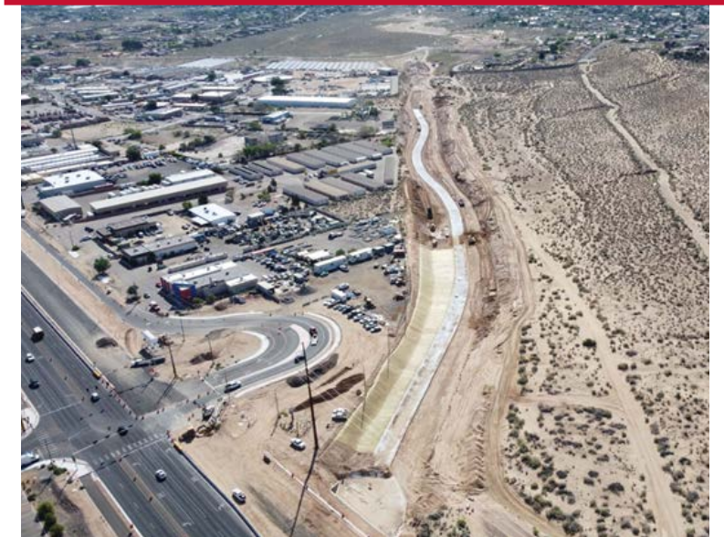
The Rio Rancho Wastewater Plant is adjacent to the arroyo.
