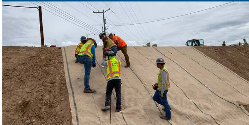
Overview of the Arroyo during installation. Source: Propex Geosolutions
