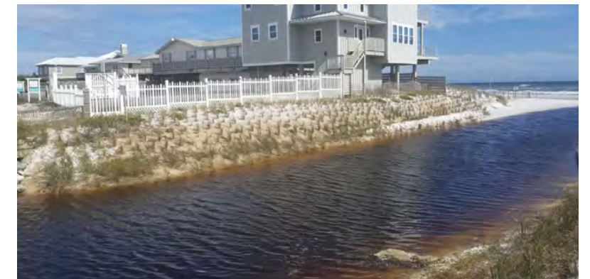
Multiple beach front homes are located at the mouth of the outfall Source: Propex GeoSolutions, https://propexgeosolutions.pixieset.com/oysterlakestabilization/
