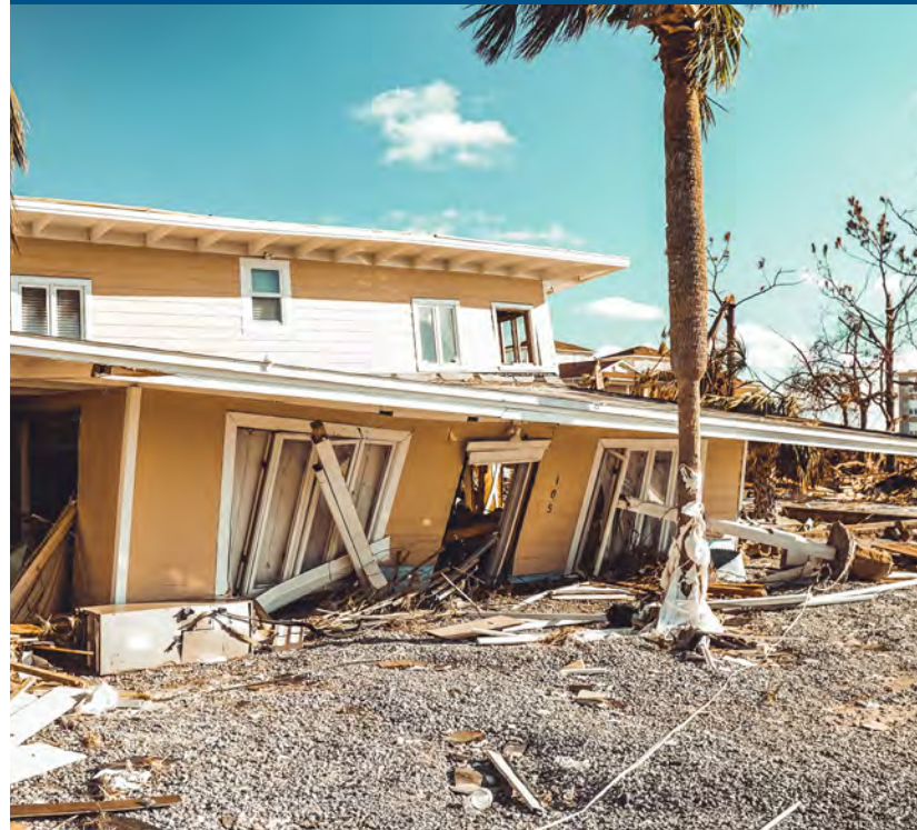
Damage caused by Hurricane Michael in Mexico Beach, FL Source: Shutterstock
