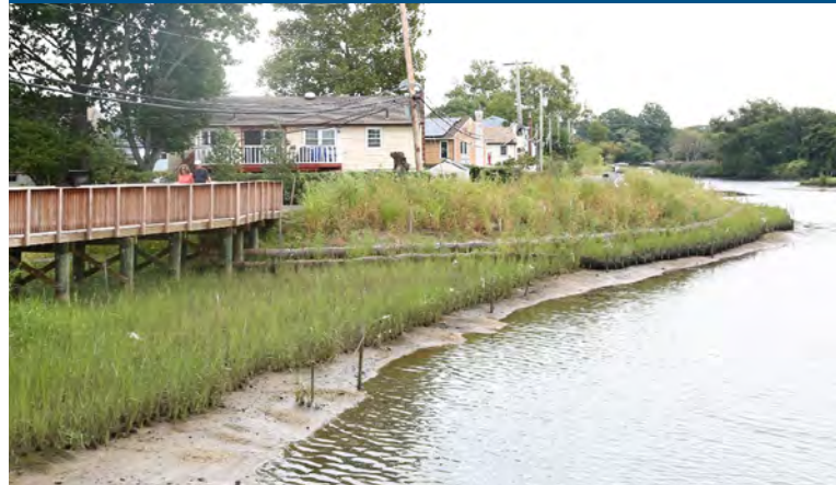
Natural coastal buffer designed to reduce erosion and sedimentation and improve wildlife habitat
