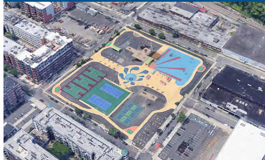
Site of future Northwest Resiliency Park Source: Google Earth Pro, used under license
