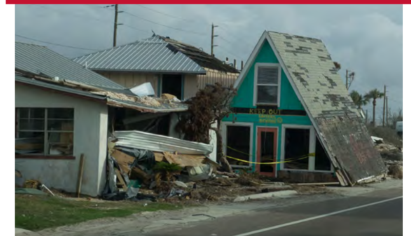
Damage caused by Hurricane Michael in Mexico Beach, FL Source: Shutterstock
