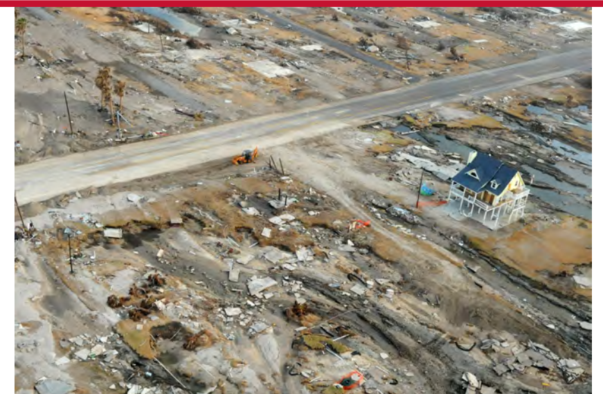
Hurricane destruction surrounding a standing house
