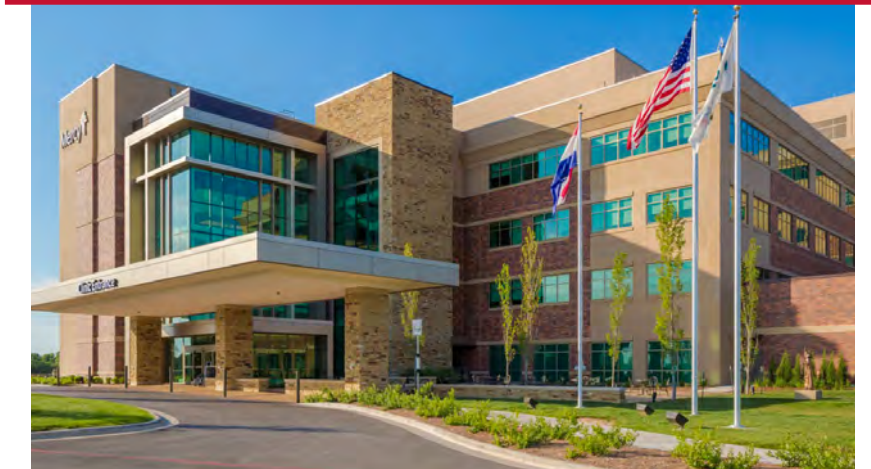
Rebuilt Mercy Hospital as it looks today
