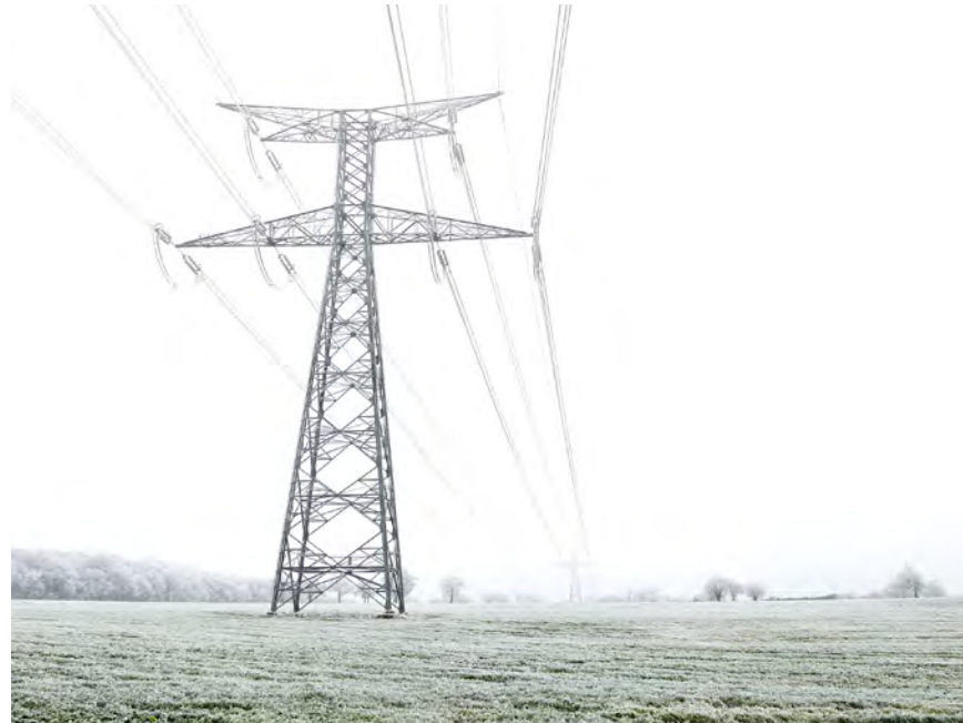
Ice covers electrical sources
