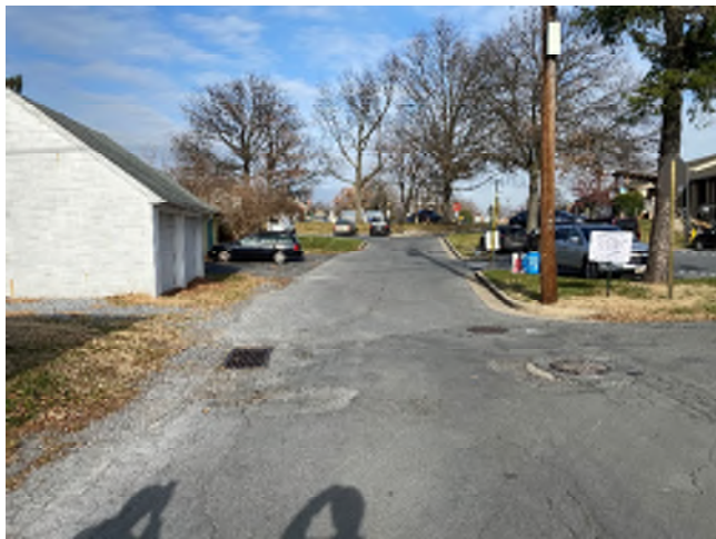
Photo 1: Looking North Along Mews Lane (Project Beginning)
