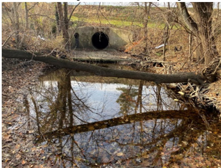
Photo 3: Existing headwall and Plunge Pool
