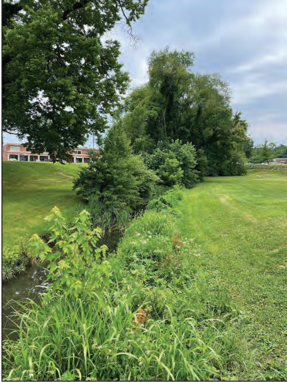
Photo 3: View of the Area of Concern (Phase 2), Abraham Faw Run, facing southwest
