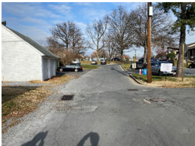
Photo 1: Looking North Along Mews Lane (Project Beginning)
