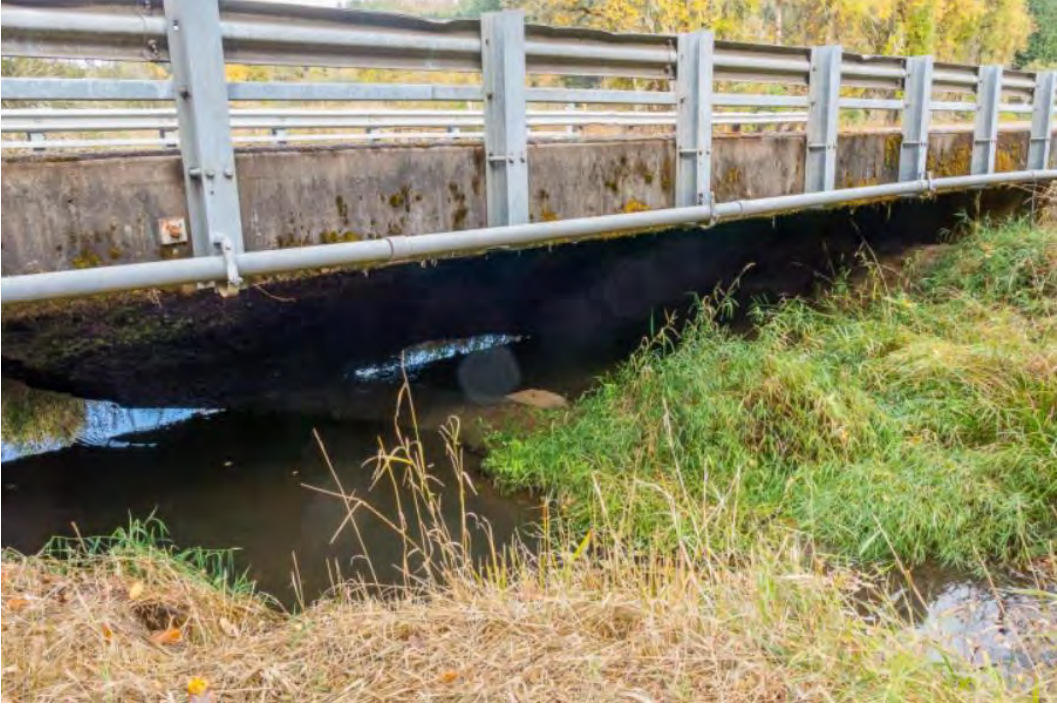
Figure 3: View of existing north bridge (04057A)
