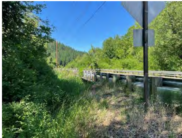
Figure 23: Typical viewshed in the vicinity of the project area
