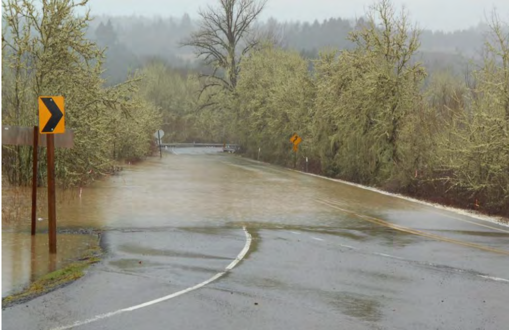
Figure 6: Example of substantial flooding at the intersection of Territorial Highway and Lorane Highway from February 2014
