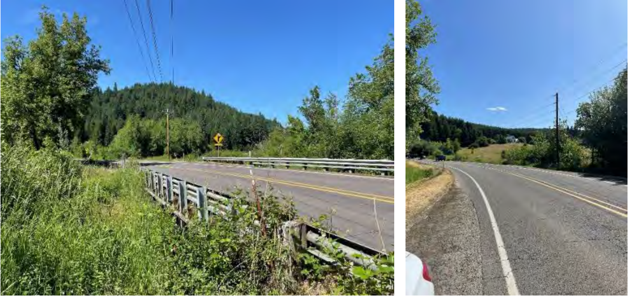
Figure 11 and Figure 12: Overhead utility lines located immediately adjacent to the roadway
