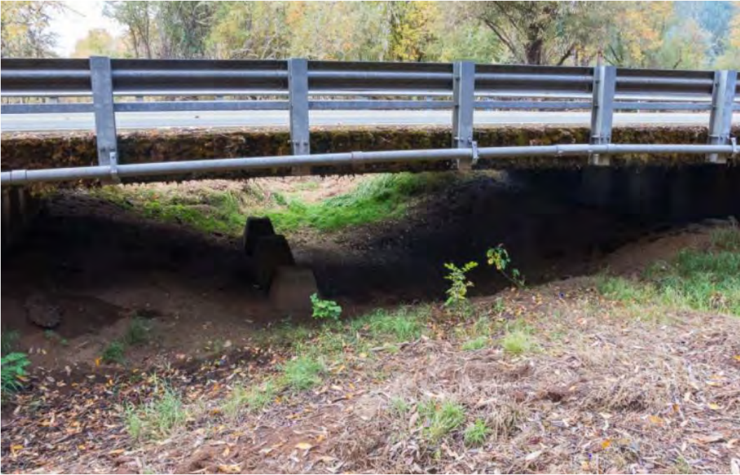
Figure 4: View of existing south bridge (04057B)
