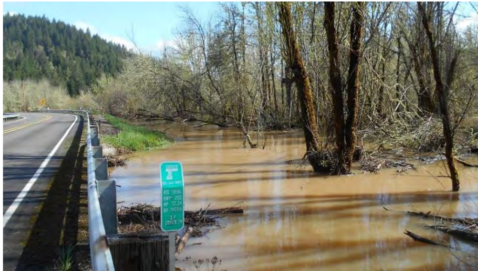
Figure 18: View of the upstream side of south bridge during a flood event
