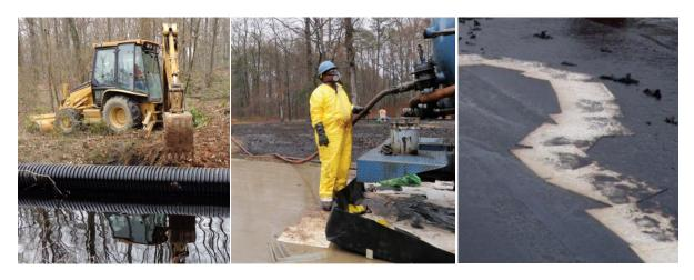
Figure 50: Damming, vacuuming, and sorption for contamination control following a surface spill
