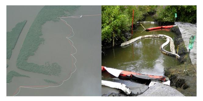
Figure 52: Containment booms on large and small bodies of water
