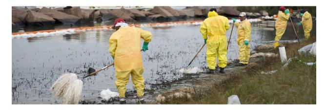
Figure 1: PPE-clad responders cleaning an oil spill with pom-poms and rakes
