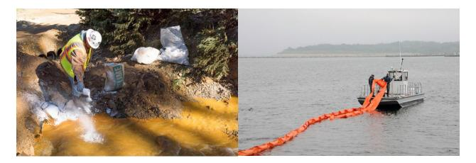
Figure 49: Containment control mechanisms: neutralizing mining wastewater (left) and moving an oil containment boom (right)
