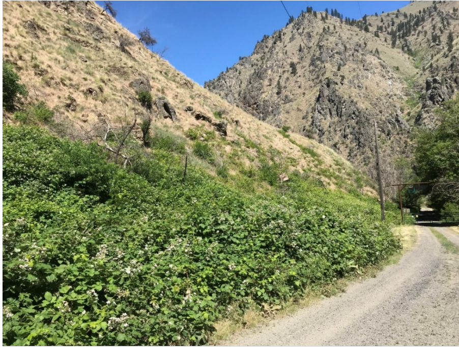
Figure 3-1. Representative Access Road in Project Area
