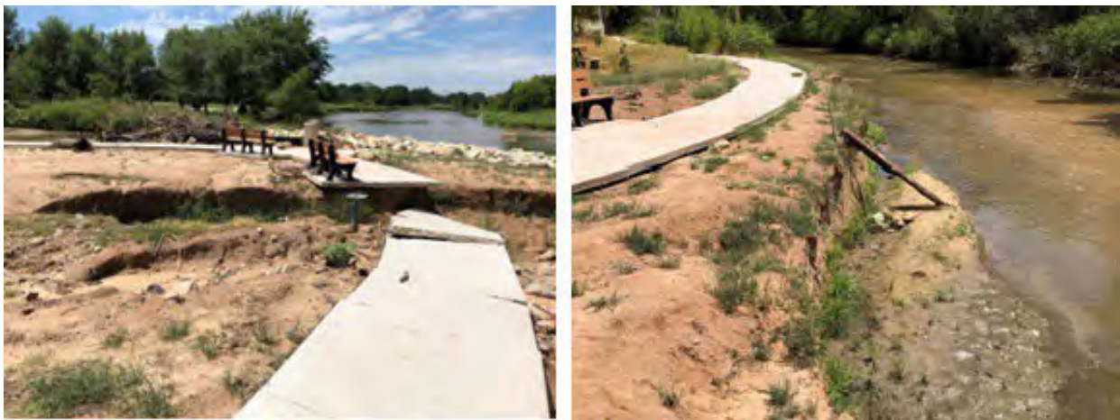
Figure 5: Examples of Damage from 2019 Flood Event
