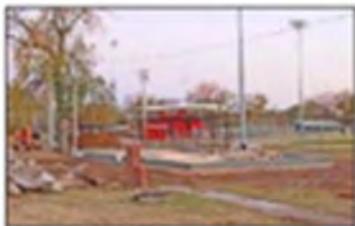
New Restroom/Concessions under construction
