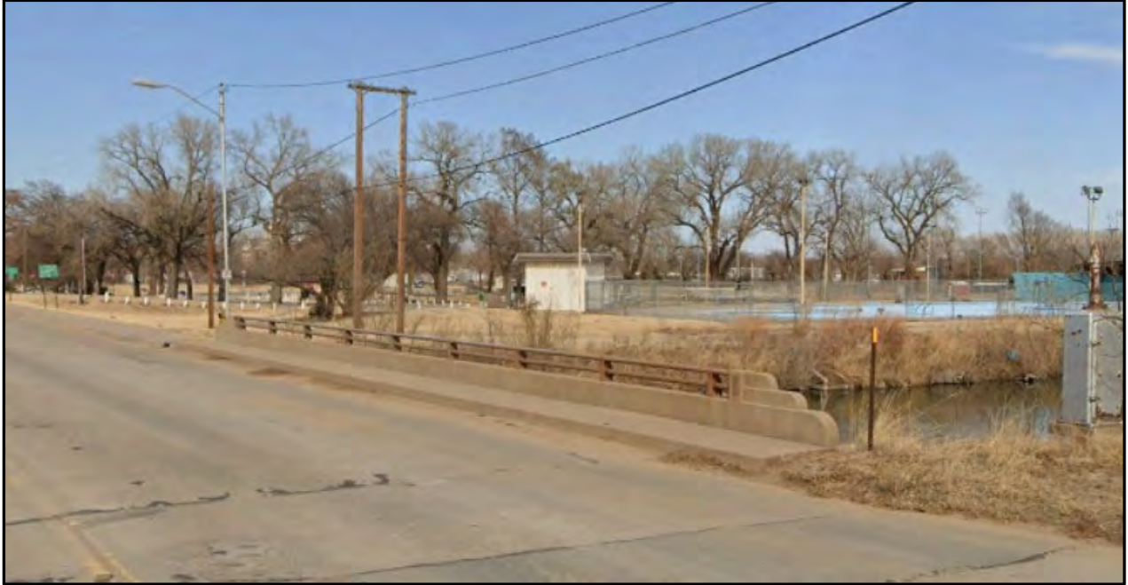
Main Street crossing Ninnescah overflow (Mill Race) view to northeast Source: Google Earth street view (Imagery date – February 2022)
