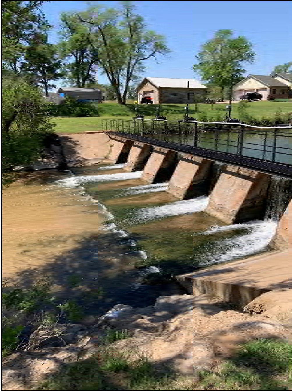
Mill Race Dam (ca.1933) view to southwest Image date: 9 May 2022 FEMA EHP staff photograph
