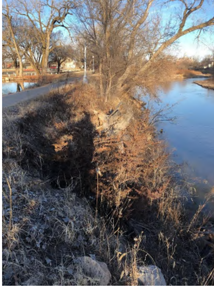
Figure 10: 2021 Ground Level Photos at Eastern End of Eastern Bank Conditions
