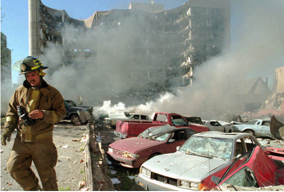
A firefighter surveys the Murrah Building following the Oklahoma City bombing in Oklahoma City, OK on April 19, 1995.
